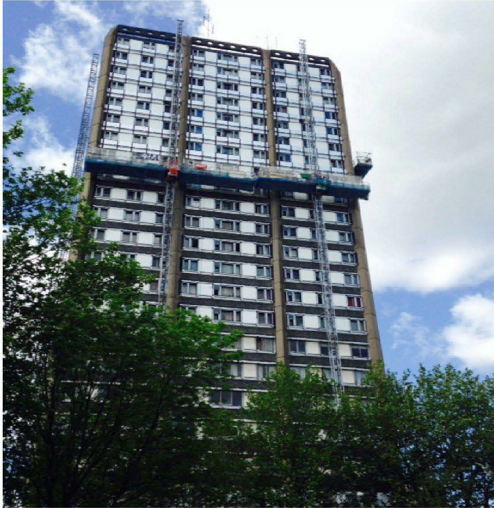
Windows and insulation being installed on the East elevation
