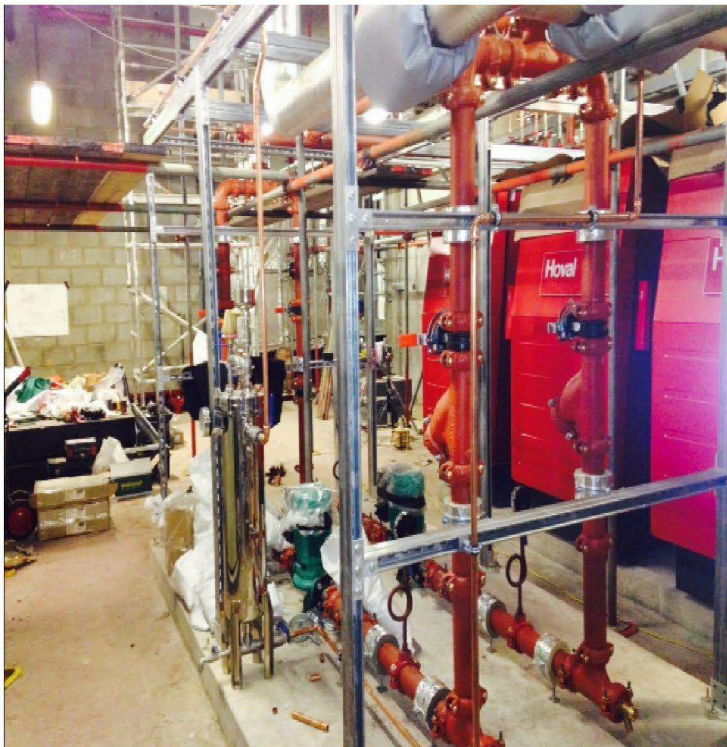
Boiler room works well underway
