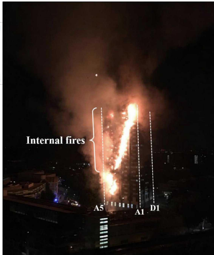
Figure 10.43: Diagonal flame front along External Flame Spread Route 1, that is, on the North elevation of the building envelope at 02:34 on 14 June 2017 (MET00012593) (SEA00010474)
