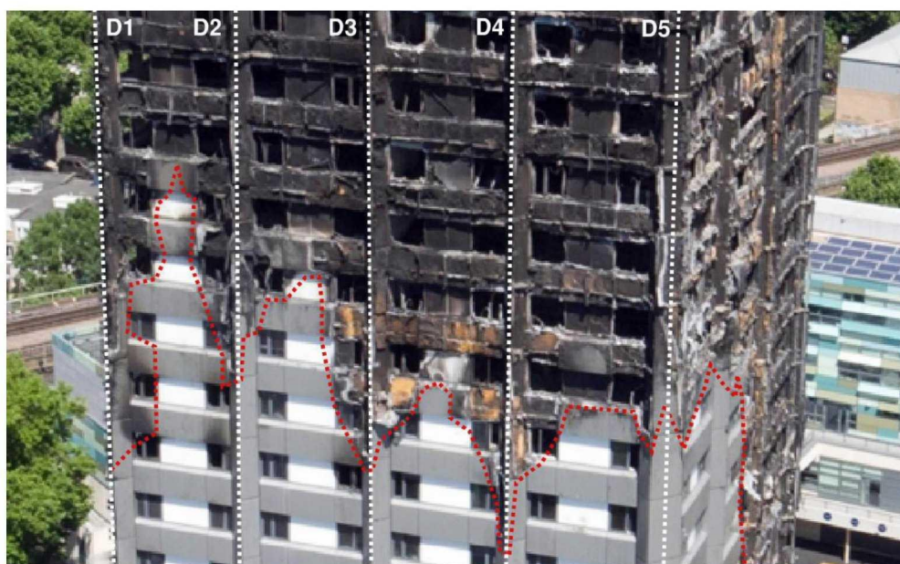
Figure 10.70: Post-fire damage on South elevation of Grenfell Tower (METS00020582)
