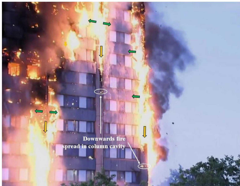
Figure 10.67: Downwards flame spread along columns on the West elevation. 18
