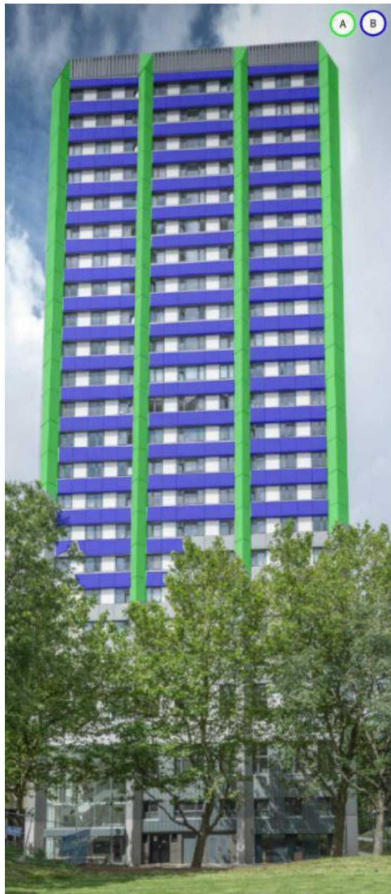
Figure 10.61 Pathways for external fire spread: pathway A and B (SEA00000387)
