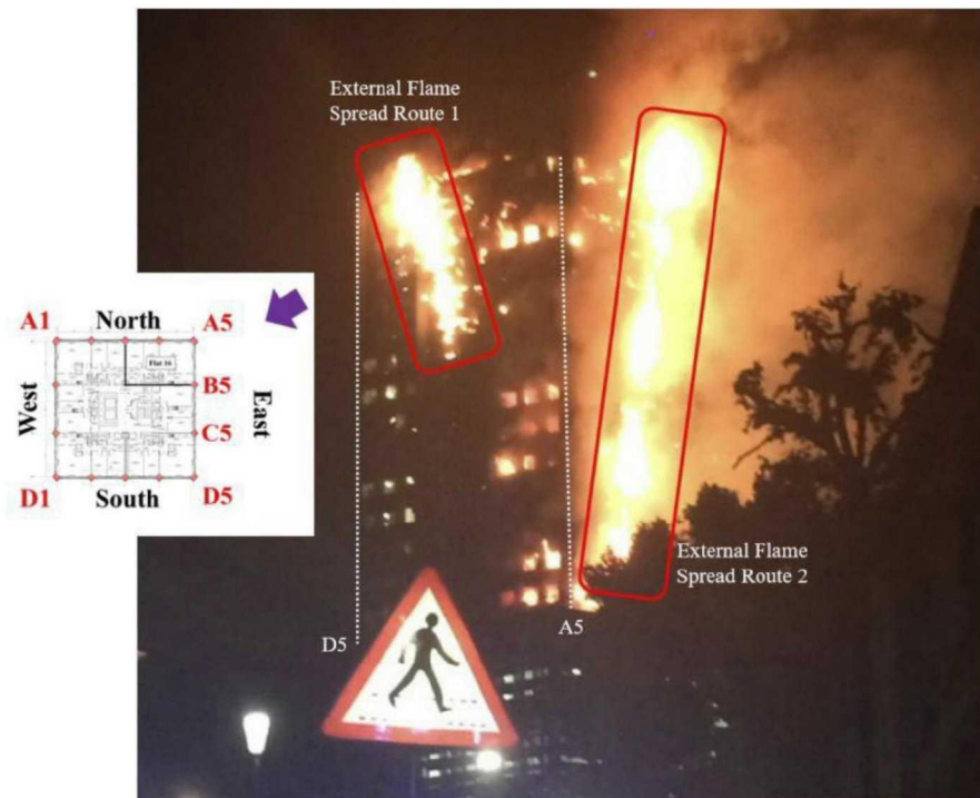
Figure 10.41: Diagonal pattern for External Flame Spread Routes 1 and 2 at 02:08 on 14 th June 2017 (MET00012593) (SEA00010474)
