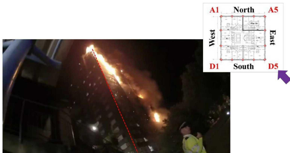
Figure 10.42: Diagonal flame front along External Flame Spread Route 2, that is, around column D5 (southeast corner of building), from East elevation to South elevation of the building envelope at 02:33 on 14 June 2017 (MET00012593) (SEA00010474)
