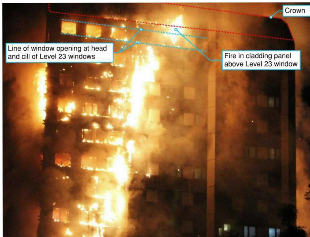
Figure 10.74: Fire in cladding panel above 19
