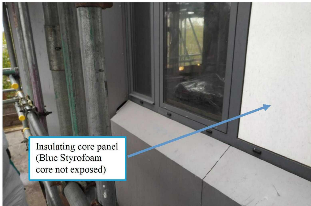
Figure 11.9 Insulating core panel between windows
