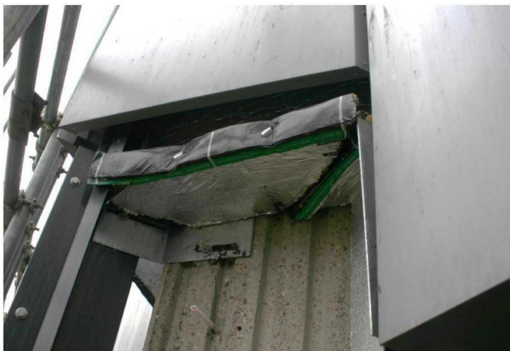
(a) Horizontal cavity barrier affixed to column – upside down position indicated by green logo facing down
