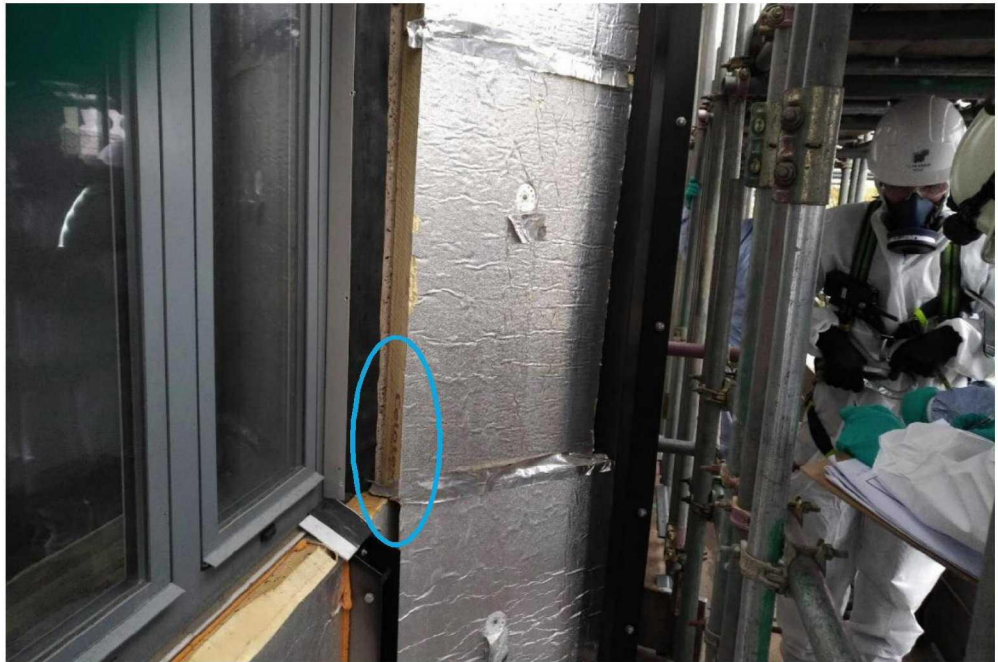
Figure 11.13: Evidence of Celotex in place on the columns of Grenfell Tower note Celotex logo printed on insulation (circled in blue)
