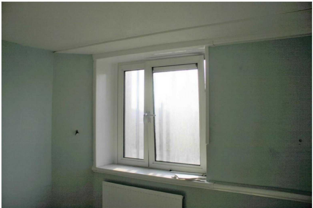
Figure 11.26 Undamaged UPVC surround of window
