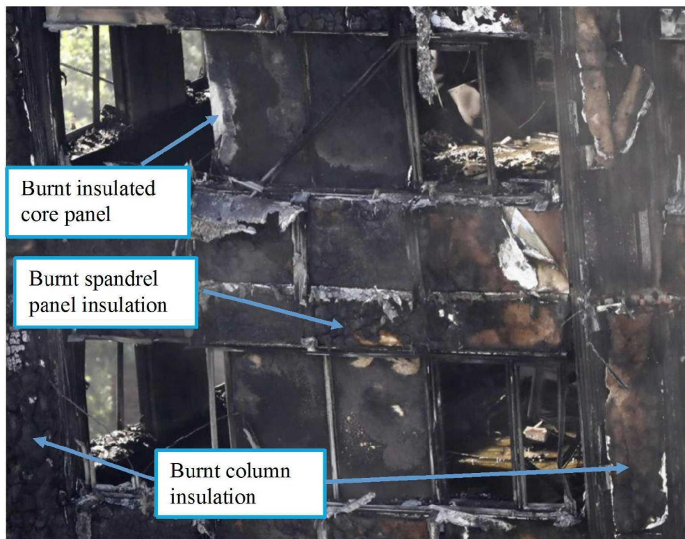
Figure 11.36 External view of burned surfaces
