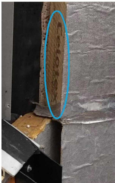
Figure 11.14: Evidence of Celotex in place on the columns of Grenfell Tower (expanded image of Figure 11.13)
