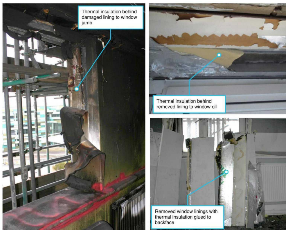
Figure 11.11 Thermal insulation behind the window opening linings
