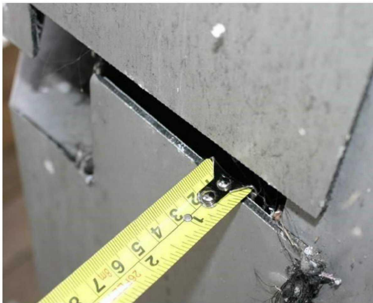
Figure 11.6 Black core observed onsite (photograph from flat 10 on level 3)
