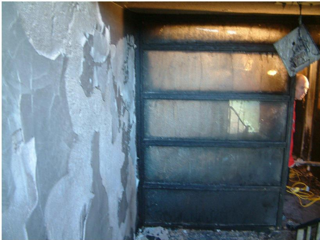
Georgian wired glass partition separating lobby from stairwell on 14 th floor
