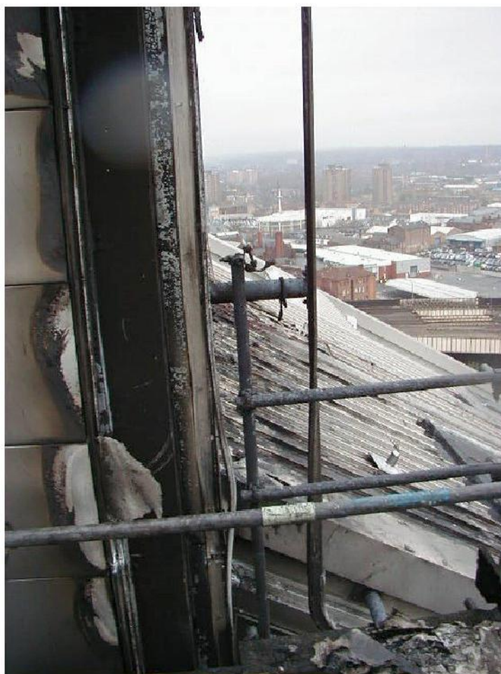
Roof where fire had spread horizontally and downwards due to wind
