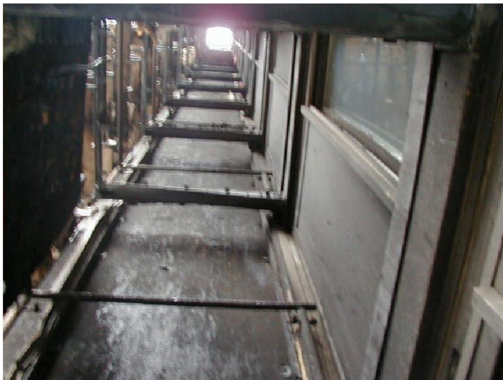
Walls where sandwich panels have been burnt away
