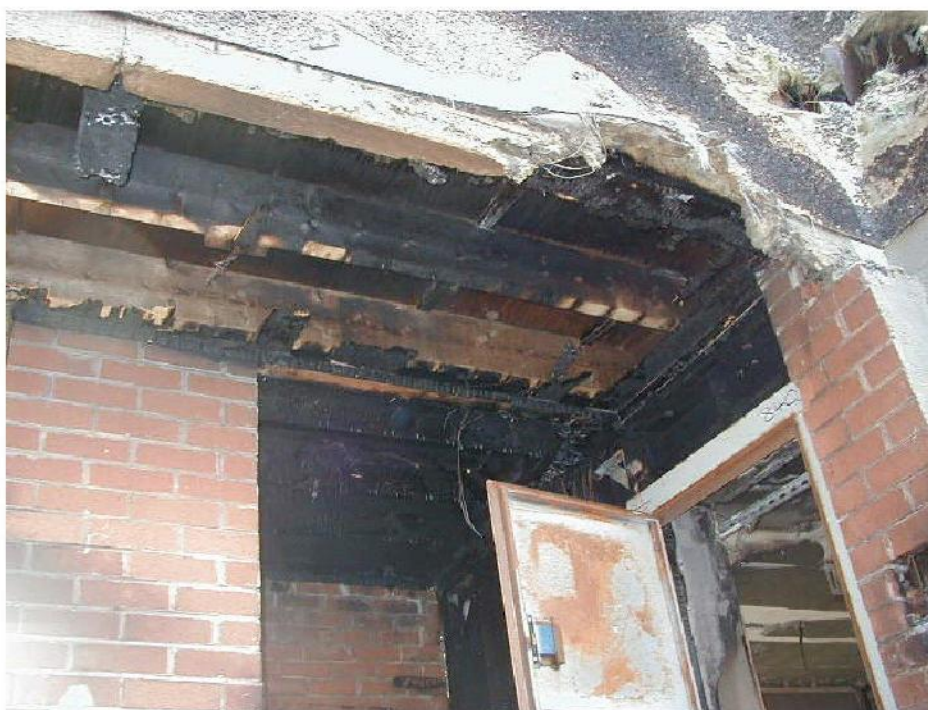
Walkway outside bin store and final exit with wood panelling burnt away
