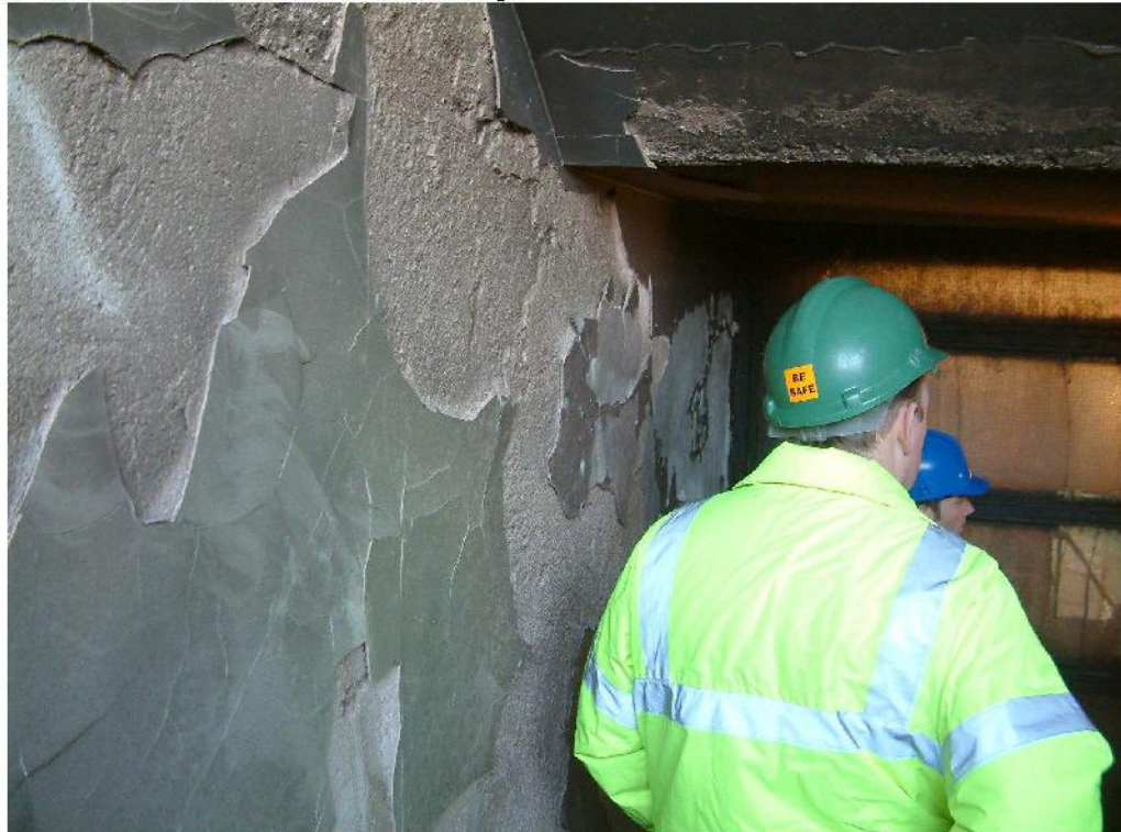
Smoke damage to 14 th floor stairwell
