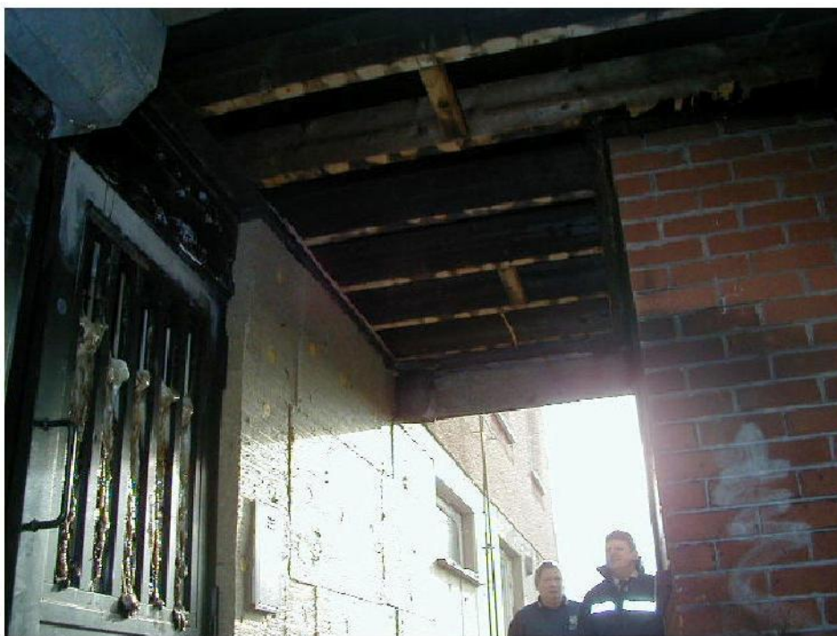
Melted vision panels in final exit door
