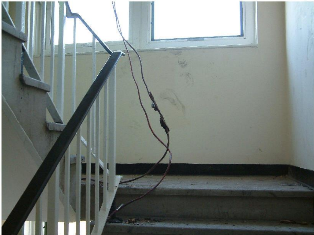
13 th floor stairwell with no smoke damage
