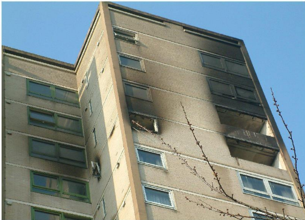
Building side showing missing windows on 14 th and 15 th floor.
