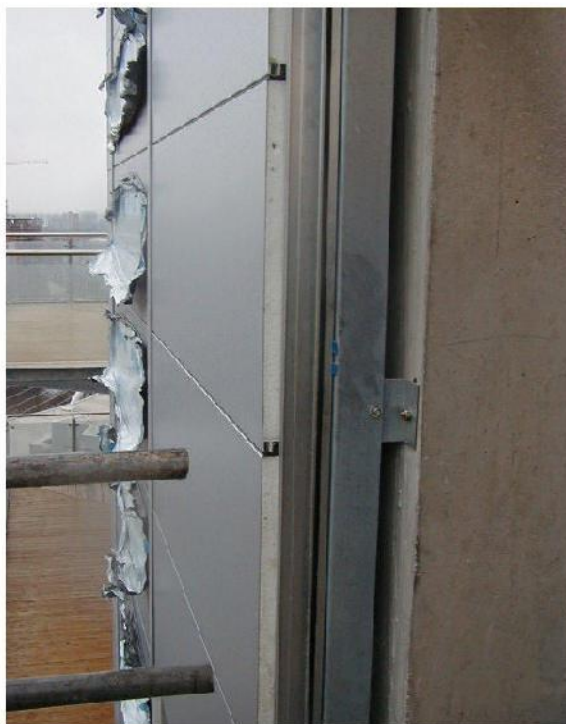
Intact sandwich panel assembly
