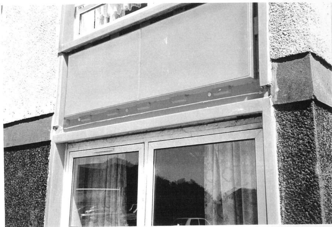
Photograph 3. The living room window of Flat 1. Note the white sealant which has been used to fill the gap at the overlap.
