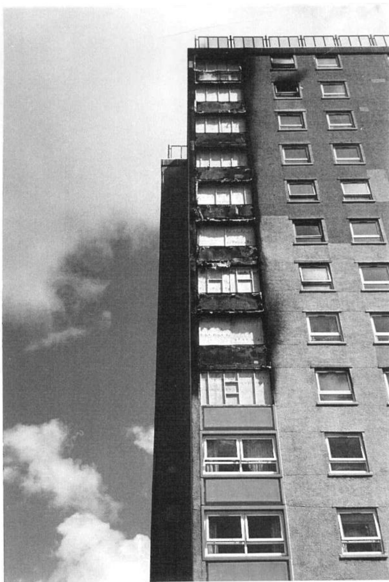
Photograph 1. South Elevation of Garnock Court, showing the external fire damage on the SW side. The lowest level of damage is the fifth floor.
