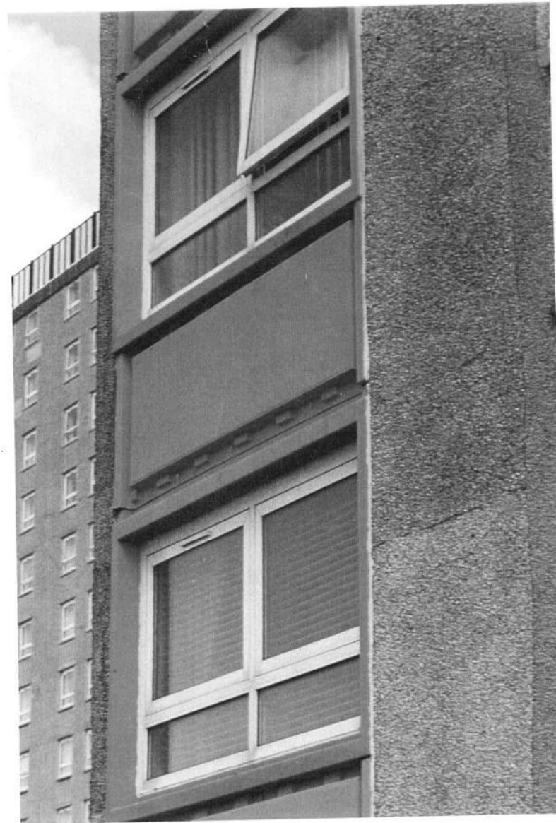
Photograph 2. Detail of the windows on 2 nd and 3 rd floors, directly below the fire damaged section. Note the open window, and the overlapping panel just above the second floor window.
