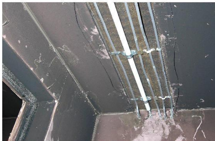
Figure 3 - Close up of cable set fixed to a timber sleeper with the selection of cable supports prior to an experiment
