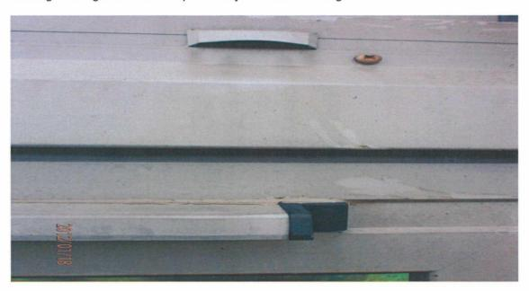
Visible damage to the flat above 123 Taplow House on the 18<sup>th</sup> floor, which shows damage to both the window and rainscreen cladding. It was also noted that Rydon's Maintenance division have replace the glass unit with a temporary replacement.
