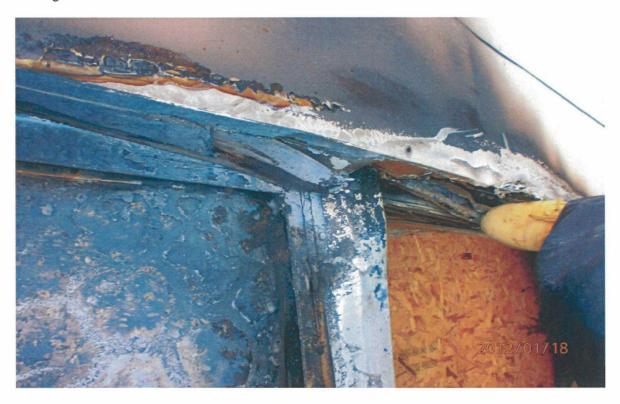
Photograph showing damage to the window vent location on the west elevation 17<sup>th</sup> floor, which has twisted the substructure and damaged the system.
