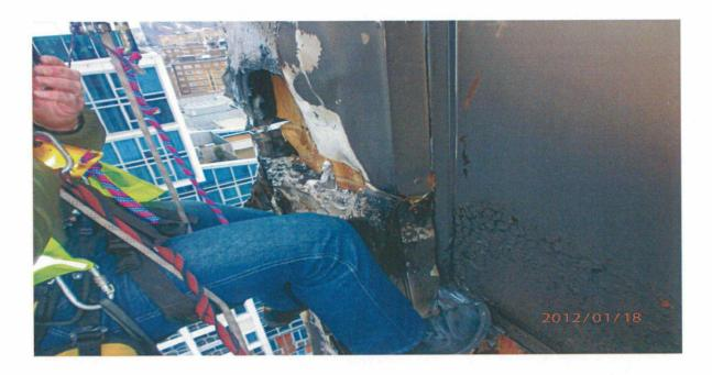
Damage to the bedroom window and surround panels and substructure on the  $17^{\rm th}$  and  $18^{\rm th}$  floors south elevation.
