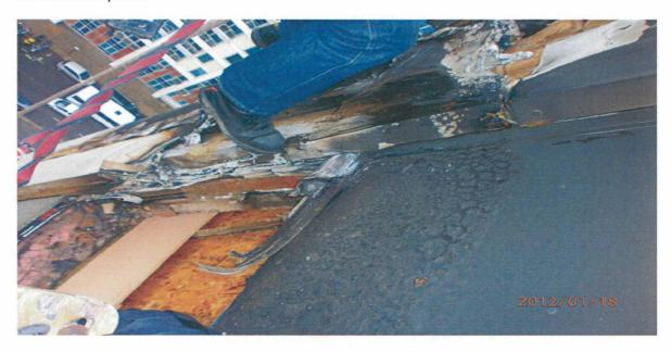
The hot residue from the burning flat has spread down to the 15<sup>th</sup> floor on the south elevation. This has stuck to the panels and burnt the PVDF surface
