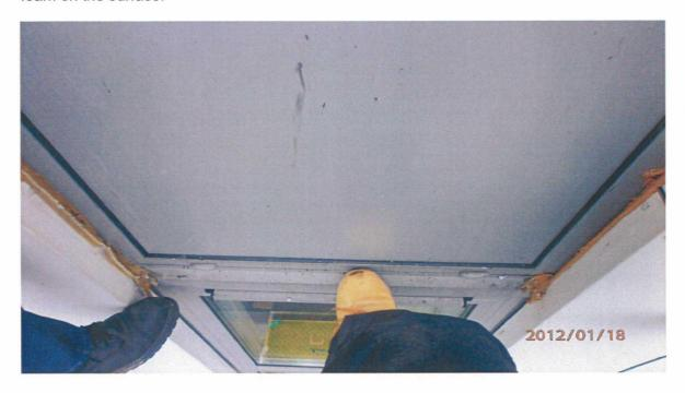
The fire damage to the south elevation appears to be more severe with damage evident on the 19<sup>th</sup> floor window, affecting both the powder coating and active glass coating.
