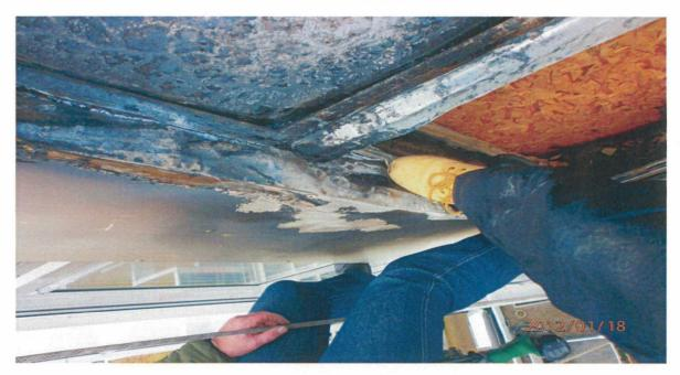
Extensive damage has also occurred to the left hand jamb section of the living room window, where the fire started. The damage includes the panels above and below the flat on the 17<sup>th</sup> floor and includes all panels on the west elevation as it meets the south elevation.
