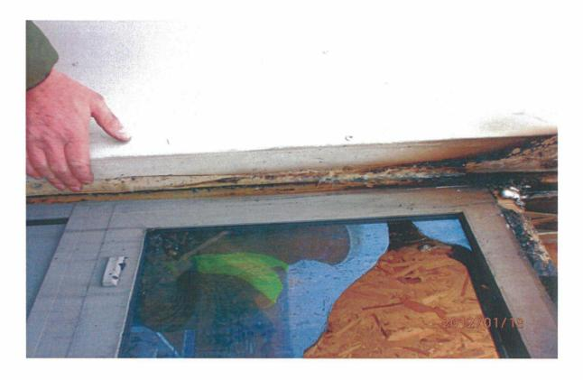
Damage to the window on the 16<sup>th</sup> floor below the fire damaged flat.
