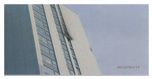
The South Elevation appears to have carried the brunt of the fire as shown on the photograph below. The extent of the fire also includes the flat above and below to the 16<sup>th</sup> and 18<sup>th</sup> floors. Temporary weather proofing will be required to prevent further damage by the weather as the design wind load for this project is said to be up to 2000pa.
