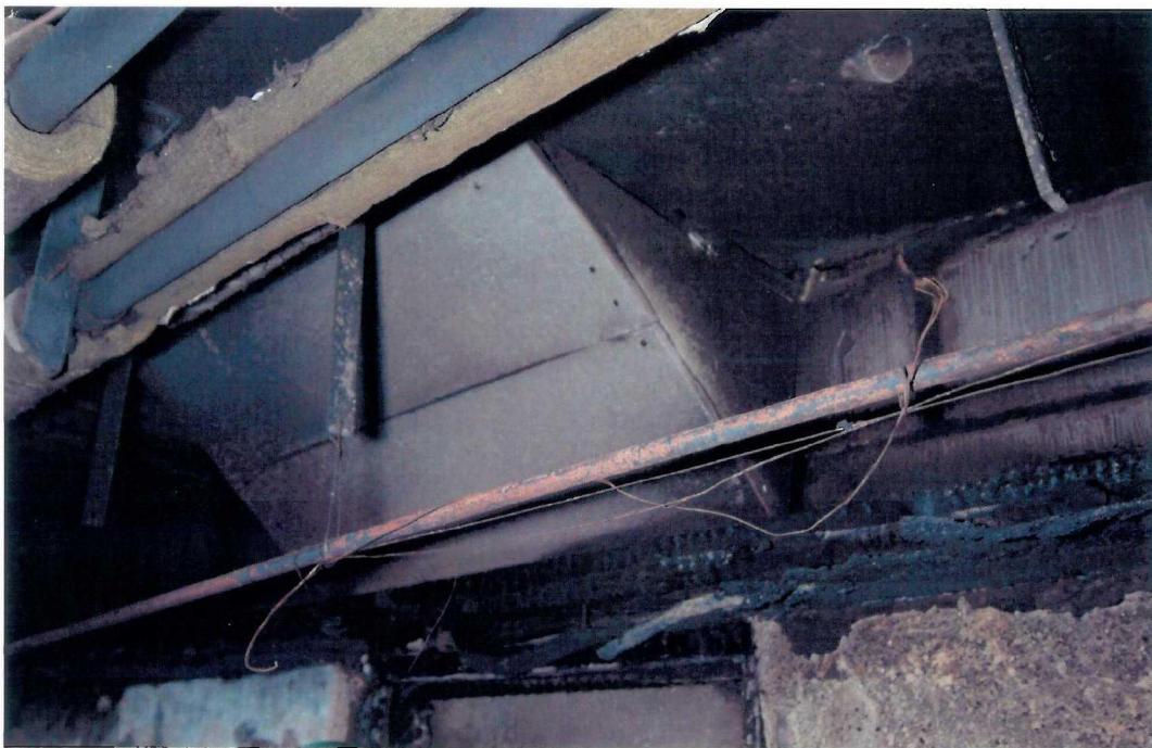
Figure 6 – Mineral board covering staircase cut into corridor ceiling slab.
