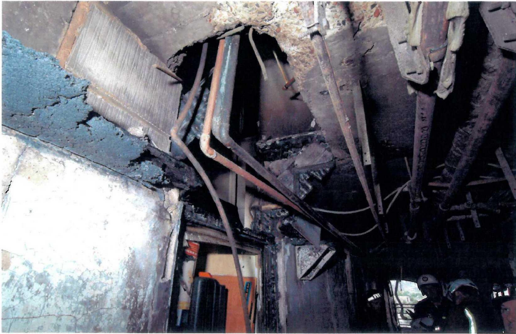
Figure 7 – Hole left by covering falling away and burnt staircase.
