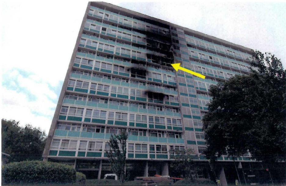
Figure 1 – West face of Lakanal House. Arrow indicates room of origin on 9 th floor. Fire spread to floors below believed by LFB to be caused by drop down of flaming material from window frames.
