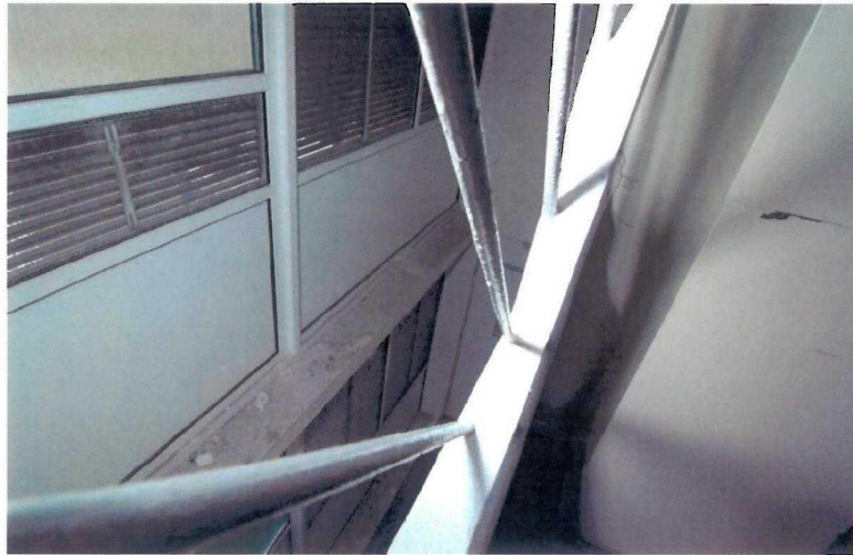
Figure 9 – Lobby ventilation grilles and gap allowing air and smoke movement between floors.
