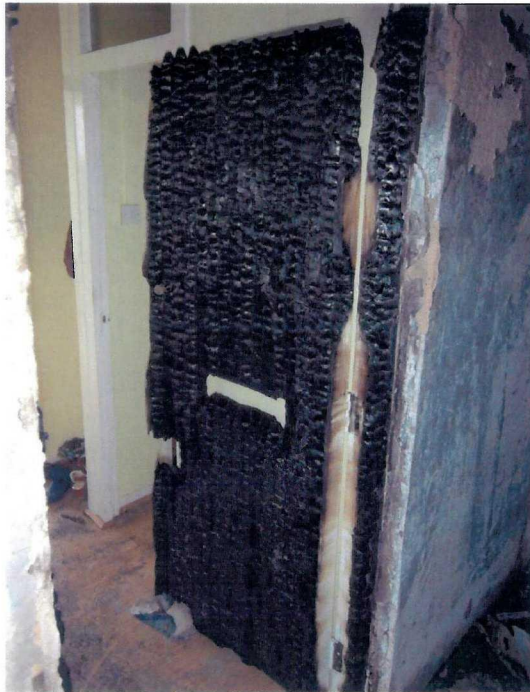
Figure 8 – Heavy charring to flat. Note even depth of char throughout height of door.
