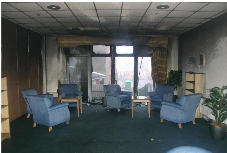
Figure 13 - Fire spread from broken windows controlled by sprinklers (Photograph courtesy of Avon Fire and Rescue Service)
