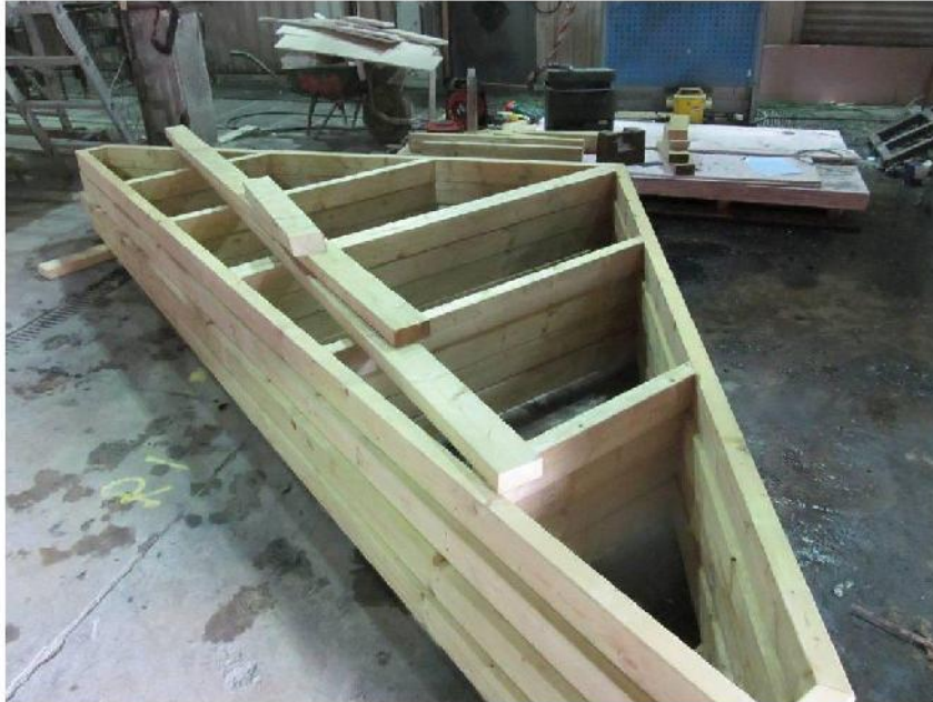
Figure 2 - Timber used to form spandrel panels
