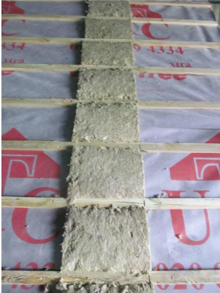
Figure 5 - Insulation between tiling battens prior to fixing roof tiles
