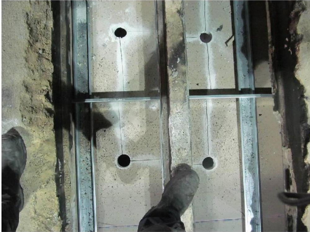
Figure 6 - Holes drilled through plasterboard in centre of fire compartment (The finished roof with the location of the intermediate spandrel panel indicated by yellow paint is shown in Figure 7)
