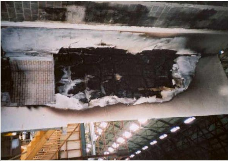
Figure 8 Thermosetting core without adequate fixings or fire breaks
