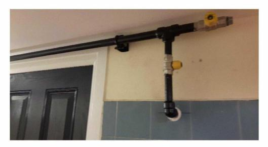
Gas pipe passing through the flat to lift lobby area compartment wall, what fire stopping materials have been used to in fill this hole around the pipe?
