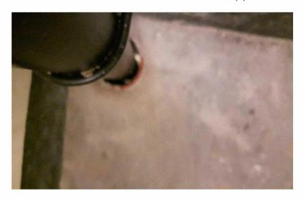
Pipe penetrating the staircase landing, hole through the landing, the hole not made good.
