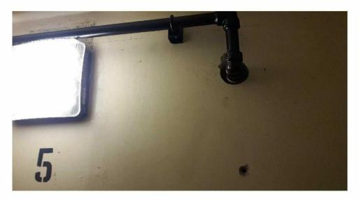
Gas pipe passing through the staircase to lift lobby area compartment wall, no fire collar has been fitted and the hole has not been made good.
