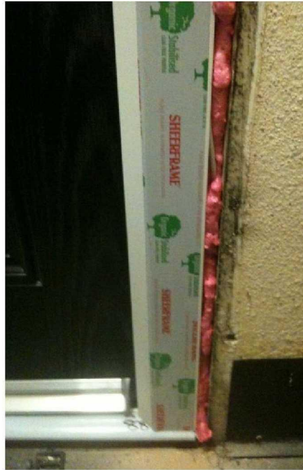
These images illustrate quality of installation, with packers applied next to the fixings.
