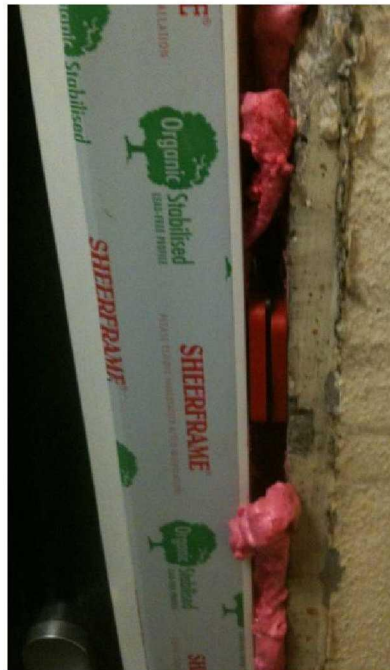
These images illustrate quality of installation, with packers applied next to the fixings.
