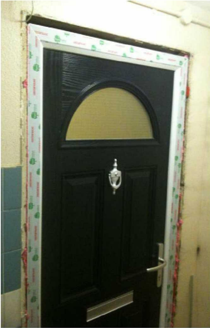
These images illustrate quality of installation, with packers applied next to the fixings.
