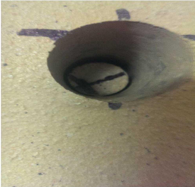
Pipe holes sealed into the flats
