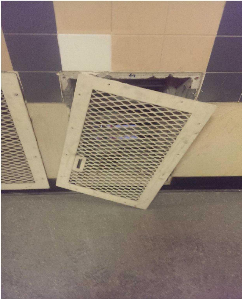
The construction site can be seen through this ventilation grille
