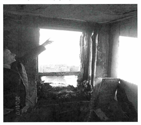
It was evident that despite the fire and the amount of flammable items in the flat such as paper etc. The fire breaks were still intact and prevented the fire spreading between flats. The Harley designed fire break system is visible, now the surrounding fabric has melted under the extensive heat.
