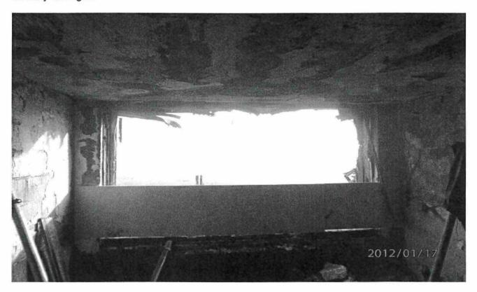
Upon close inspection it was also evident that despite the excessive damage to the whole fabric, which left steel rebar exposed, as the plaster and concreted had melted away. The fire breaks were still intact as shown the photos below.
