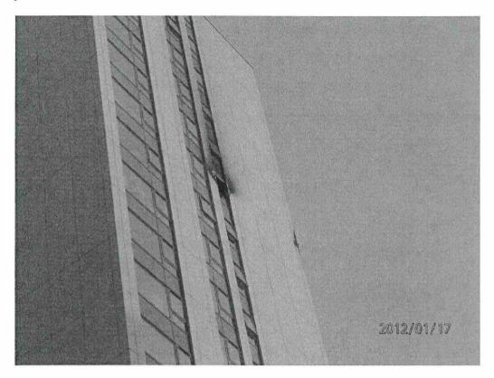
The fire damage was also evident on elevation facing Adelaide Road where the corner of the cladding was also affected. It appears that as the fire had melted the windows the cladding had been damaged by flame spread and smoke.
