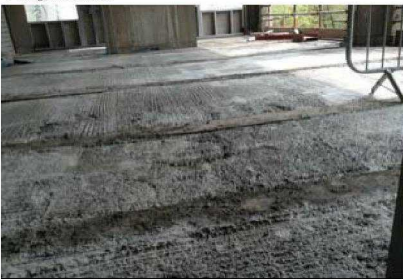
Concrete slab to walkway +1, has now been poured.
