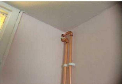
Flat 115 crimped bends now being fitted, and has been installed.
