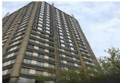
East elevation showing on average 13 floors of windows frames been fitted from the roof down.
