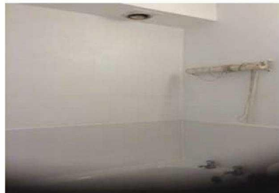
The specification calls for each bathroom ventilation grille and internal duct to be replaced. Rydons to inform all parties when this will start.
