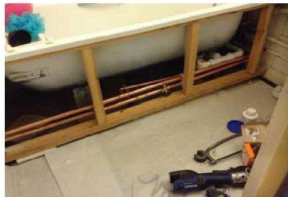
Flat 55, bath pipe work being fitted, and protection has been installed.
