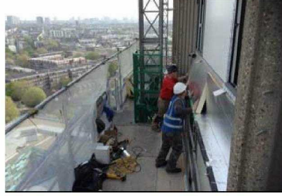
The insulation is being installed on the external cladding.
