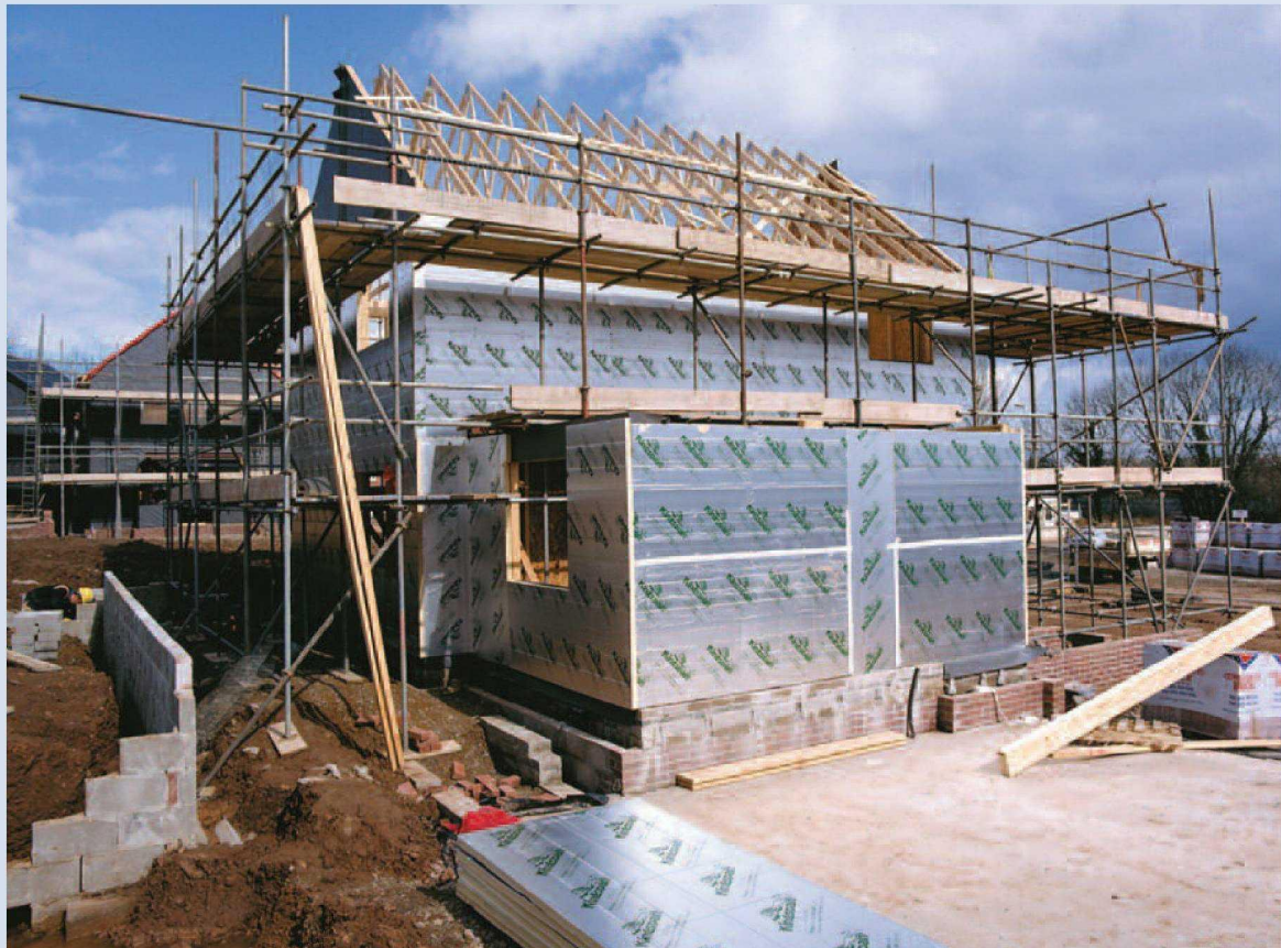
Figure 6: A timber frame building during construction
