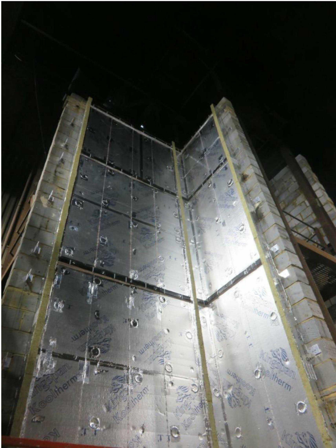
Figure 5. Partial installation of Siderise RH25G 90/30 horizontal open state cavity barriers and Kingspan Kooltherm K15 insulation.
