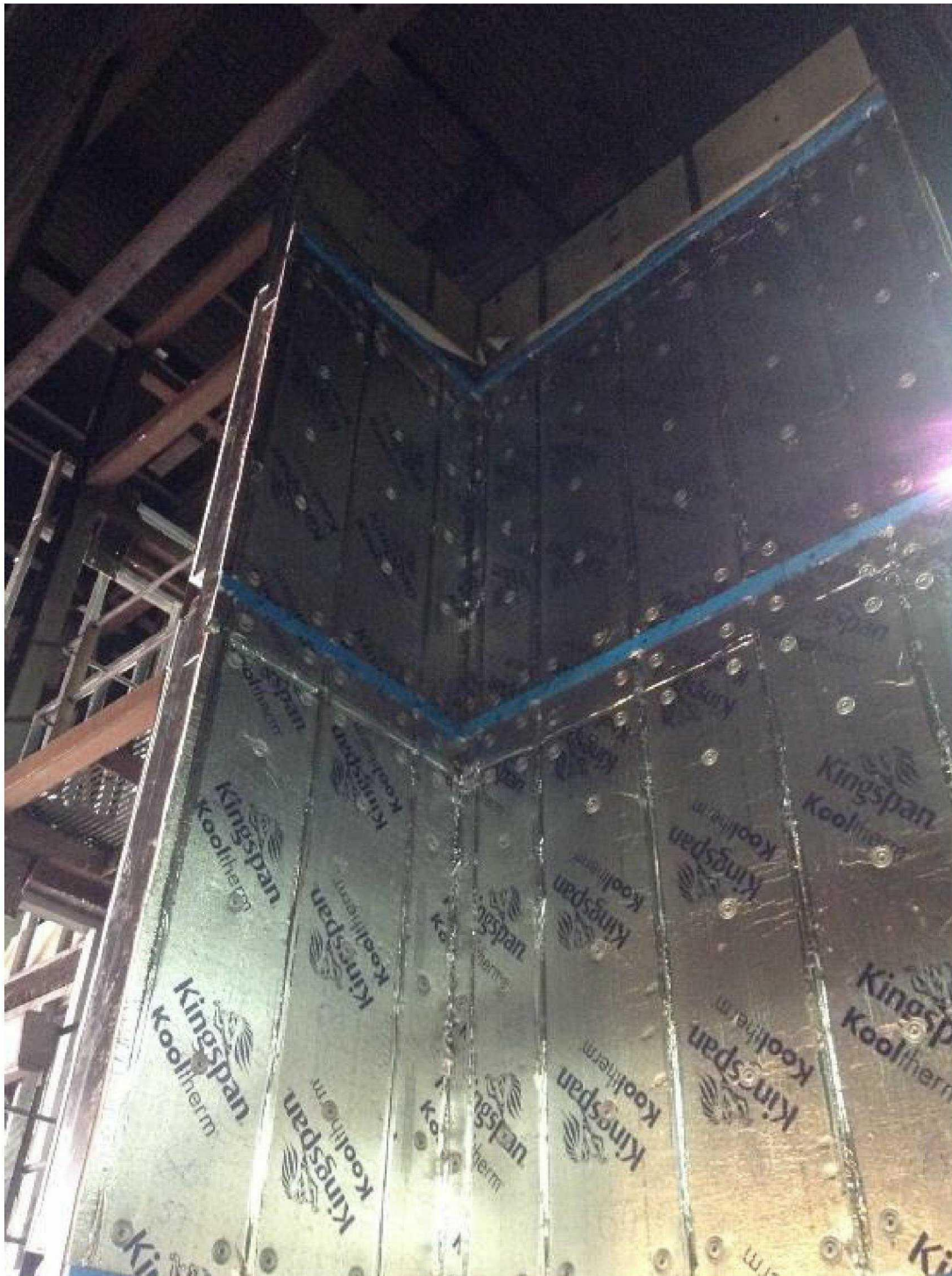
Figure 8. Photograph showing insulation and firebreaks
