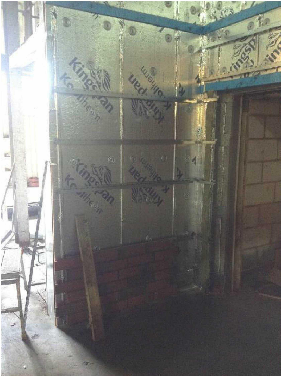
Figure 9. Photograph showing installation of the bricks slips on the support brackets
