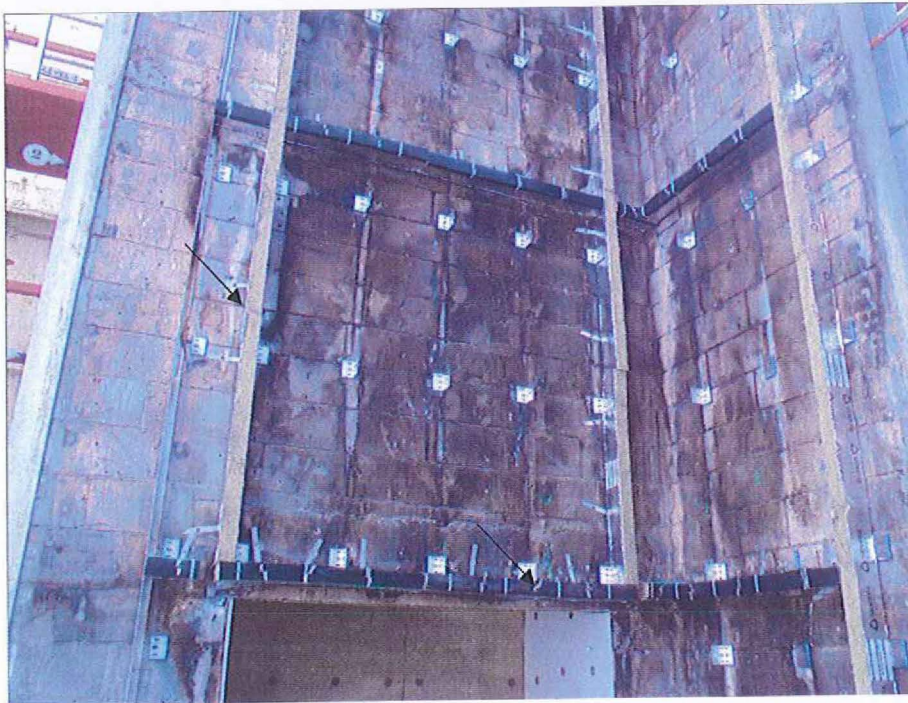
DLP C2753C/6999 Vertical and Horizontal intumescent cavity barrier
