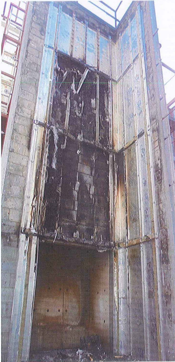
DLP C2753C/0008 Cavity barrier and insulation
