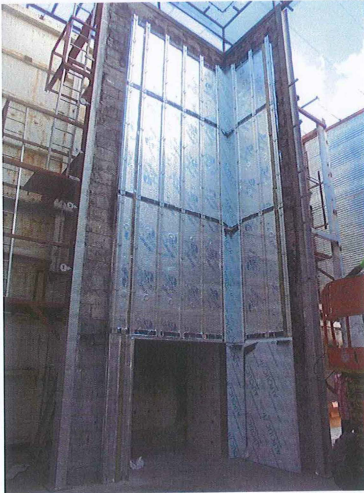
DLP C2753C/4840 Cavity barrier and insulation
