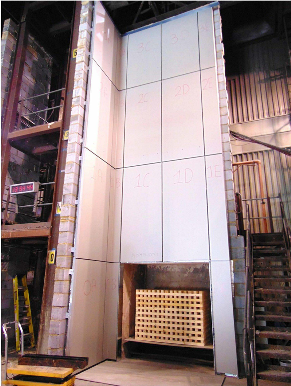
Figure 1. Completed installation prior to test.
