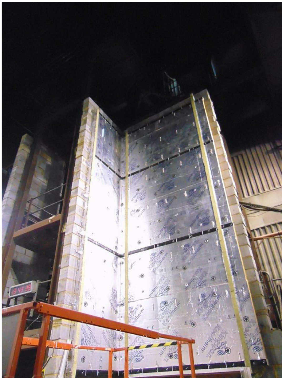
Figure 4. Installation of the thermal insulation, vertical and horizontal cavity barriers
