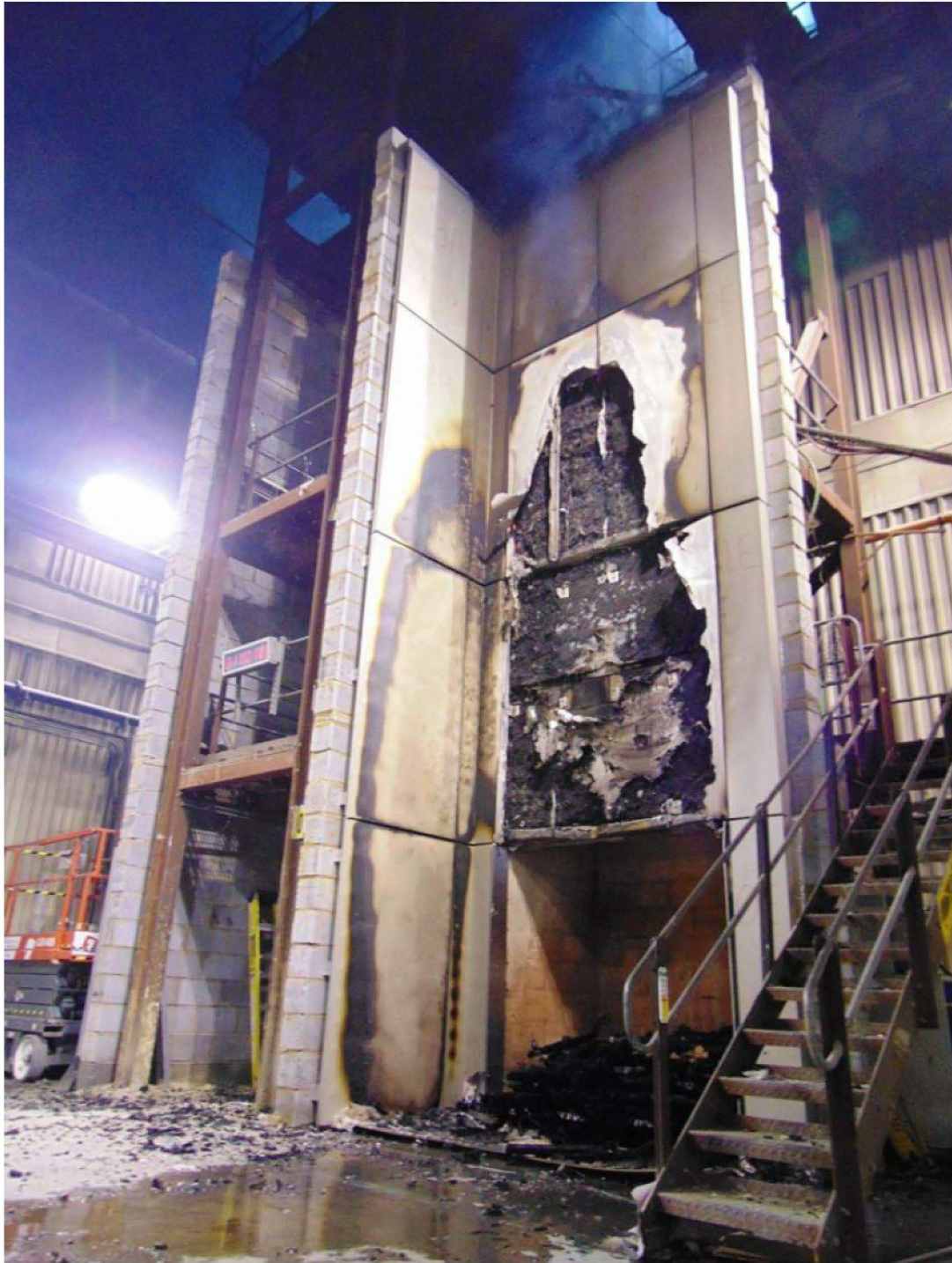
Figure 15. Full height of the system post-test (main and wing wall).
