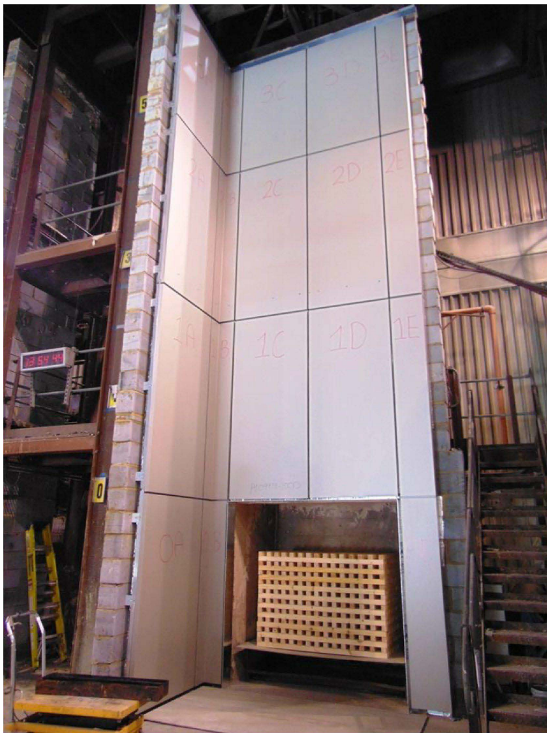
Figure 8. Completed installation prior to test.
