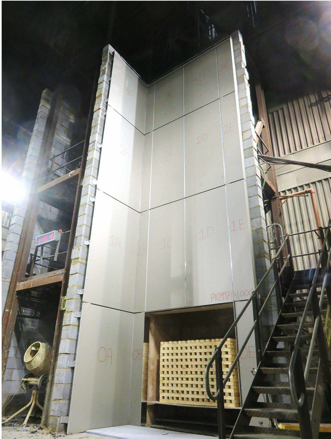
Figure 1. Completed installation prior to test.
