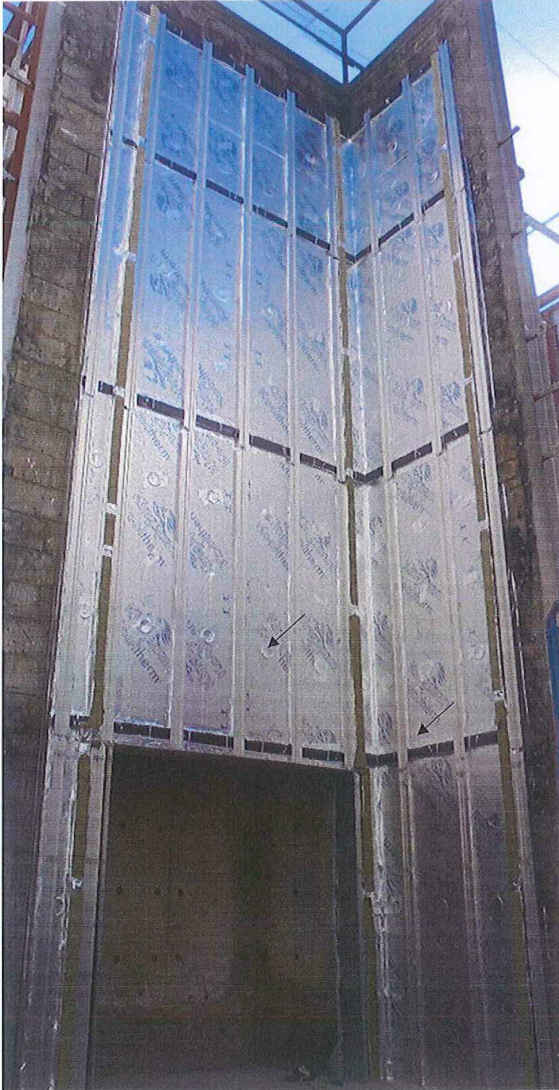
Kooltherm K15 insulation 100mm & aluminium foil tape
