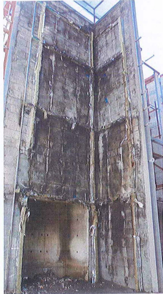
View of the cavity barriers
