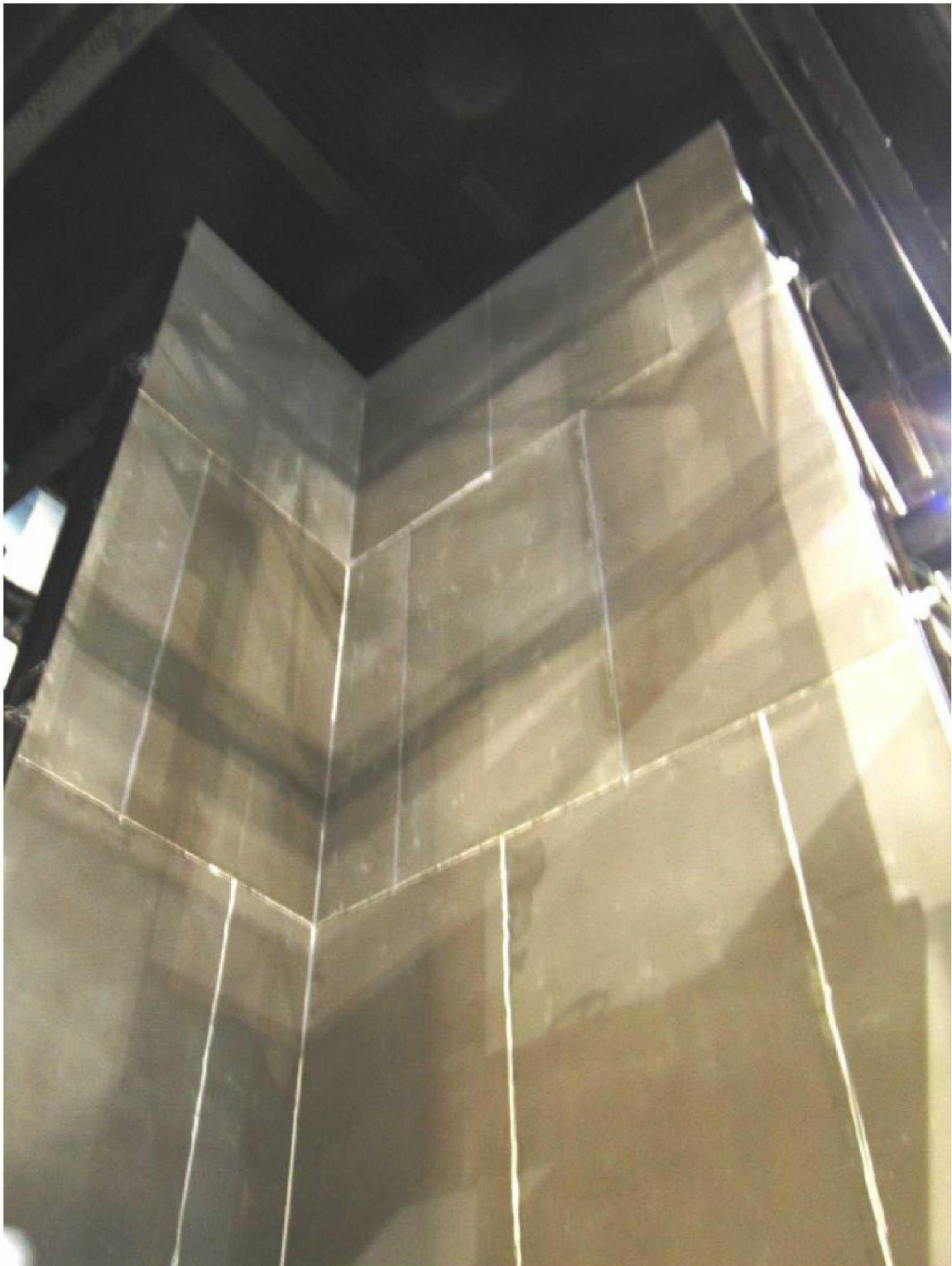
Figure 5. Cement particle board fitted to external face of Kingframe partition.
