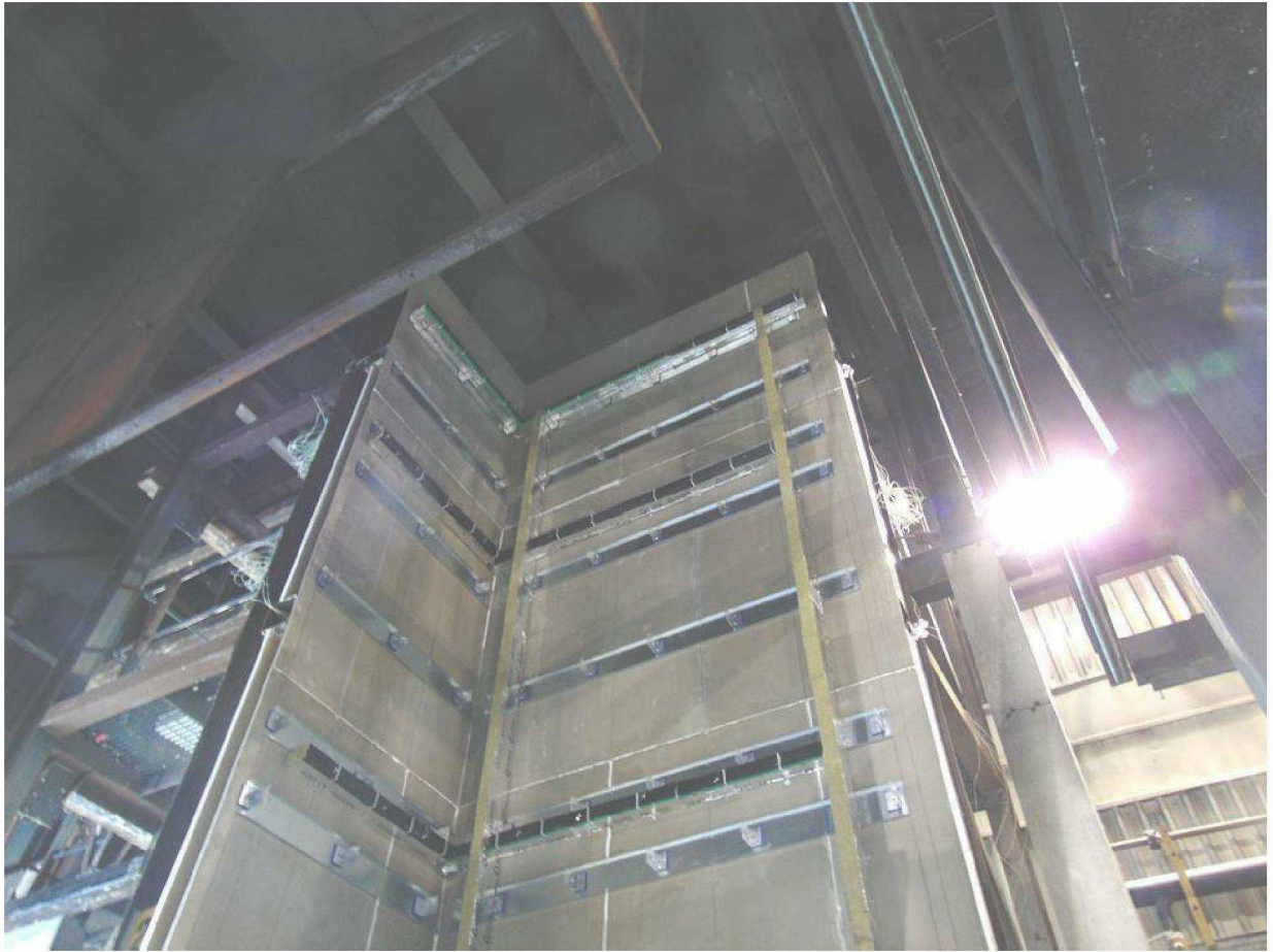
Figure 6. 'U'-shaped channels and 'L'-brackets fitted to cement particleboard.
