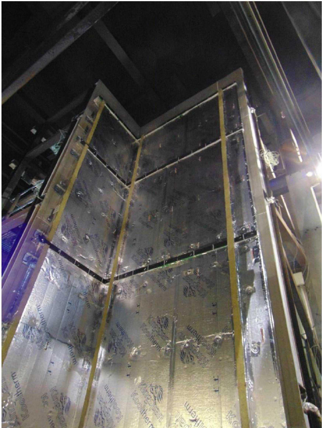
Figure 7. Insulation and cavity barriers fitted to system.
