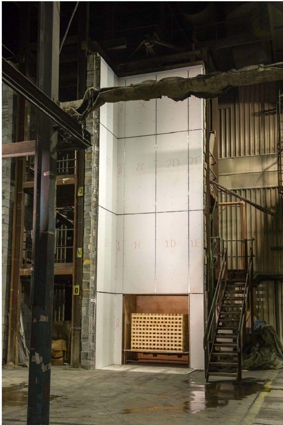
Figure 12. Completed installation prior to test.
