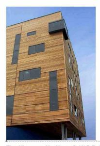
The Kingspan Kooltherm® K15 Rainscreen Board is lightweight and achieved the required U-value for the Quadrus Centre in South Tyneside. The Architect specified the material as it had the ideal properties for a built-up rainscreen system.
