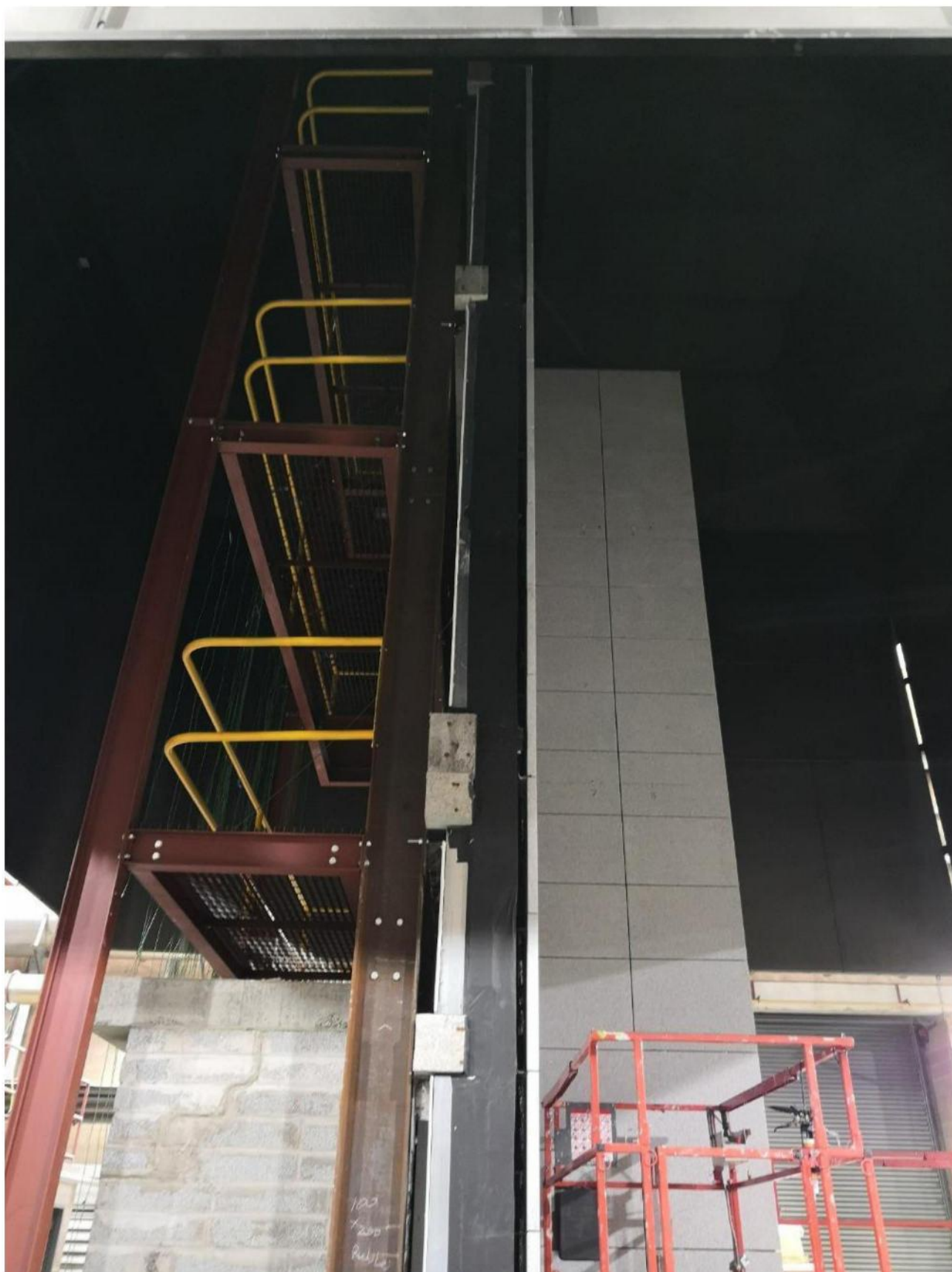
Figure 4.9. Cladding system before test. Wing face.
