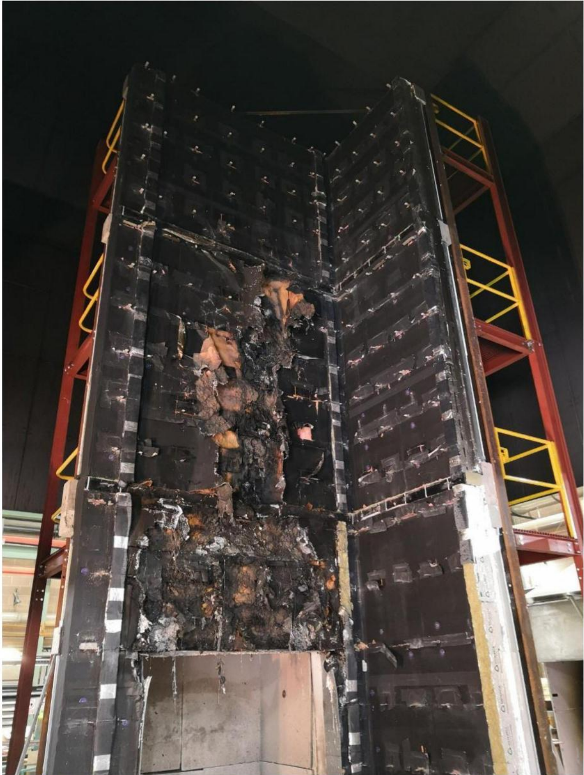
Figure 4.16. Post-examination damage. Insulation mainly charred and burnt above the combustion chamber on the main face; intact on the wing face. Vertical fire stop barriers in-place with some damage on the one located right of the chamber.
