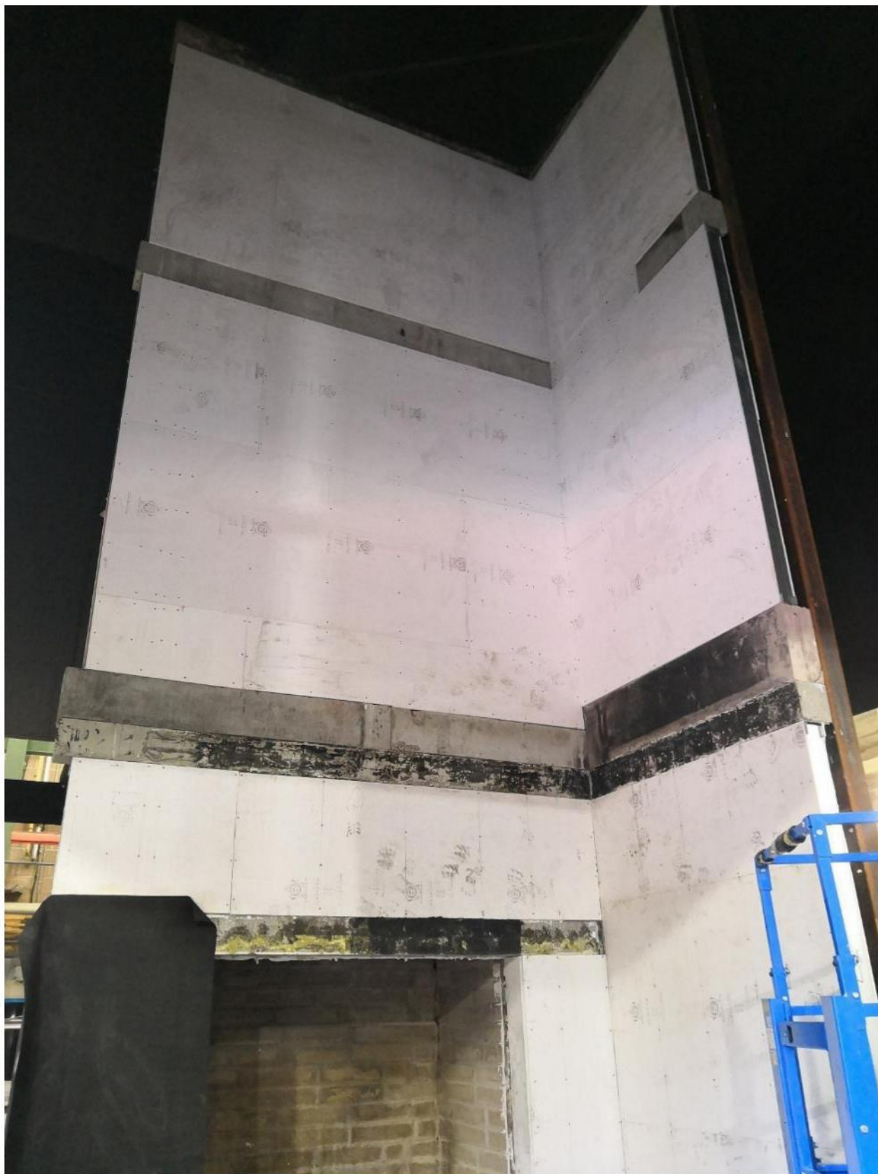
Figure 4.4. View after completing sheathing board layer mounting during construction. Start of waterproof membrane installation.
