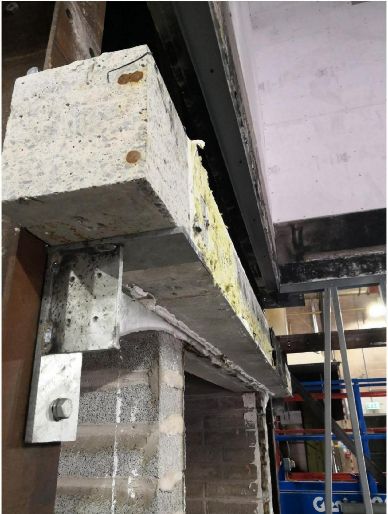
Figure 4.2. Installation of concrete lintel in front of combustion chamber's lintel on the main face during construction.
