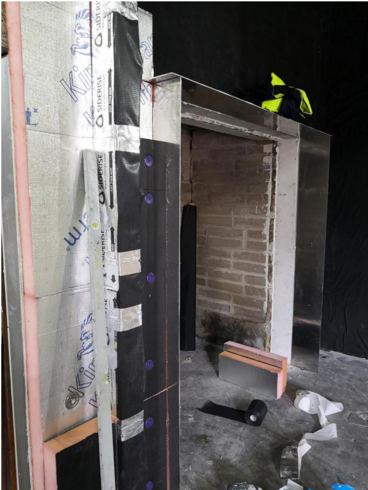
Figure 4.6. Close view of insulation and vertical fire stop barrier installation.
