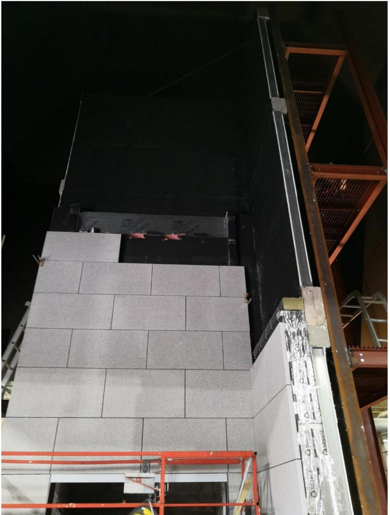
Figure 4.7. Installation of stone cladding panels during construction.
