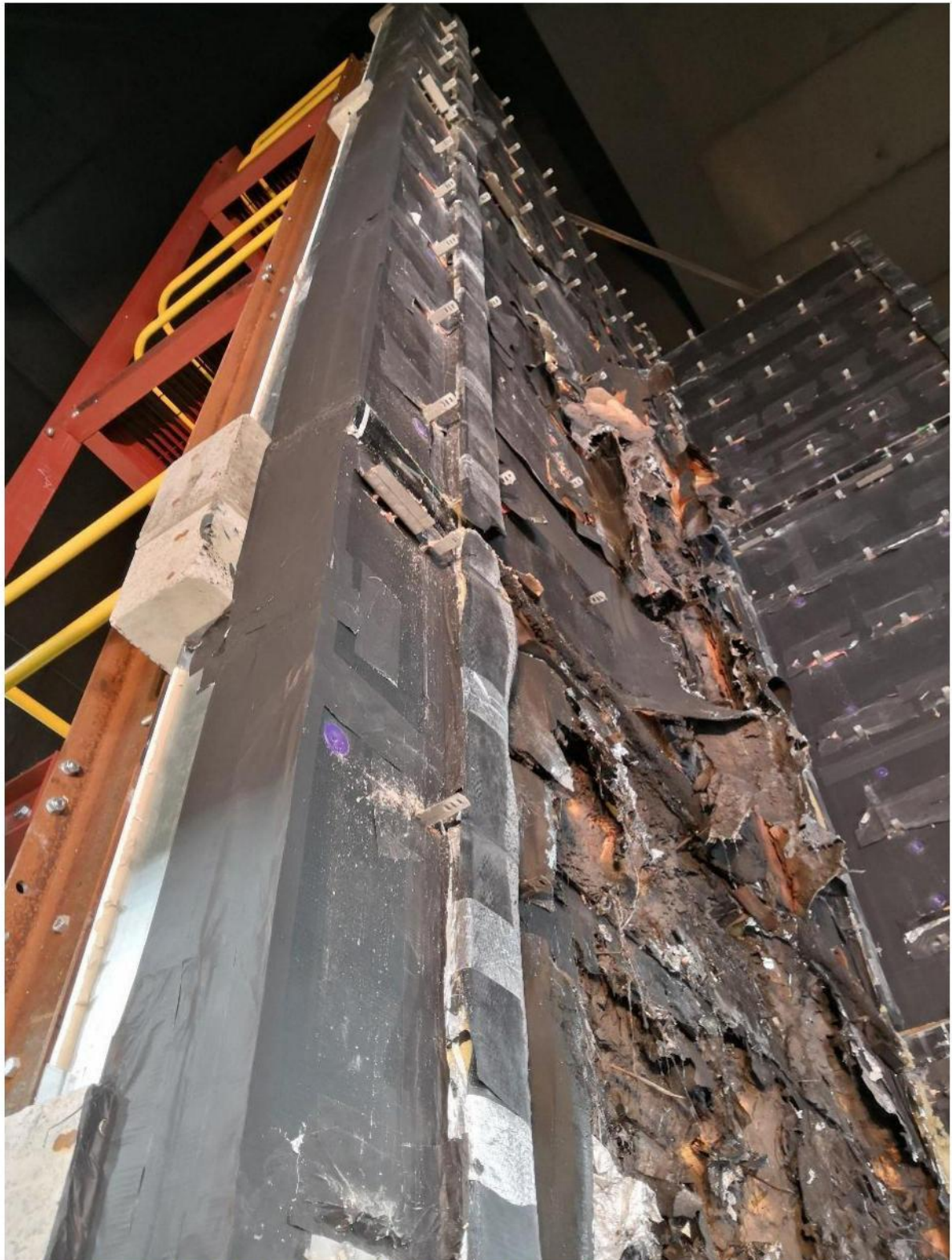
Figure 4.19. Post-examination damage. Vertical fire stop barrier located on the left-hand side edge of the system's main face. No damage observed; in-place and intact.
