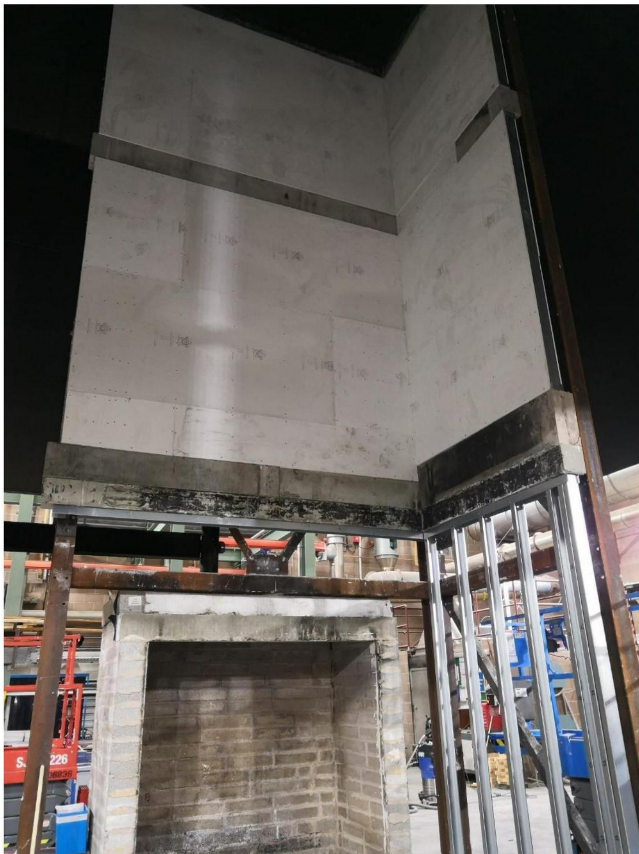
Figure 4.3. Insulation of SFS Kingframe and sheathing board layer during construction.
