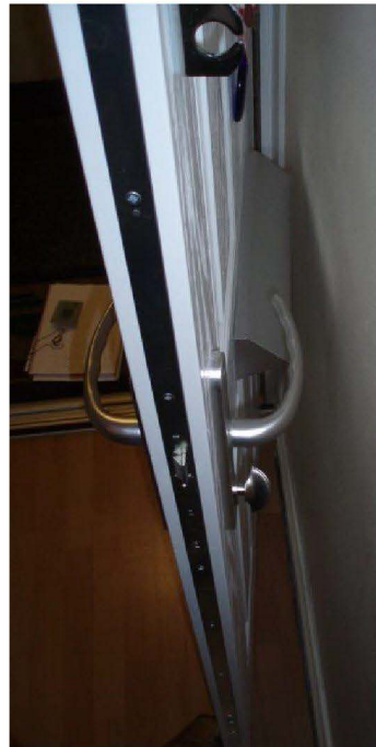
Door hardware, including handles, lock, chain keep and letter box cowl.
