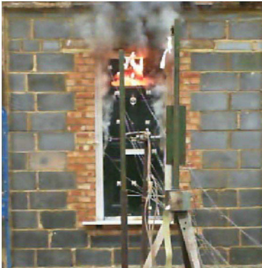
Exposed face of specimen at time of first integrity failure (15 minutes).
