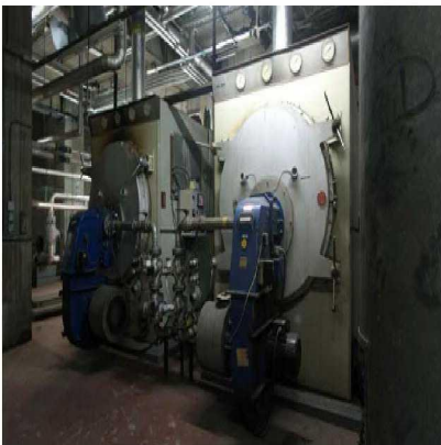
42 The 40-year-old boilers under Grenfell tower serving all of Lancaster West 1.
