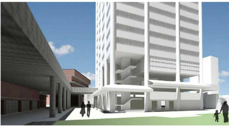
Existing South West View
