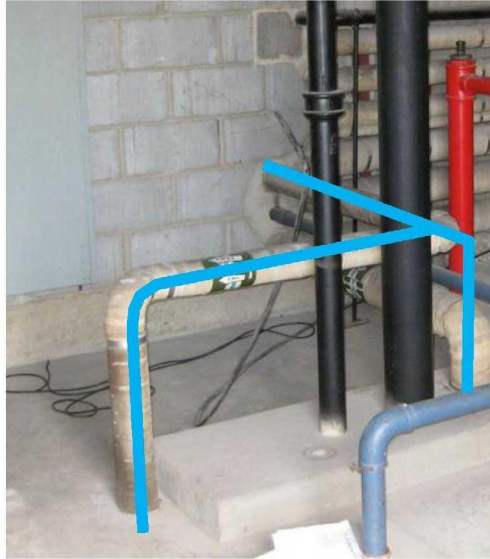
Figure 8-4 - Blue line shows potable water supply connected to existing non-potable supply
