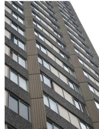
Existing façade precast spandrel panels and column cladding
