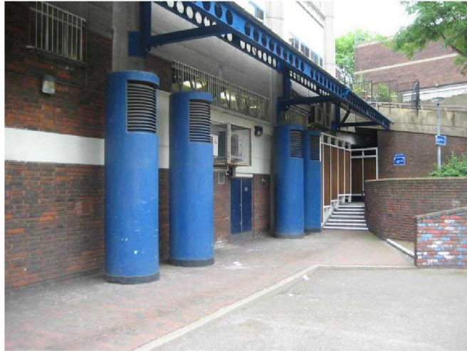
Existing external canopy fixed to the RC columns
