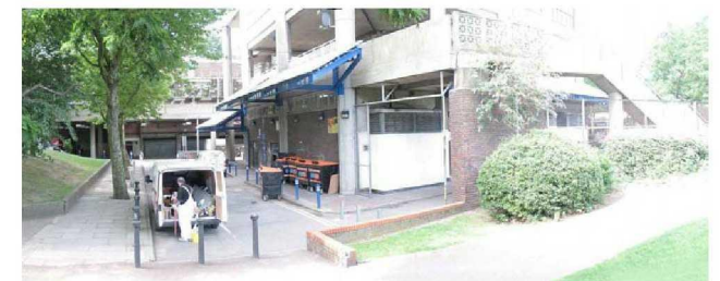
Fig. 5 Service Access to east side of tower
