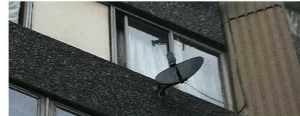
Figure 2-1 - External wiring for communal satellite system
