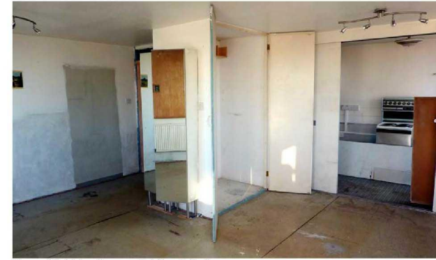
Figure 14. Living Room – Existing 2 Bed
