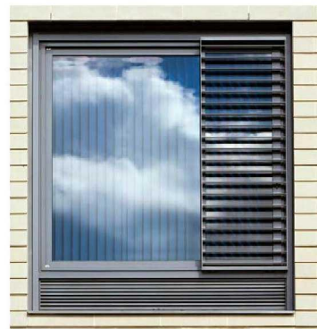
Fig. 26 Grille to purge vent
