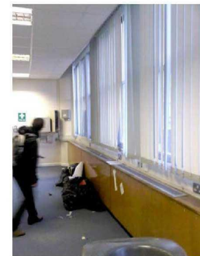
Walkway +1 - Vacant offices
