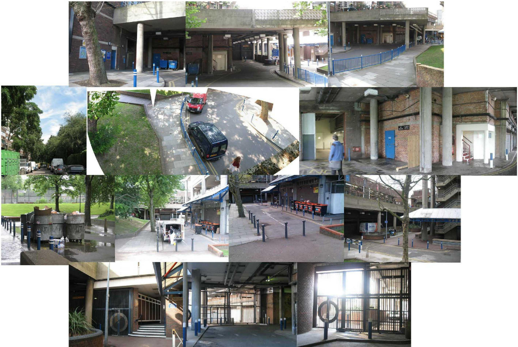
Figure 11 Views showing vehicle access to the undercroft of Lancaster West and around the base of Grenfell Tower
