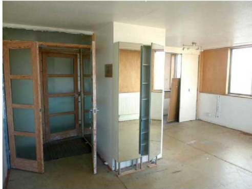
Figure 15 Living Room looking towards kitchen – Typical 2 Bed
