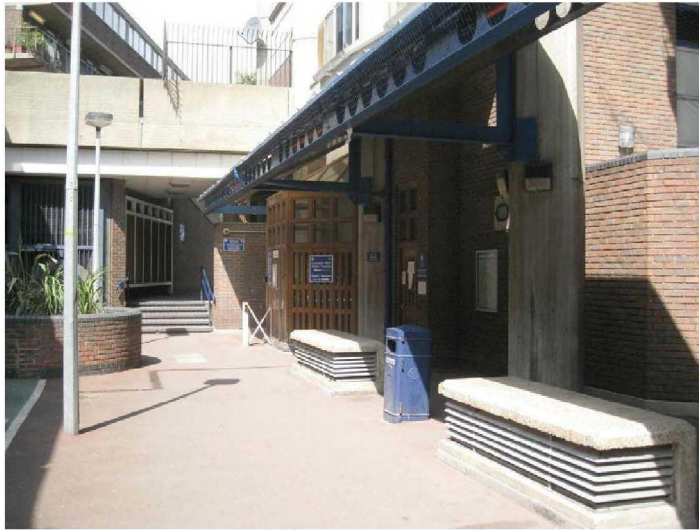
Figure 35 Existing approach to tower entrance
