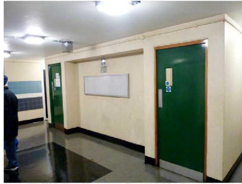
Figure 13. Lift lobby – Fire escape door on right, refuse chute on left
