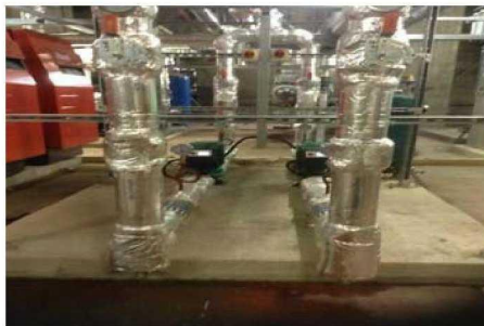
The new pipes to the basement have been lagged, but need to be clad.
