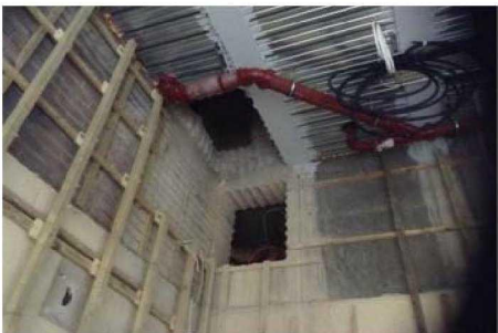
All the AOV holes are cut out except two to do. The extract ducting will not be on site for some 4 weeks.
