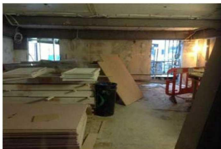
The ground floor openings have been formed, and the partitions and M&E 1st fix have also started.
