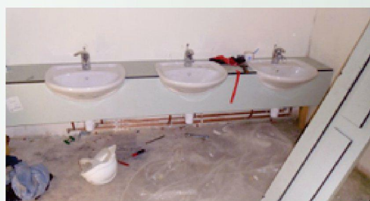
Fitting out of the nursery
