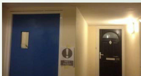
The redecoration of all 20 lift lobbies is underway
