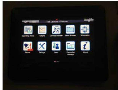
Basement boiler panel is still yet to be installed fully. Can Rydons confirm why 142 alarms have been activated. Still no Schematics have been installed. Rydons have now confirmed the date to start commissioning the boiler controls, etc, has been moved from Friday 13th, to a later date.
