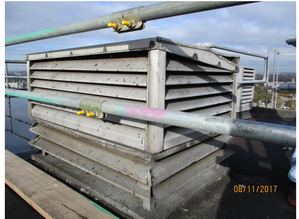
Weatherproof housing/roof vent on Roof above north smoke shaft
