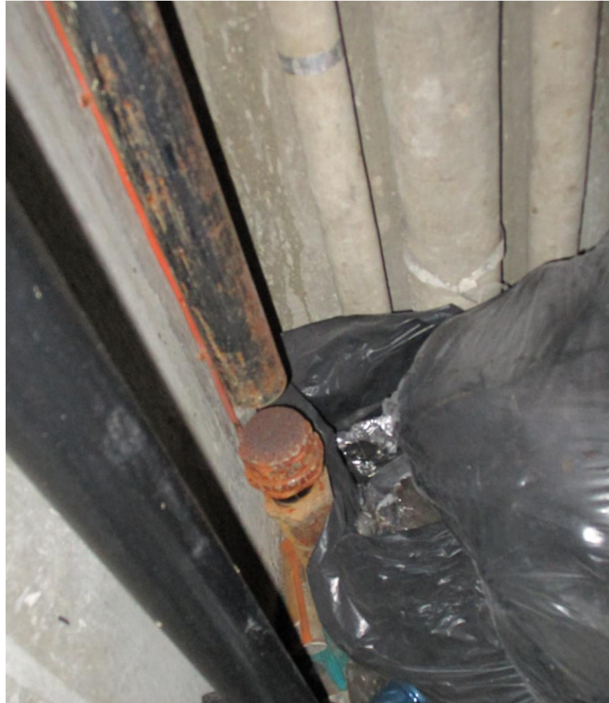
Decommissioned gas riser – original residential gas supply Capped on Ground Level
