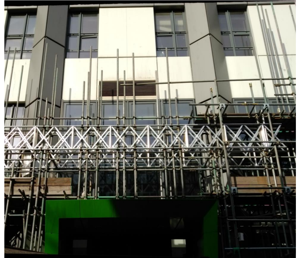
Vent on Level 2 for south smoke shaft
