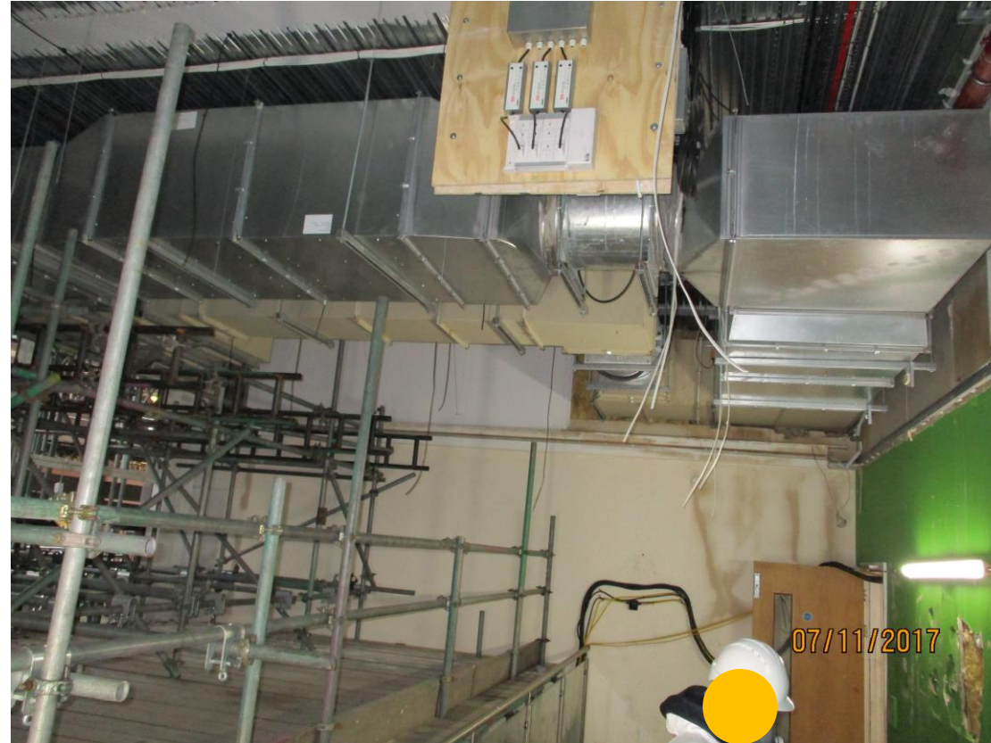
Ductwork at Level 2 for south smoke shaft
