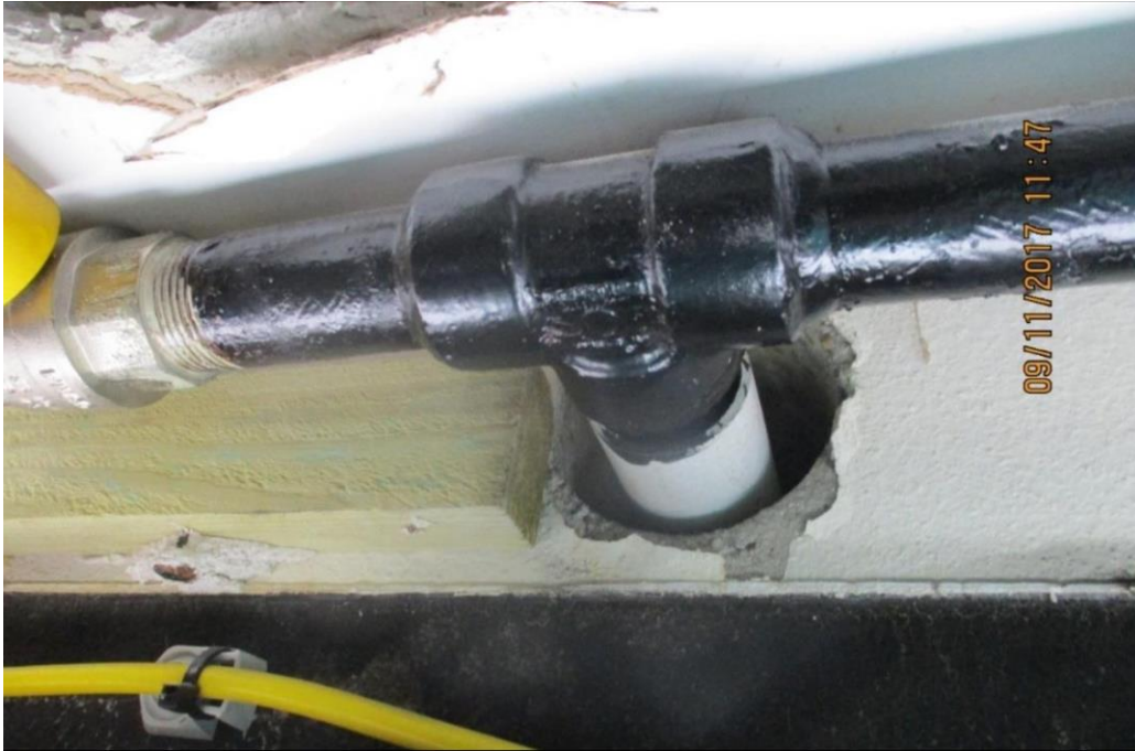
Gas pipe penetration through stair compartment wall
