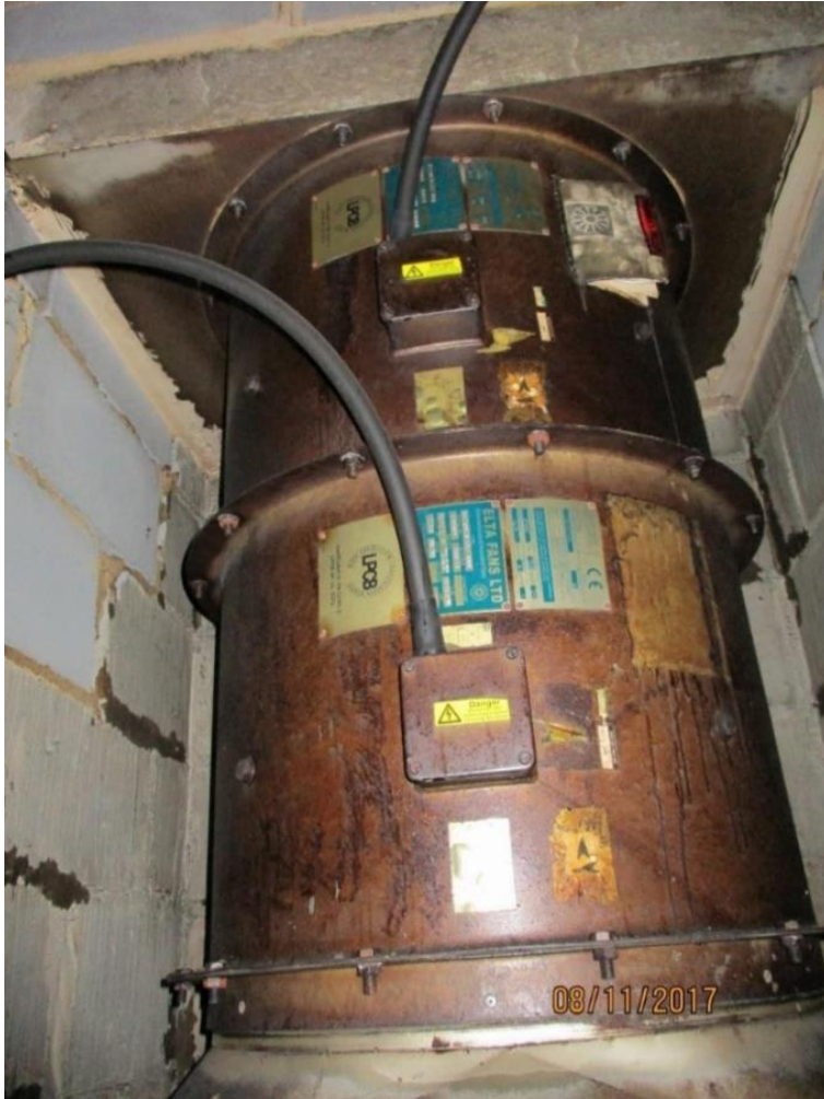
Environmental fan and smoke extraction fan in Rooftop Plant Level
