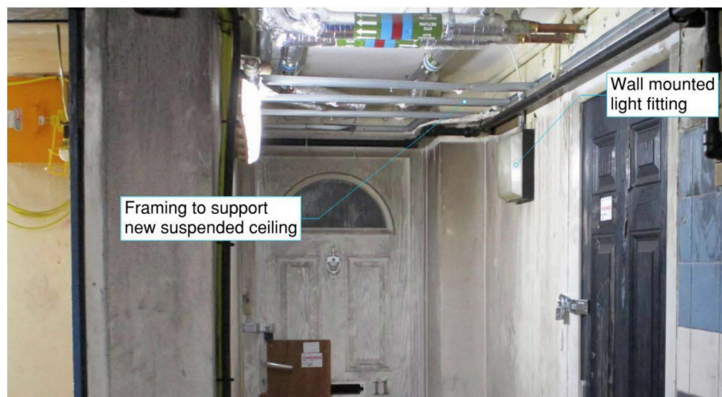
Figure G.46: Evidence of new suspended ceiling (Level 4 corridor, south side of lobby)
