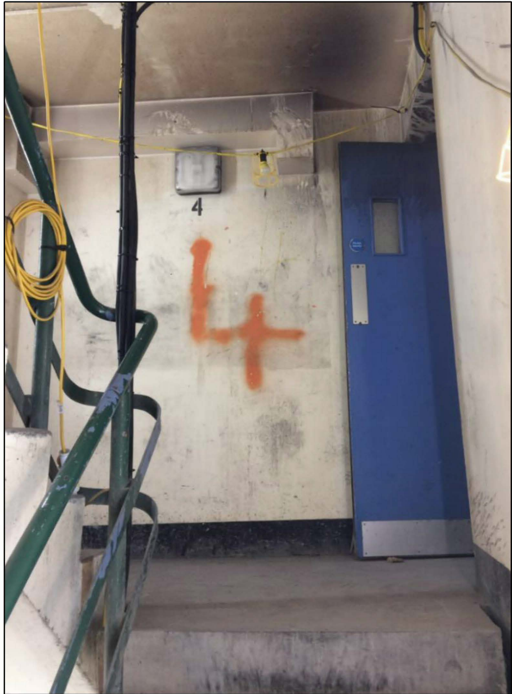
Figure G.31: Level 4 stair landing showing handrail on one side of stair only
