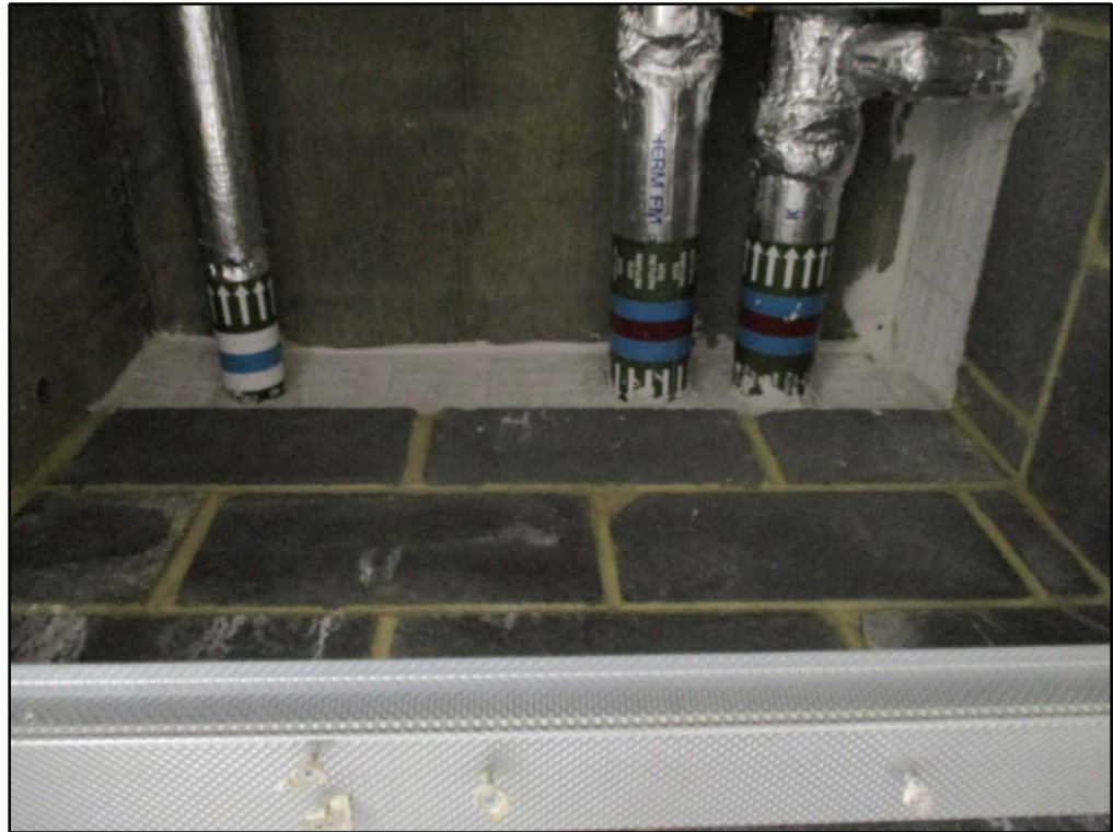
Figure G.32: Insulated pipes in protected stair on Level 3
