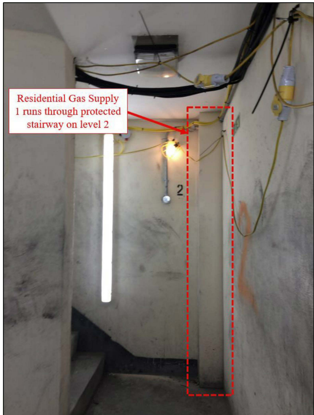
Figure G.33: Enclosed gas piping in protected stair from Levels 2 – 22
