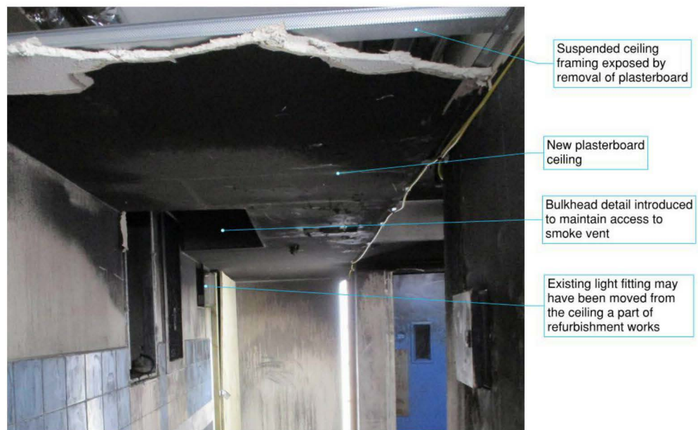
Figure G.45: Evidence of new suspended ceiling (Level 4 corridor, north side of lobby)
