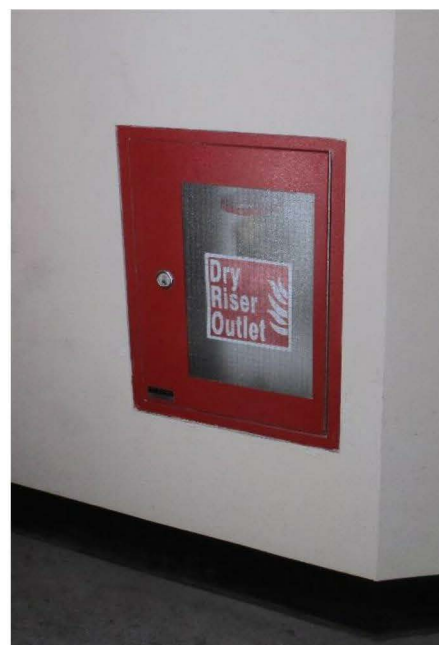
Figure H.21: Example fire main outlet on Level 1
