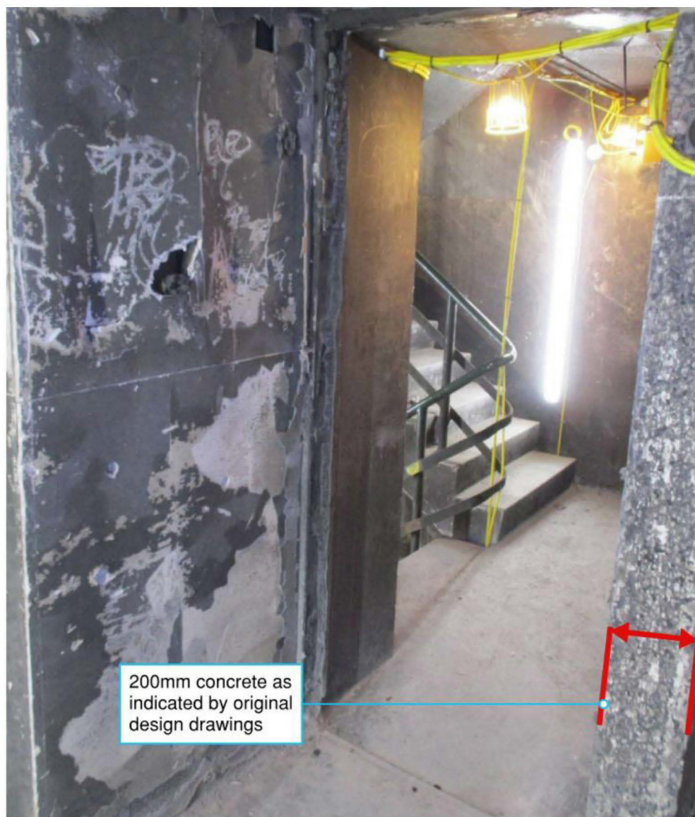
Figure H.36: Photograph of Level 20 stair door showing concrete enclosure of stair
