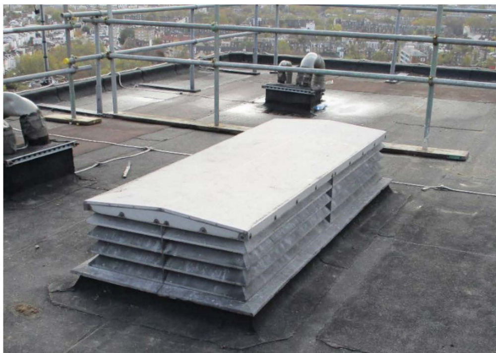
Figure H.Figure H.2829: Permanently open vent at head of stair, observed 8th November 2017
