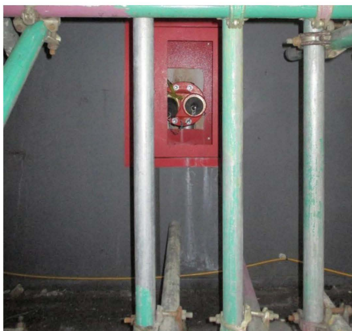
Figure H.20: Dry fire main inlet at Grenfell Tower
