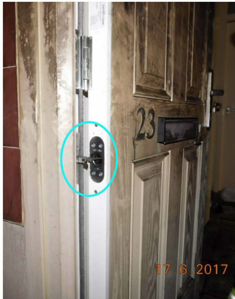
Figure I.17 Door closer on flat 23 (circled in blue) was attached (MET00018892)
