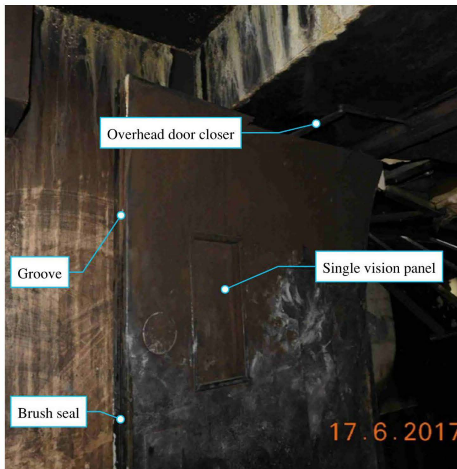
Figure I.29 Level 11 stair doors (MET00018873)
