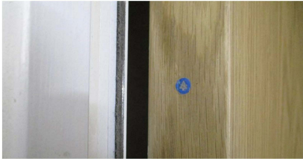
Figure I.35: fire door marking on entrance door to Flat 7 (Level 3)
