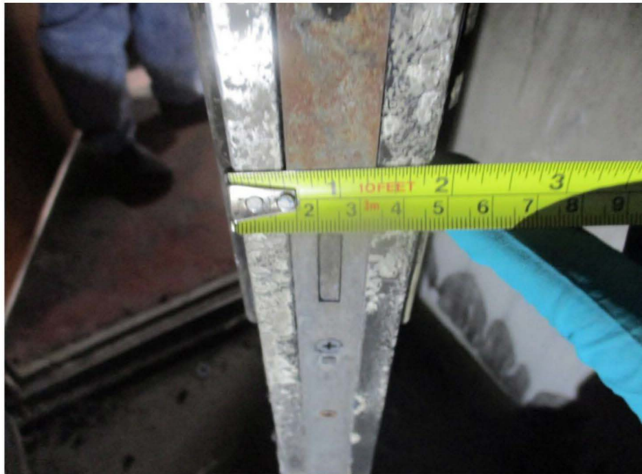
Figure I.11: 44mm door leaf (photo from Flat 26)
