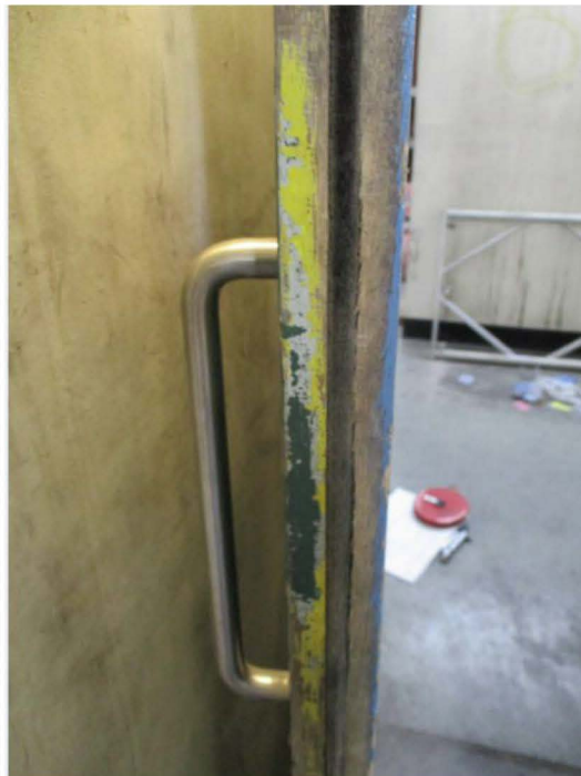
Figure I.26: Level 6 stair door (brush seal present, unknown if intumescent seal present below brush seal)
