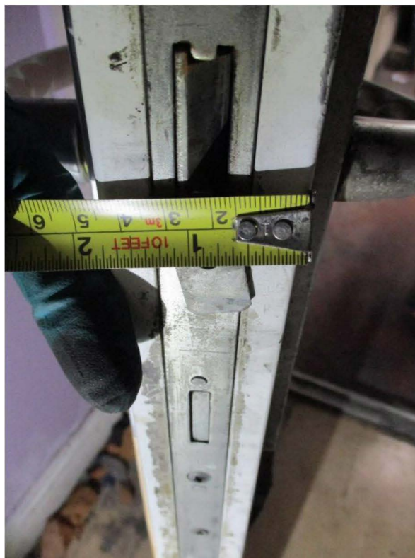
Figure I.13: Example lock (from Flat 24)
