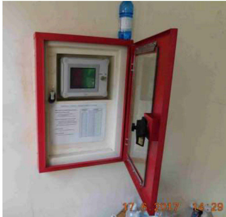
Figure J.40: HMI panel, located in the Entrance Lobby, photographed on 17 June 2017 showing key switched to the 'On' position. (MET00018915).
