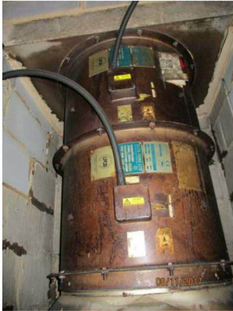
Figure J.27: Environmental / Smoke control fans in the roof plant room
