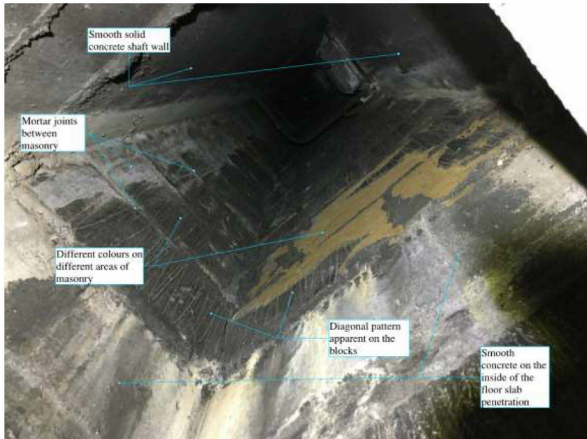
Figure J.19: Inside of shaft at Level 7
