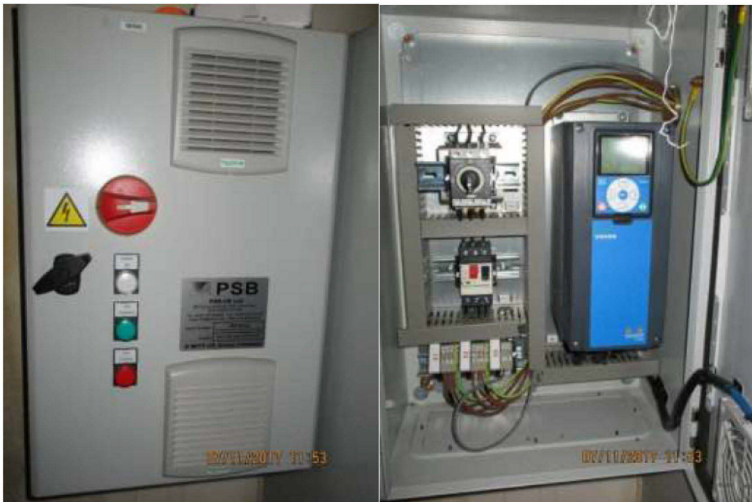
Figure J.44: Environmental fan inverter panel located in the Ground Floor Hub Room
