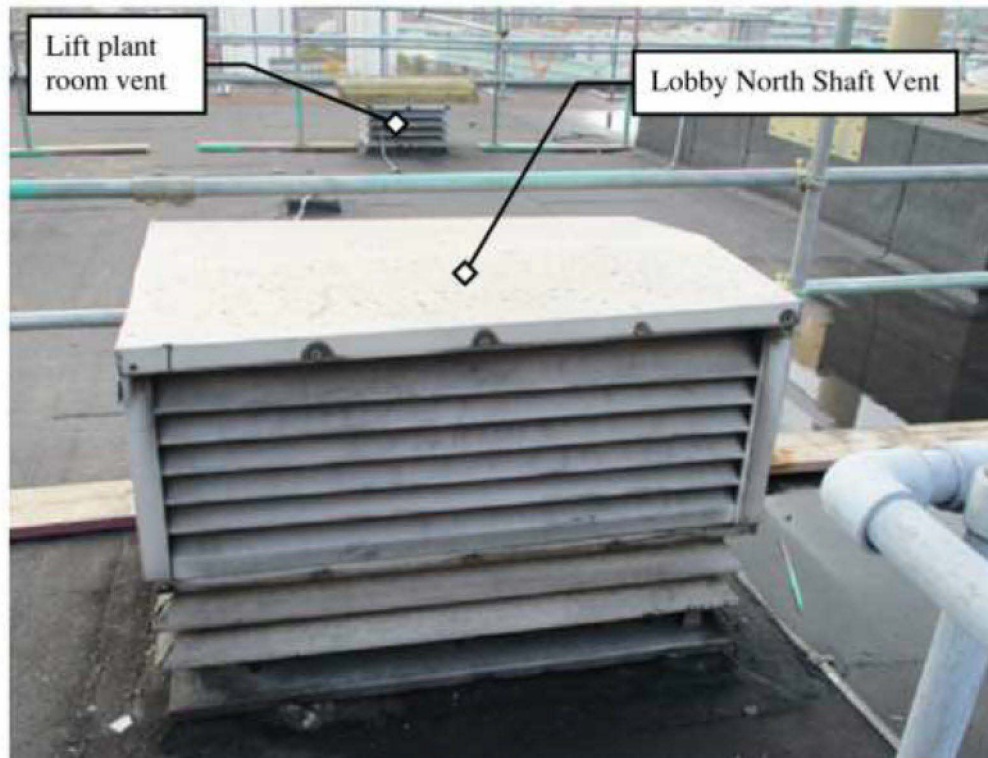
Figure J.30: North vent shaft outlet
