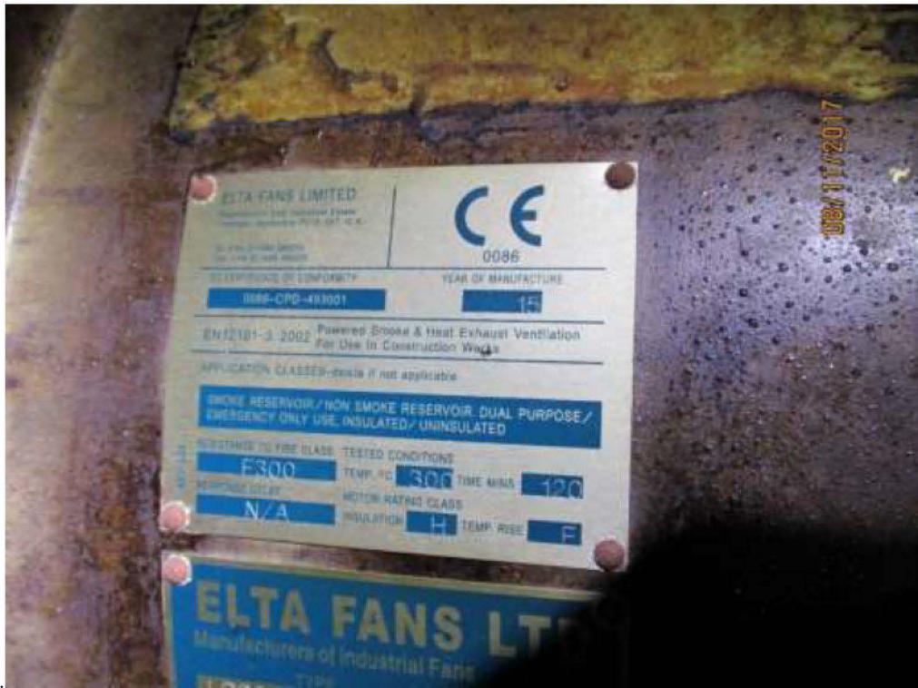
Figure J.28: Post fire inspection of fan information plates stating that the temperature rating of the roof smoke fans was 300°C for 120 minutes.
