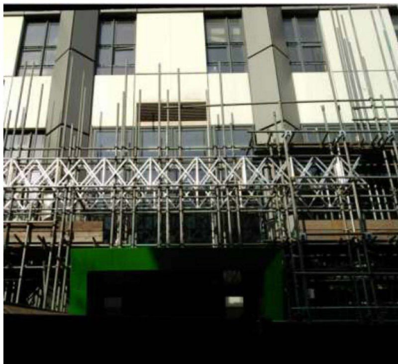
Figure J.36: Smoke system intake / exhaust louvre at Level 2. In smoke mode, smoke will be exhausted from these louvres. In environmental mode, fresh air will be drawn into the building through these louvres (BLA00004531).
