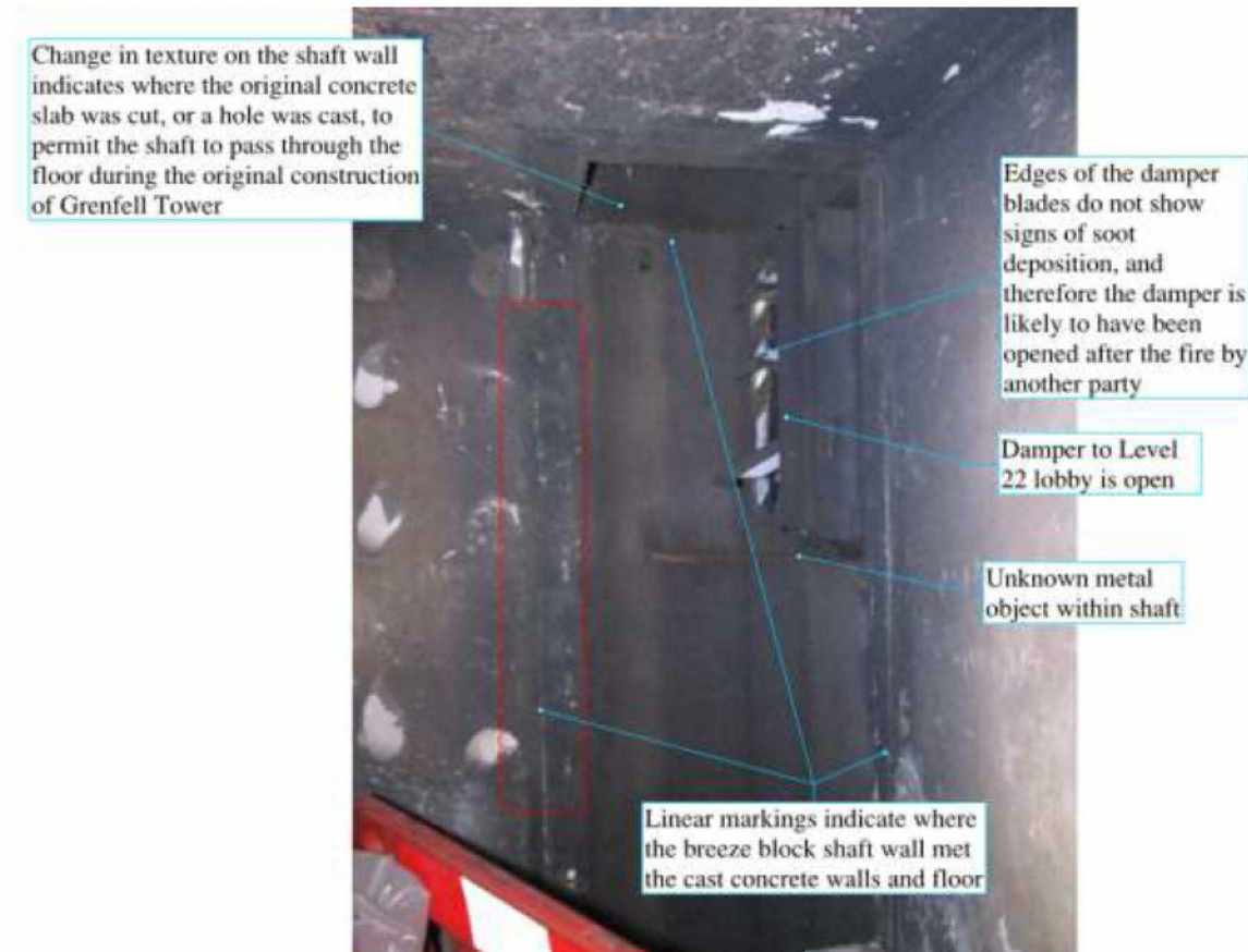
Figure J.26: Destroyed smoke shaft in flat 195 on Level 22
