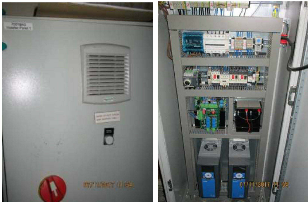
Figure J.45: Inverter panel for the smoke fans located in the Ground Floor Hub Room
