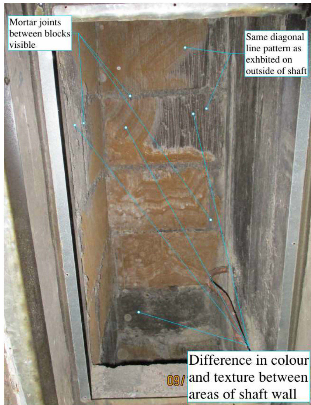
Figure J.16: interior of smoke shaft at Level 7
