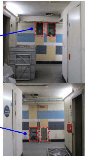
Figure J.1: Assessment of the requirements of A2.03(1) GLC Section 20 Code of Practice 1970 for staircase and lobby ventilation against the provisions in Grenfell Tower
