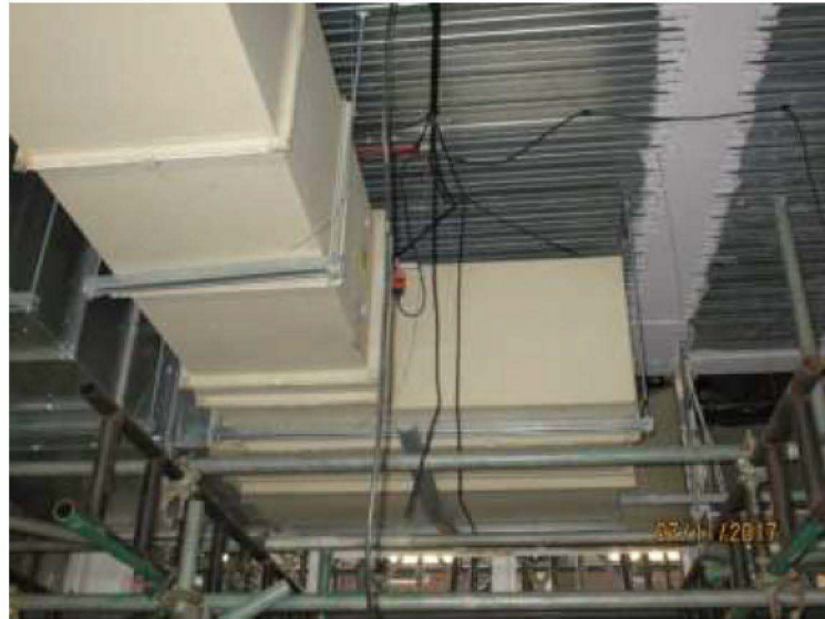
Figure J.35: Fire-rated ductwork at level 2.
