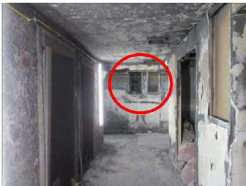
Figure J.21: North AOVs on Level 16 (My photo. Please refer to Appendix C).
