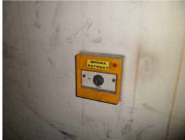
Figure J.42: Fire fighter override key switch on Level 6.
