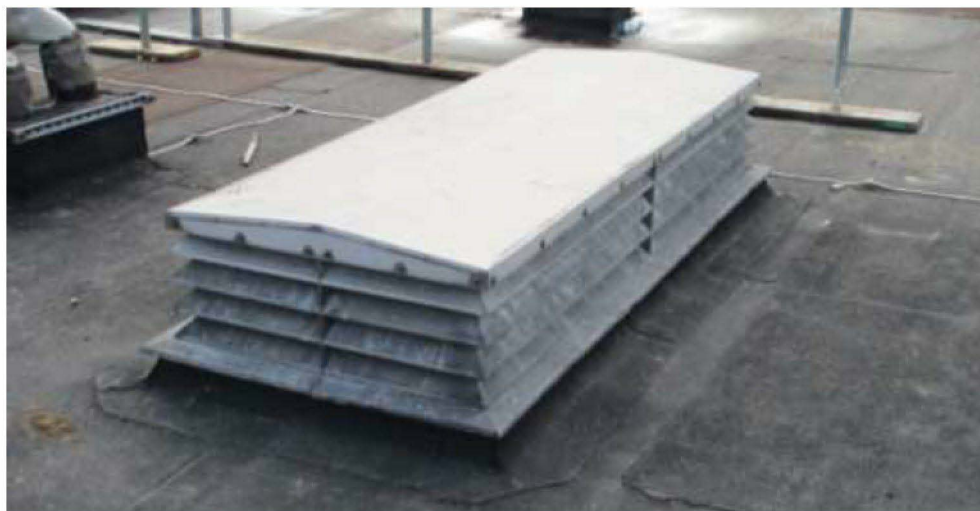
Figure J.31: Permanently open vent at head of stair
