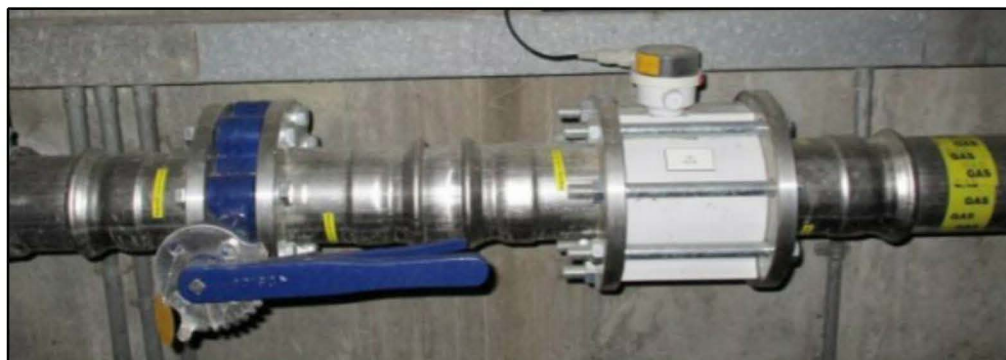
Figure K.12: Isolation valve and meter for the gas pipework serving the new boilers
