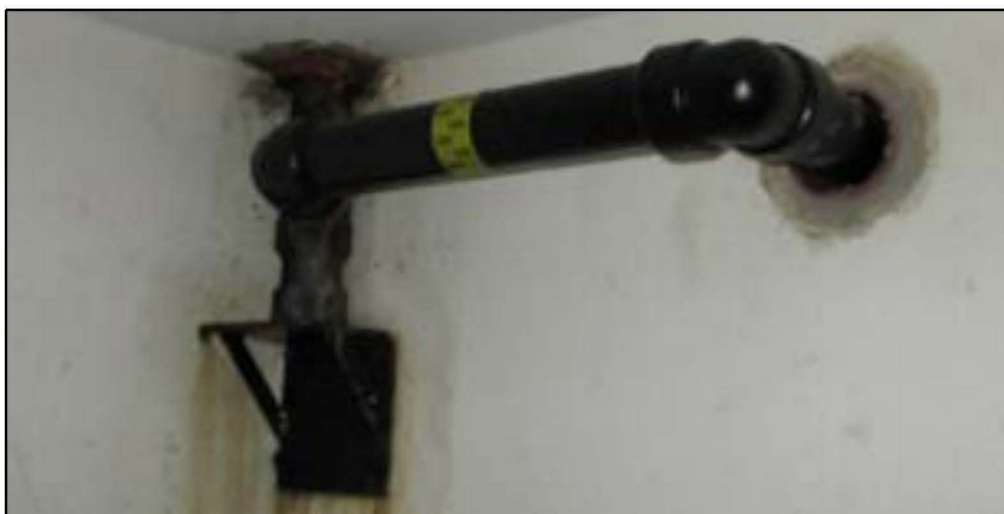
Figure K.19: Residential gas supply system 2 gas piping in Community Meeting Room (Level 2)
