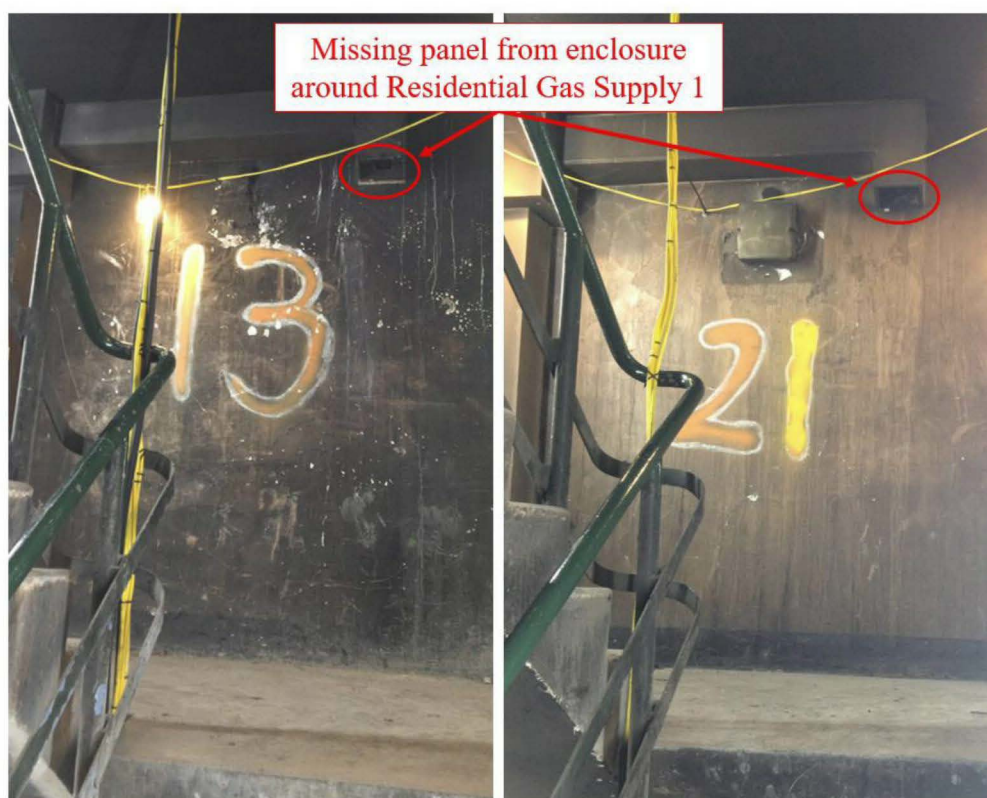
Figure K.22: Missing panel from enclosure around Gas Supply 1 in the protected stairway on Levels 13 and 21.
