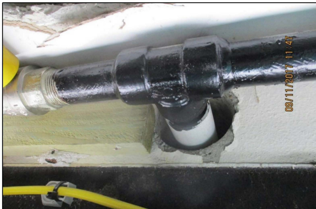
Figure K.23: Gas pipe penetration through stair compartment wall to Level 5 lift lobby
