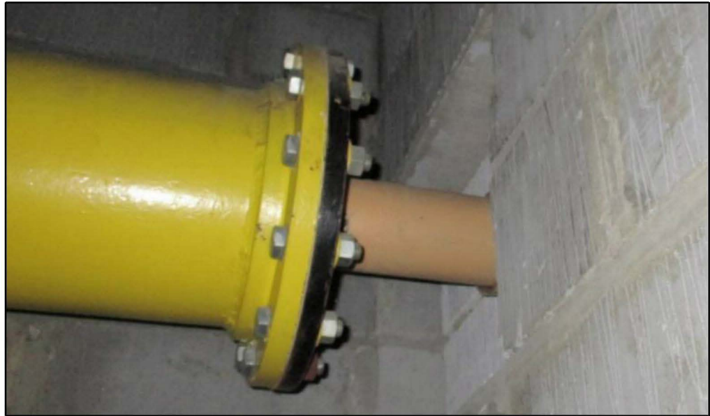
Figure K.10: Take-off for the new boiler gas supply
