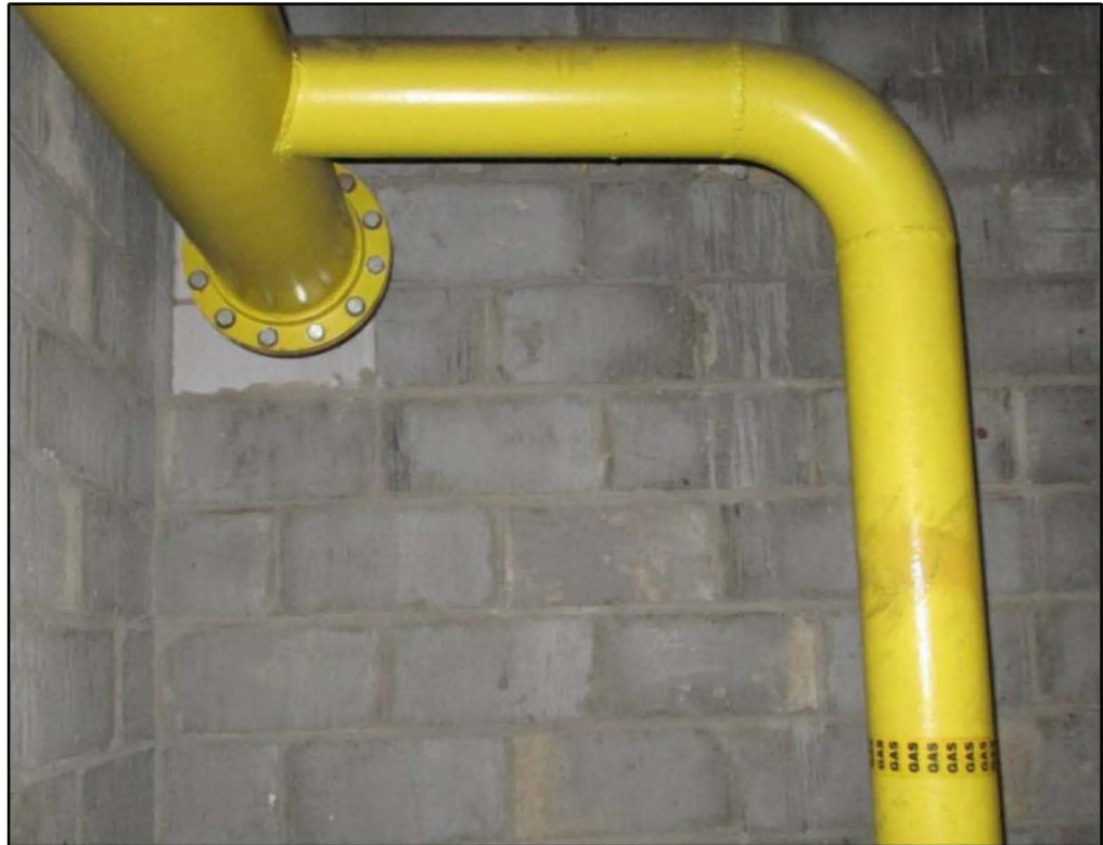
Figure K.8: Distribution header and a take-off in gas intake room 2
