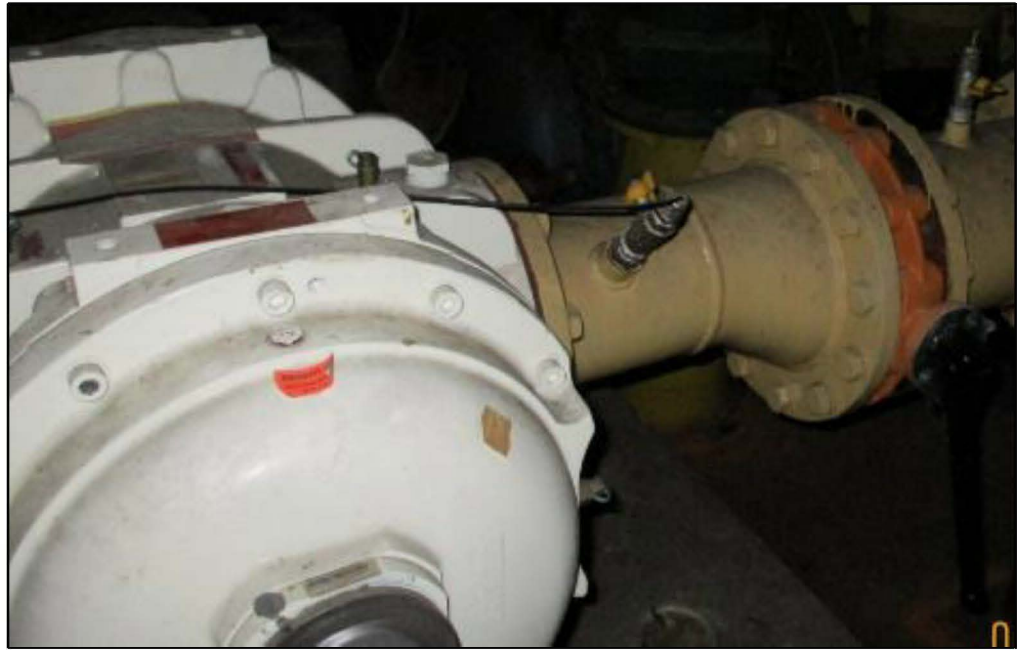
Figure K.6: Gas meter and manual isolation valve in gas intake room 1
