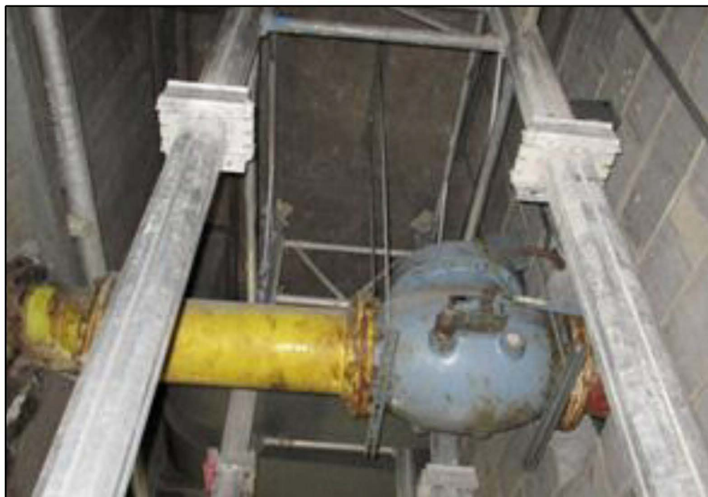
Figure K.2: Incoming pipe for Landlord Gas Supply System (approx. 4 – 5m above basement floor)
