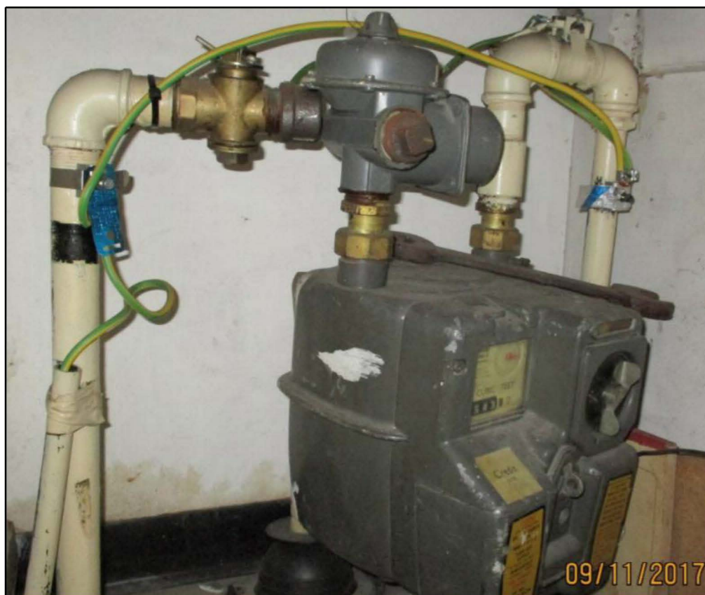
Figure K.17: Typical flat gas meter installation with emergency control valve upstream of meter
