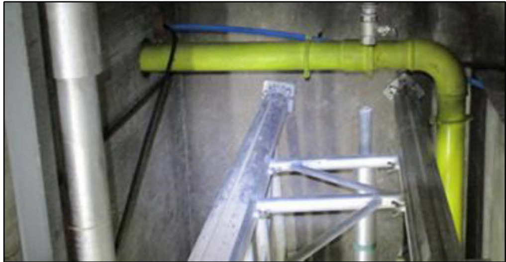
Figure K.13: Incoming pipe for residential gas supply system 1 entering basement on East elevation of building
