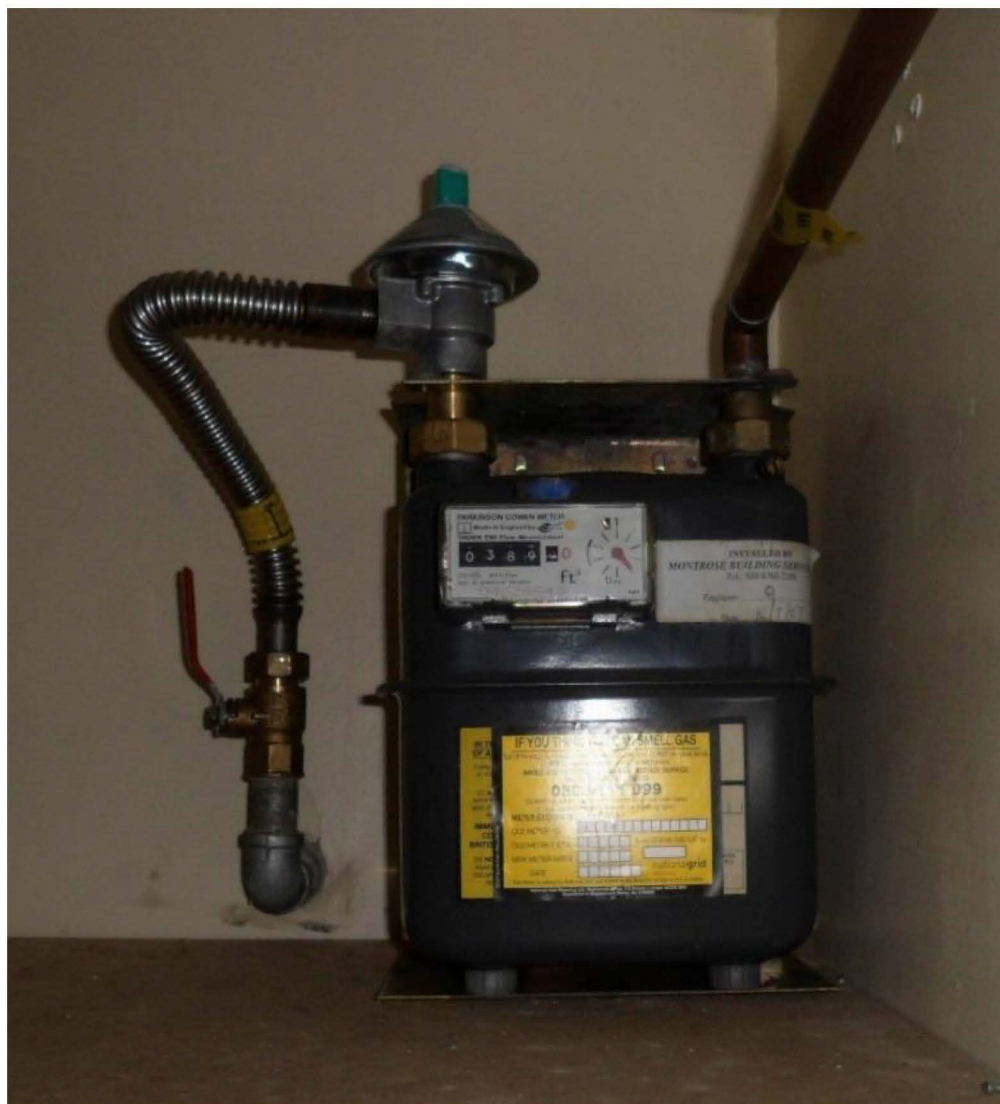
Figure K.28: Typical gas meter installation for Flat '2'
