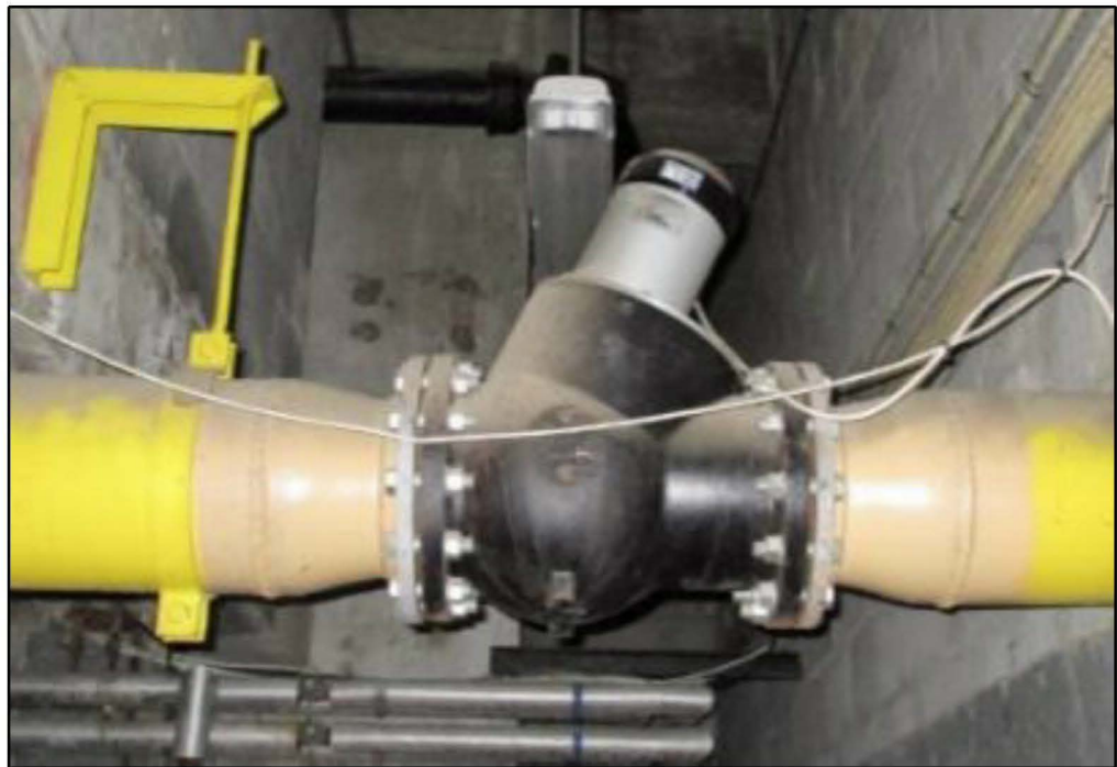
Figure K.7: Solenoid valve
