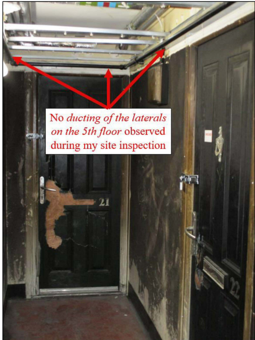
Figure K.26: Lateral gas piping distributed through Level 5 Lobby
