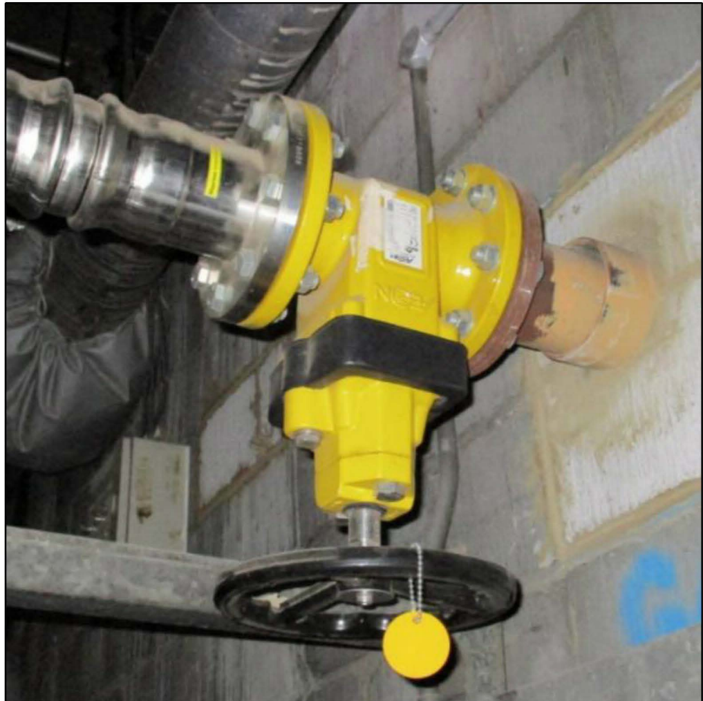
Figure K.11: Manual isolation valve for the gas pipework serving the new boilers, as it exits gas intake room 2
