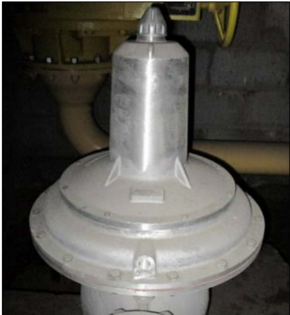
Figure K.5: Pressure reducing valve in gas intake room 1
