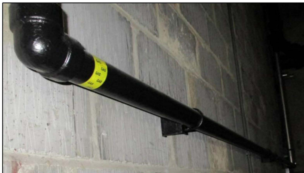
Figure K.29: Residential gas supply 1 pipe markings in basement
