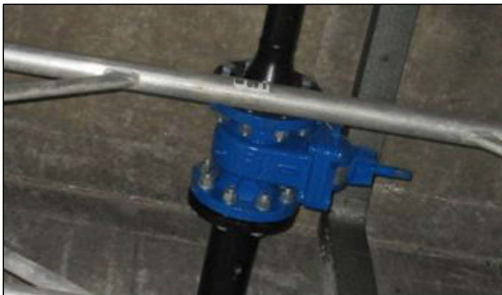
Figure K.18: Incoming pipe for residential gas supply 2 entering basement on east elevation of building with inaccessible isolation valve
