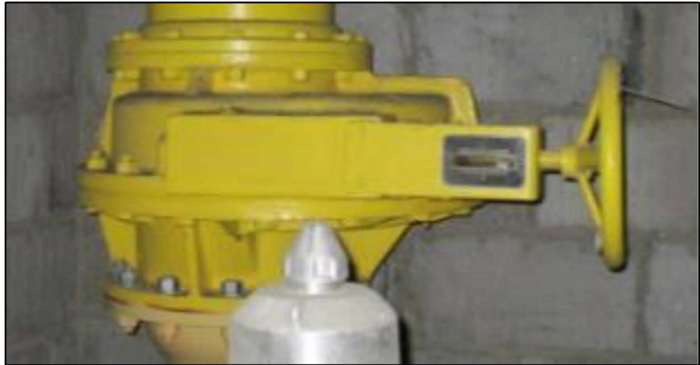
Figure K.4: Isolation control valve at low level in gas intake room 1
