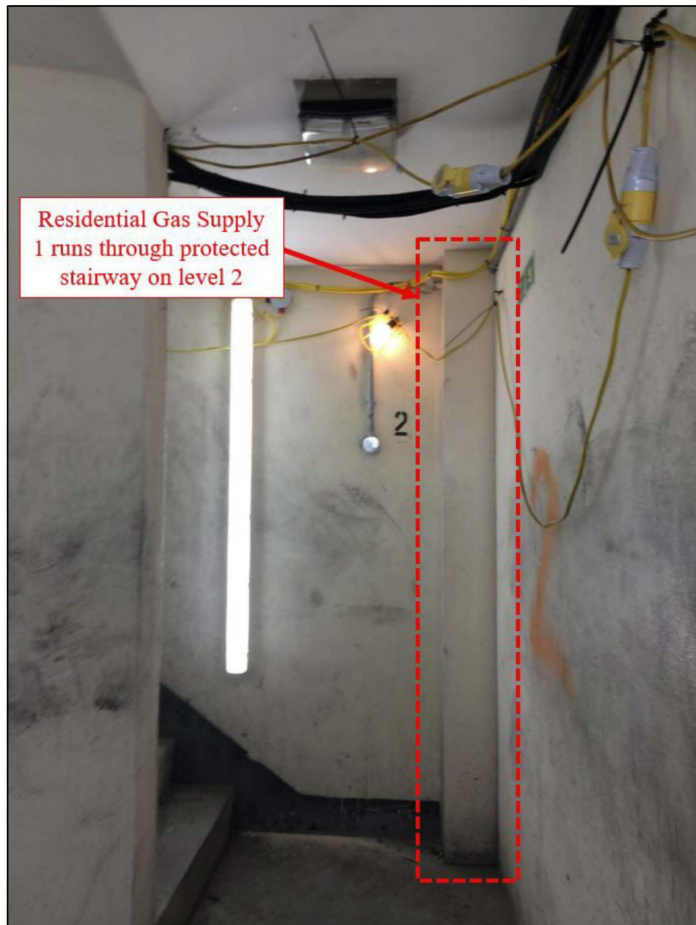
Figure K.21: Residential gas supply 1 runs through protected stairway on Level 2
