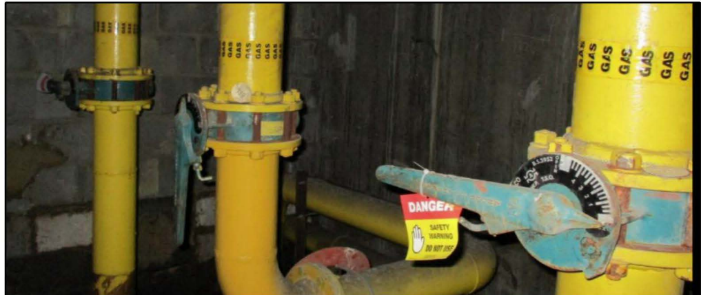
Figure K.9: Three (3) original take-offs from the gas main header in gas intake room 2 to the existing boilers
