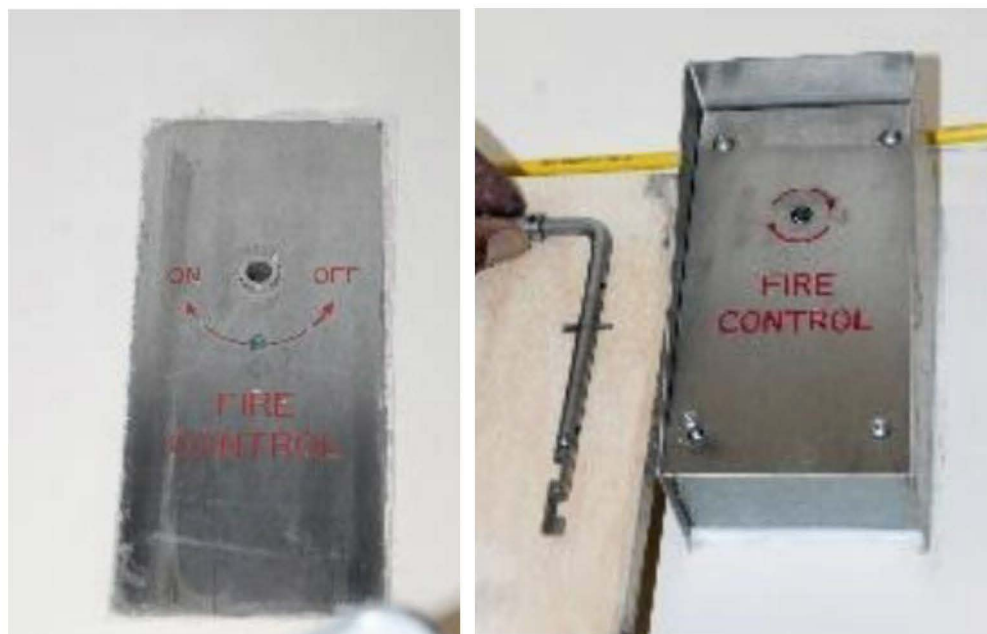
Figure L.11: Photographs from WSP site investigation report (MET00019973) showing both ground level (left) and level 2 (right) switches were embossed with 'FIRE CONTROL' in red lettering
