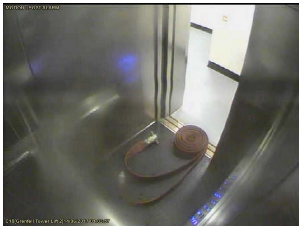
Figure L.24: CCTV image of hose reel in lift doors. Timestamp 01:03 (INQ00000150)
