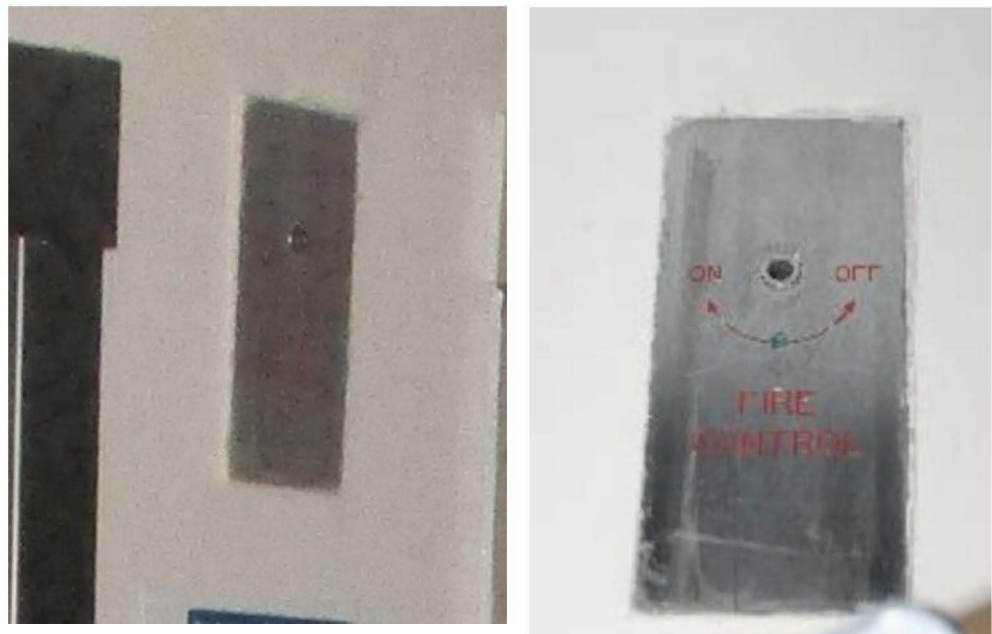
Figure L.17: Fire control switch as noted on ground level lobby (left: my observations, right: WSP site inspection report)
