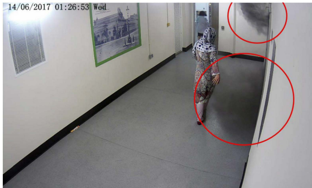
Figure L.27: Residents escaping using the lift at 01:26 (Ground) (MET00012593) Smoke leaking from lift doors circled in red
