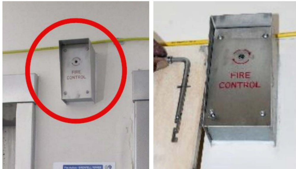
Figure L.16: Fire control switch as noted on Level 2 lobby (left: my observations, right: WSP site inspection report)
