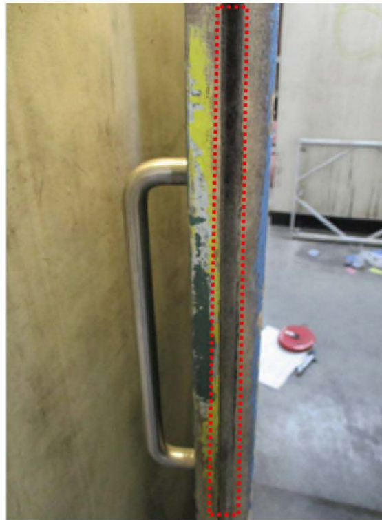
Figure M.14 Level 6 stair door (pile brush seals (potentially for cold smoke leakage) present on door leaf edge highlighted with red dashed line. Unclear whether there are intumescent materials behind the brush seal to restrict hot gas leakage. Edge of door un-planed; original paints visible (yellow and green)
