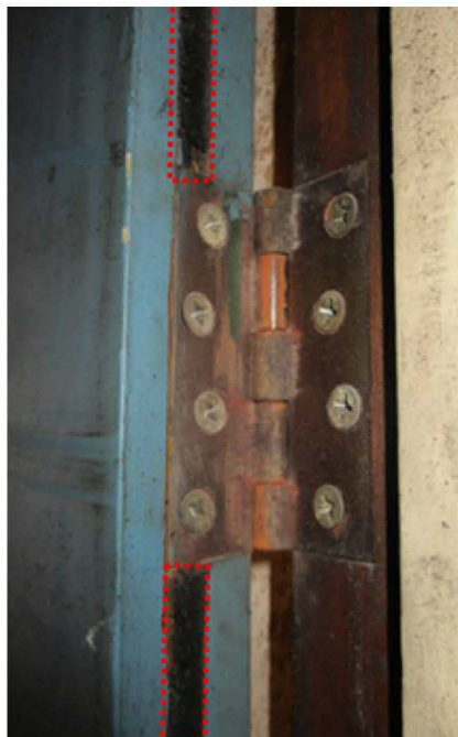
Figure M.15 Level 6 stair door (pile brush seals (potentially for cold smoke leakage) present on door leaf edge highlighted with red dashed line. Unclear whether there are intumescent materials behind the brush seal to restrict hot gas leakage. Blue and the original green paint on the door hinge
