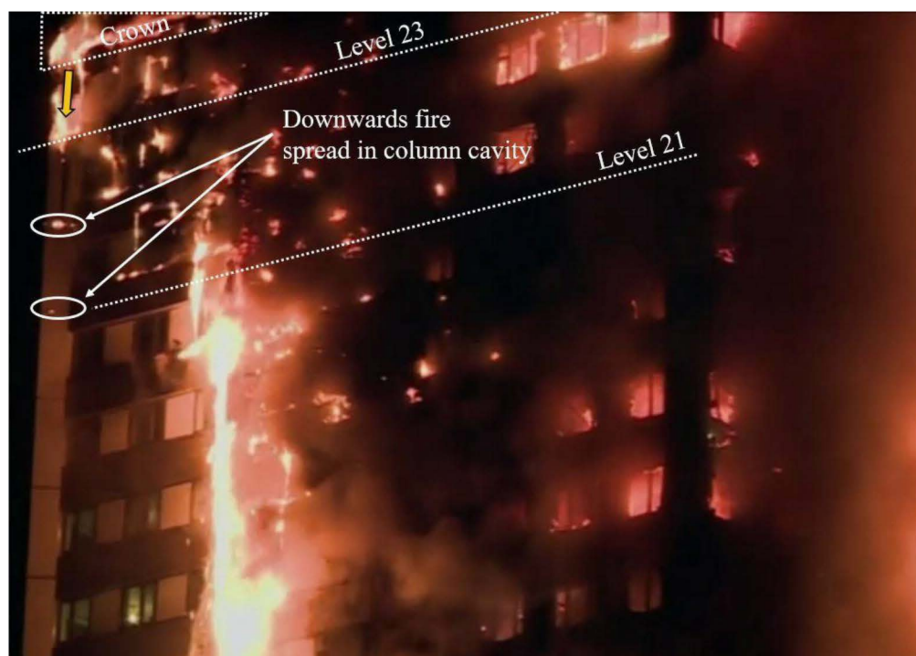
Figure 10.65: External fire spread along the exterior of the Southeast column (D5) and within the column cavity 16
