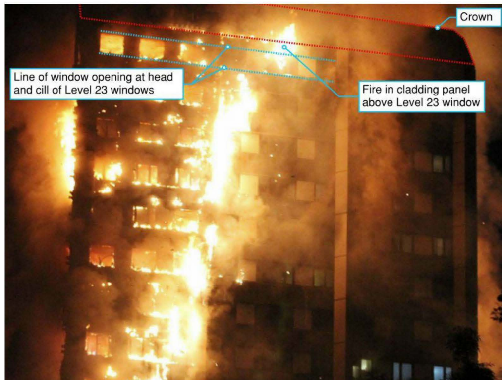
Figure 10.74: Fire in cladding panel above 19
