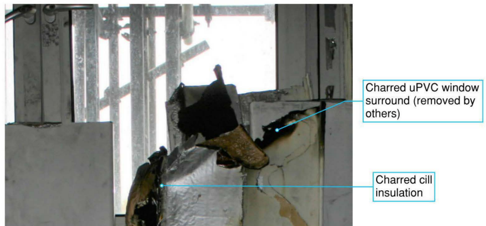
Figure 10.54: Evidence of burned uPVC and cill insulation in Flat 15
