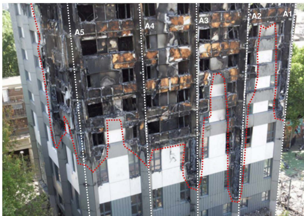
Figure 10.69: Post-fire damage on North elevation of Grenfell Tower (METS00020592)
