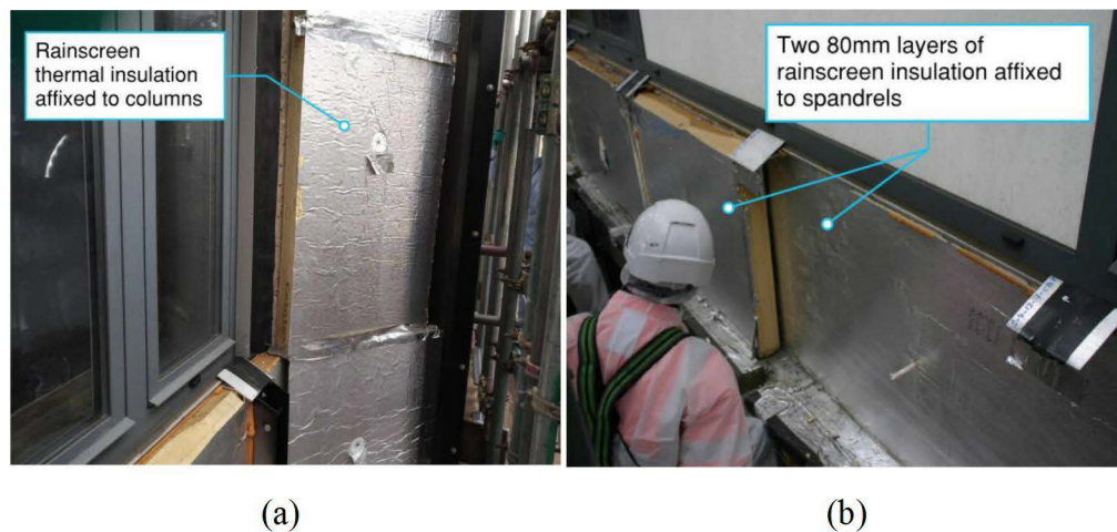
Figure 11.10 Rainscreen thermal insulation affixed to (a) Columns and (b) spandrel panels
