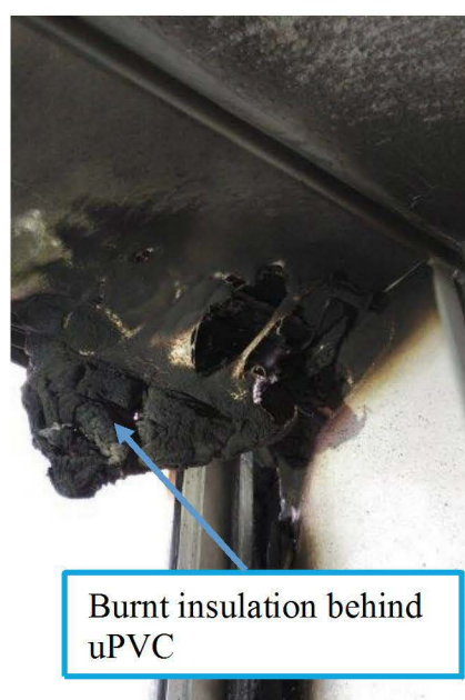
Figure 11.37 Internal window head-burnt insulation behind uPVC surround
