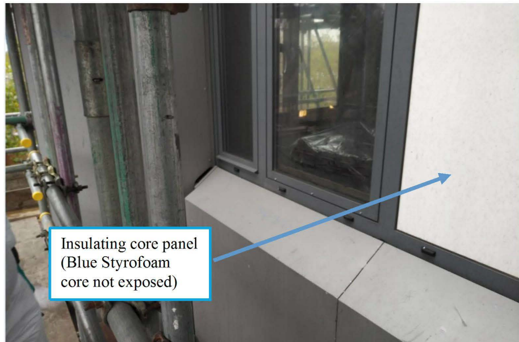
Figure 11.9 Insulating core panel between windows
