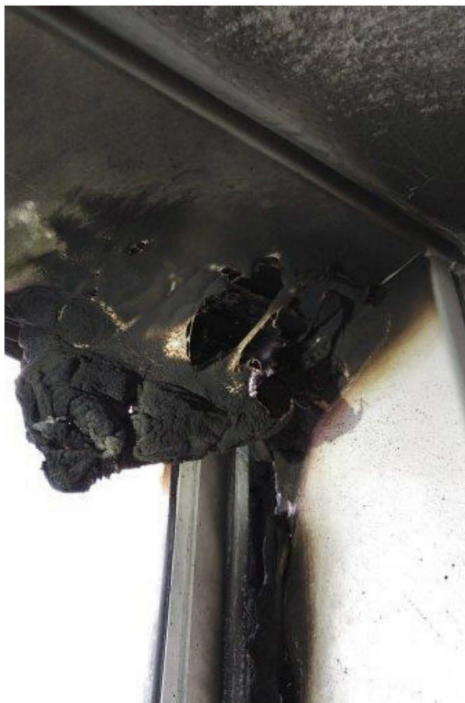
Figure 11.27 Charred foam insulation noted behind deformed UPVC window surround
