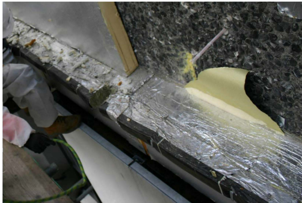
(b) Horizontal cavity barrier affixed to spandrel – upside down position indicated by absence of green logo on top surface
