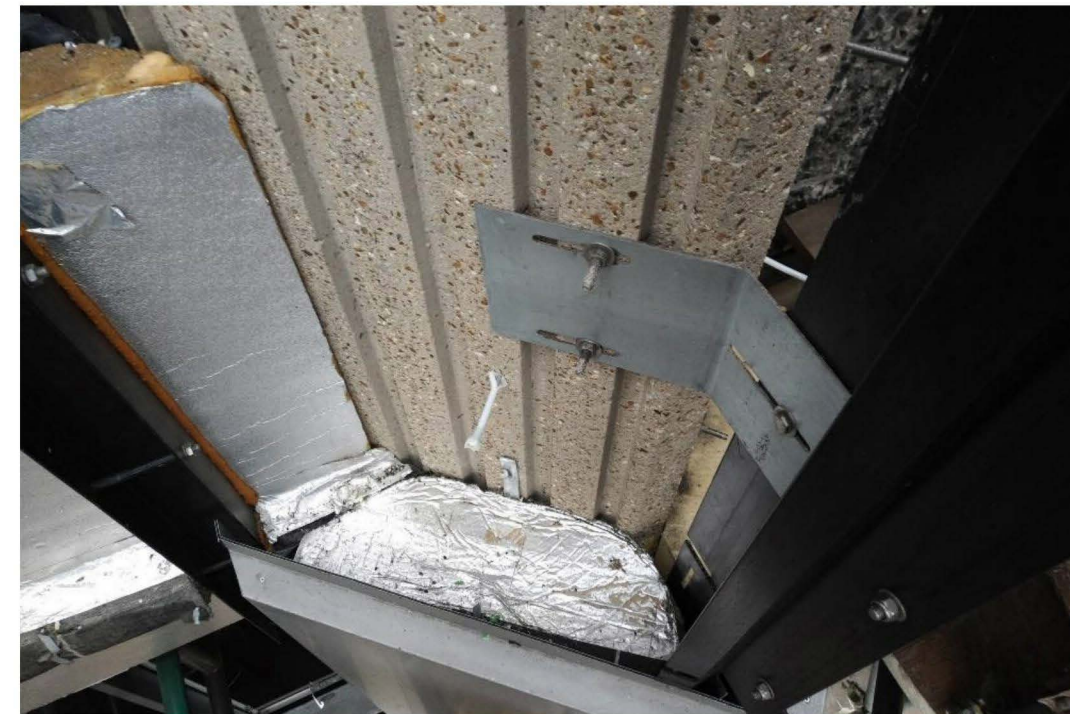
(c) visible gap at the junction of the horizontal cavity barriers fitted to the spandrel panels and the columns
