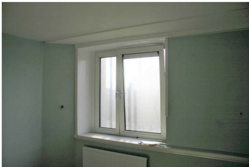
Figure 11.26 Undamaged UPVC surround of window
