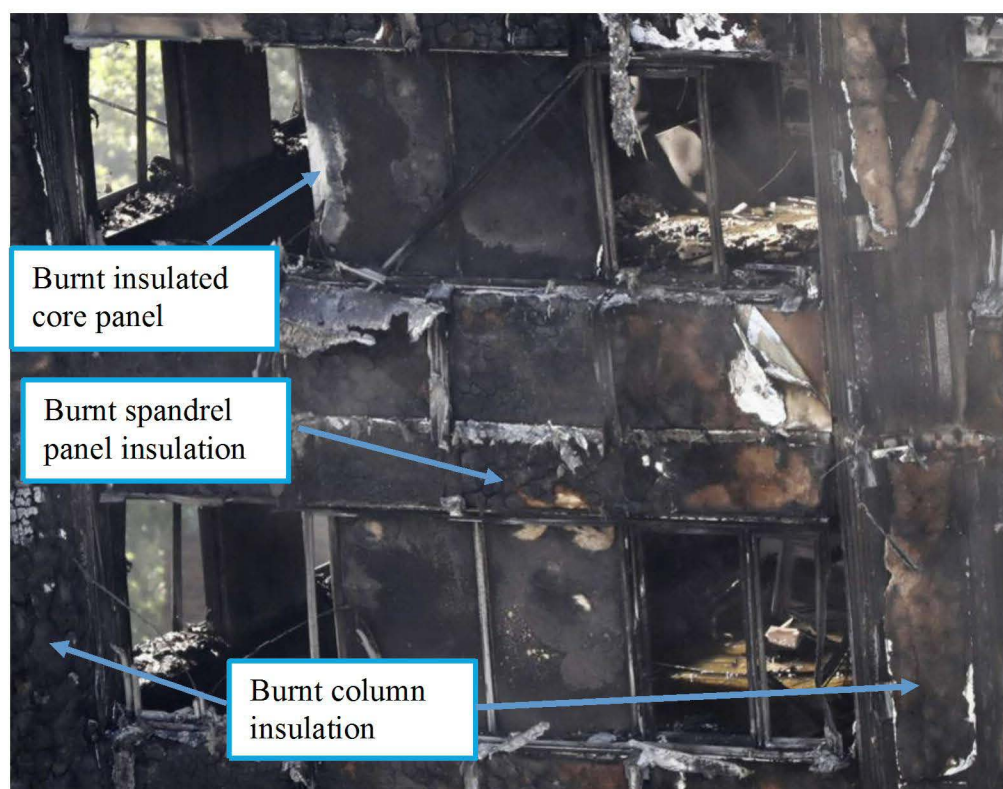
Figure 11.36 External view of burned surfaces
