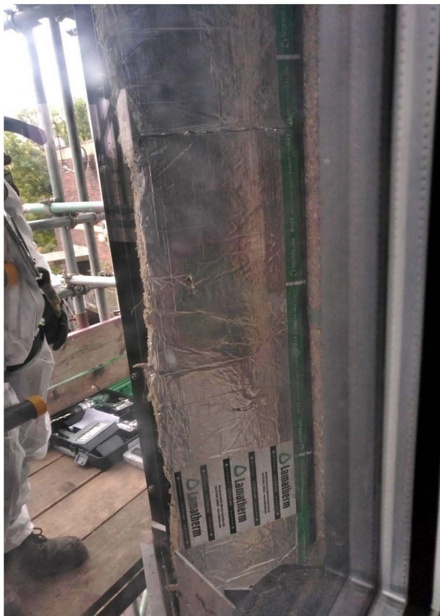
Figure 11.30 Siderise RH horizontal application cavity barrier installed vertically, with intumescent strip facing column D1 outside flat 13 (indicated by green Siderise RH logo)
