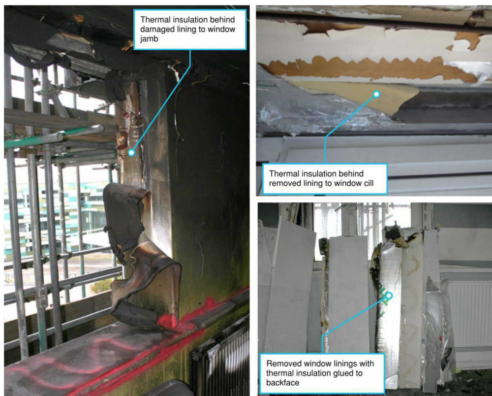
Figure 11.11 Thermal insulation behind the window opening linings
