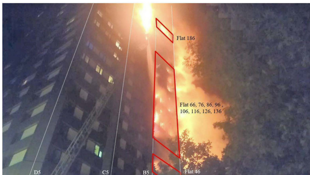
Figure 12.10: Internal fires, photograph of East elevation of building; exact time between 01:43 and 01:57 not known (extract from Video 2 accompanying Luke Bisby's supplemental phase 1 Report)
