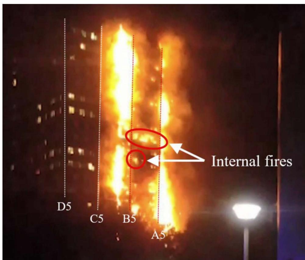
Figure 12.7: My first observation of internal fires at 01:44 on the East elevation of building envelope (extract from Bisby Video 2 accompanying Luke Bisby's supplemental phase 1 Report)
