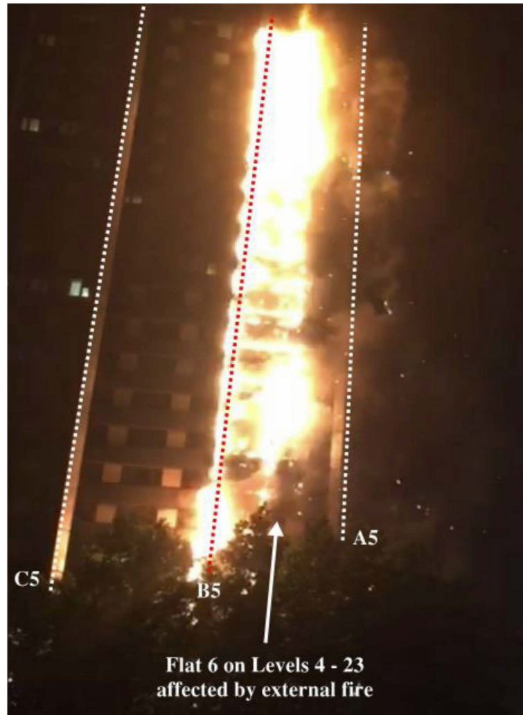
Figure 12.6: Flat 6 on Levels 4 - 23 affected by external fire at 01:26 (IWS00000046)
