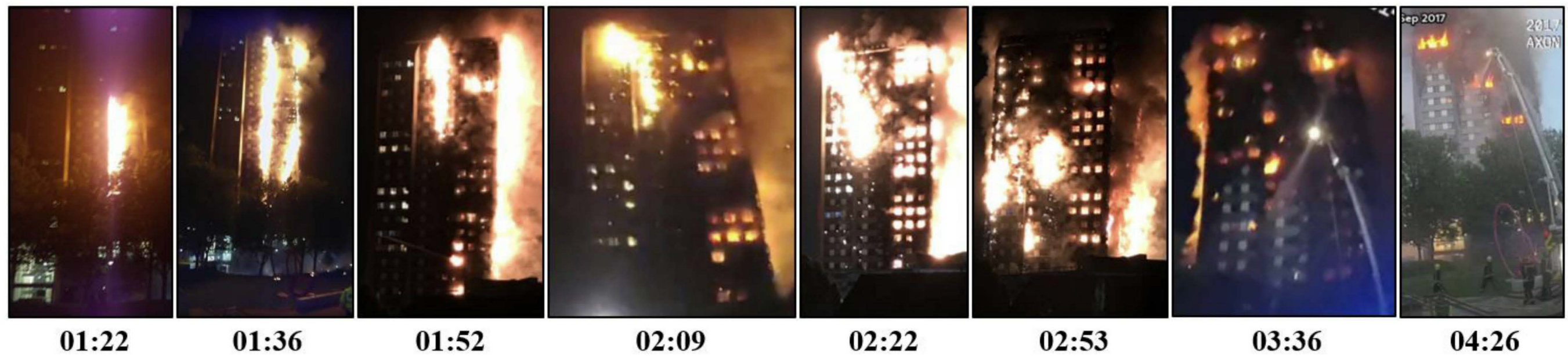
Figure 12.12.13: External flame front on East elevation of building envelope and increasing numbers of internal fires on East building elevation, between 01:22 and 04:26 (MET00012593) 4
