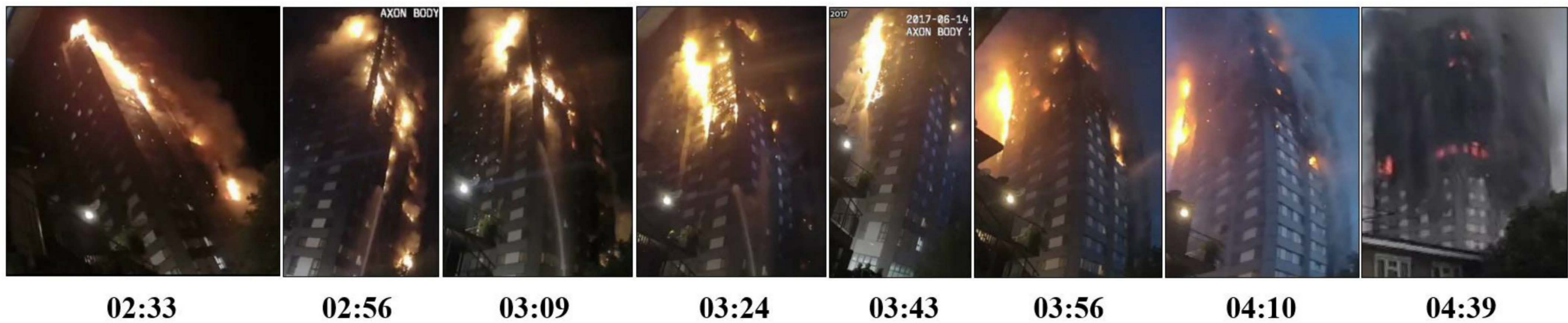
Figure 12.15: External flame front on South elevation (left) and East elevation (right) of building envelope and increasing numbers of internal fires on both building elevations, between 02:33 and 04:39 (MET00012593)
