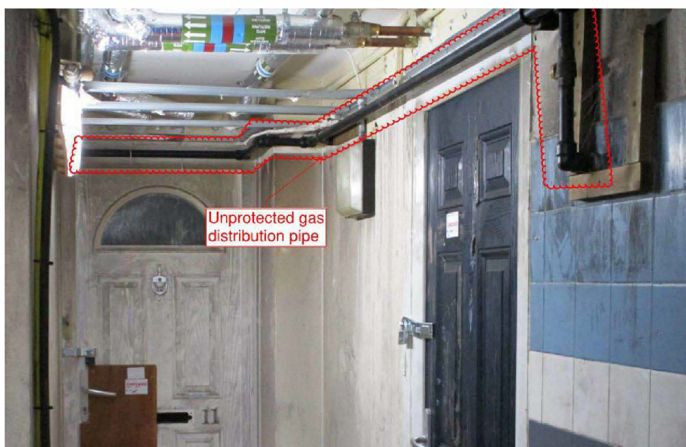
Figure 14.43: Unprotected gas distribution pipe in Level 4 lobby
