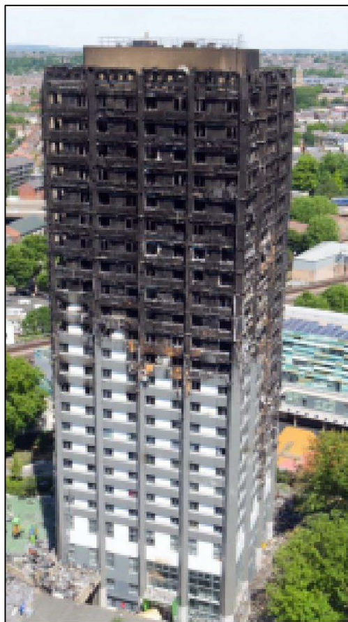
(a) South building envelope of Grenfell Tower, UAV image taken on 10/06/2017 (MET00012593)
