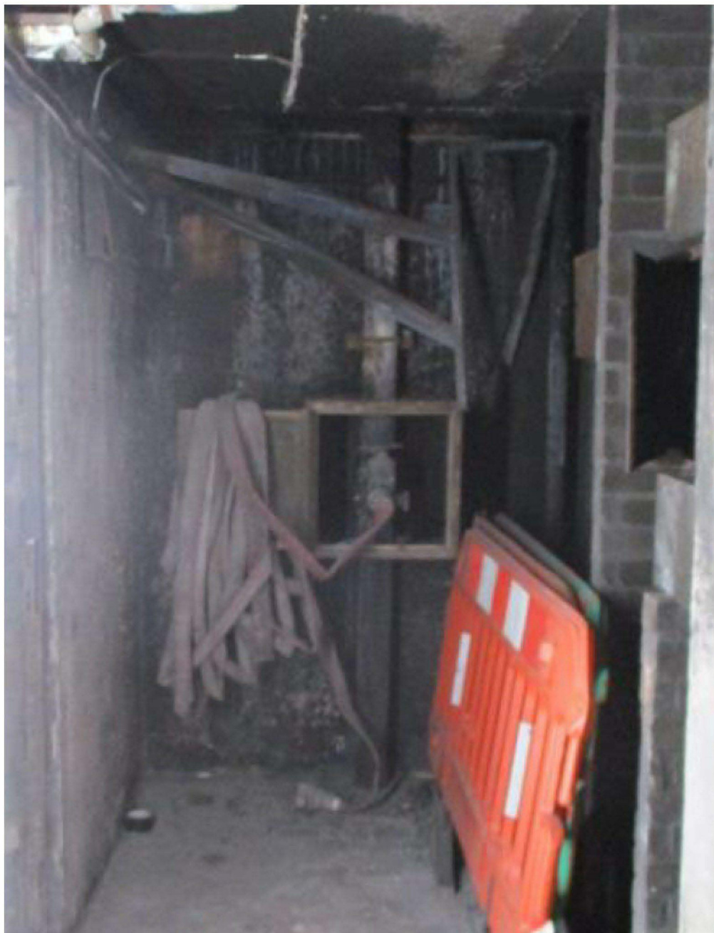
Figure 14.54: Damage around dry rising main outlet on Level 14, where a hose was attached
