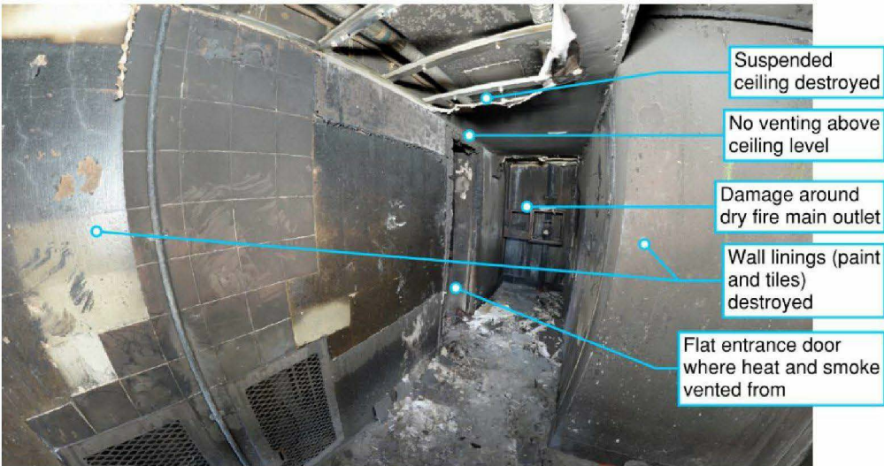
Figure 14.50: Example of how damage caused in lobby by smoke and heat venting from apartments through narrow corridor on Level 12 (South side) (METS00017072)
