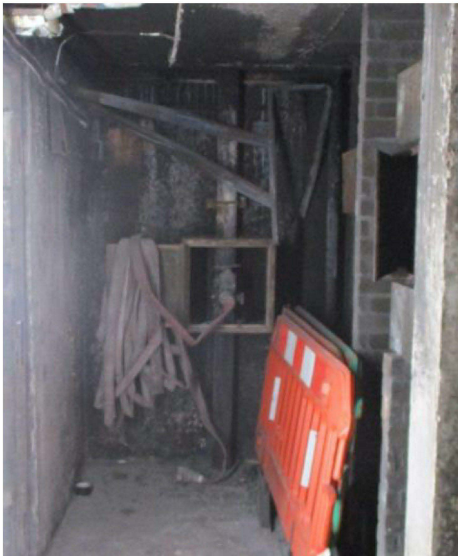
Figure 14.57 Hose connected to the fire main outlet on Level 14 of Grenfell Tower
