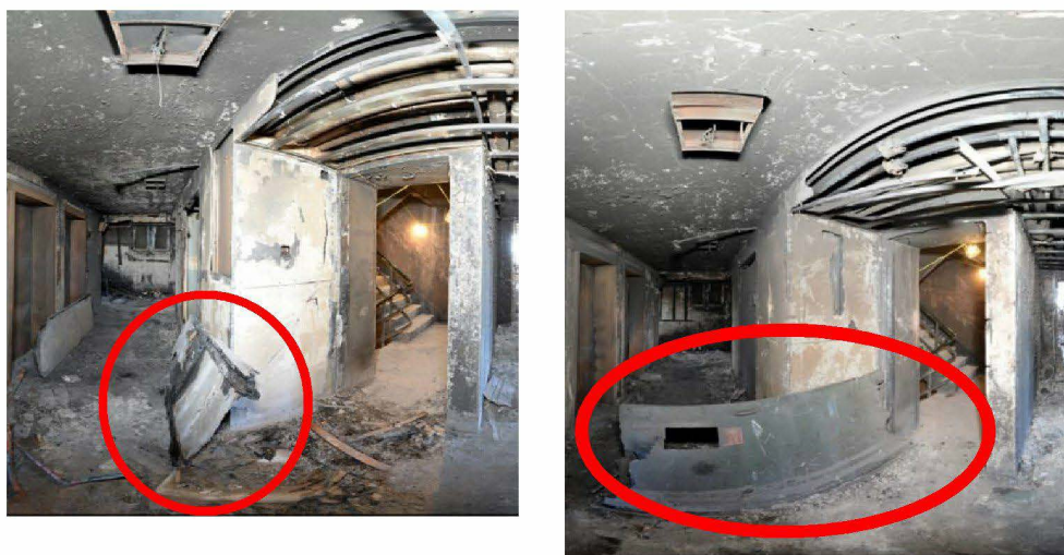
Figure 14.12 MPS photographs of the stair doors in the immediate aftermath of the fire (a) Level 16 and (b) Level 18 – remains of door circled in red in each
