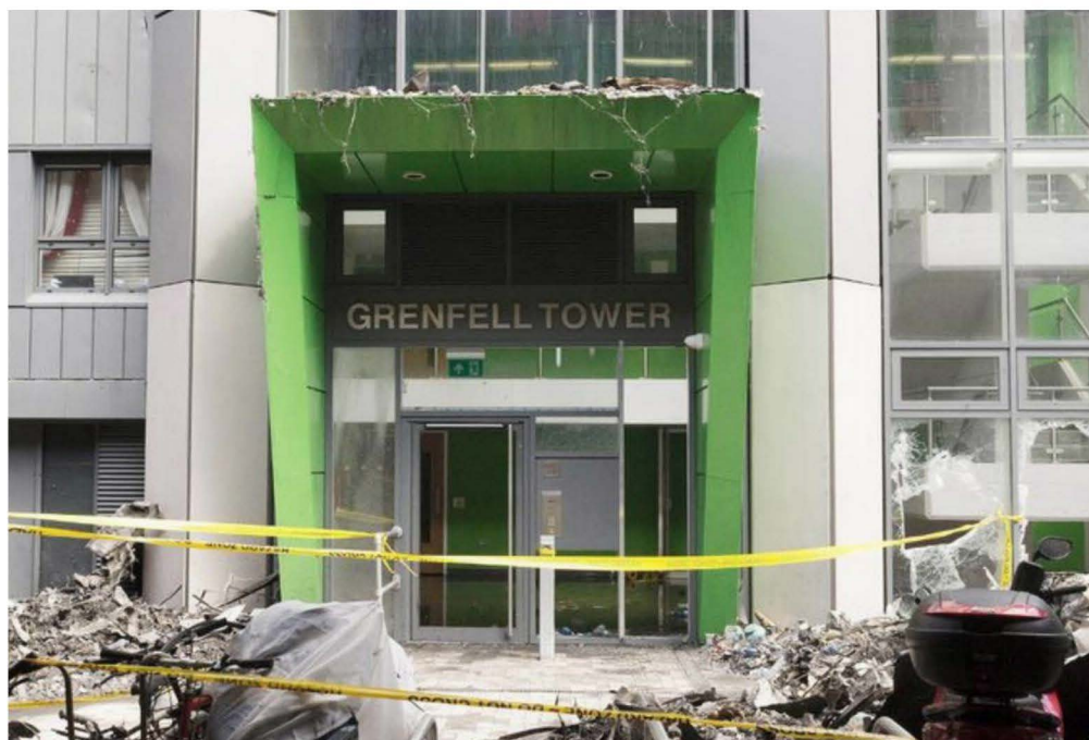
Figure 18.10: Grenfell Tower main entrance door, showing protective effect of canopy 1
