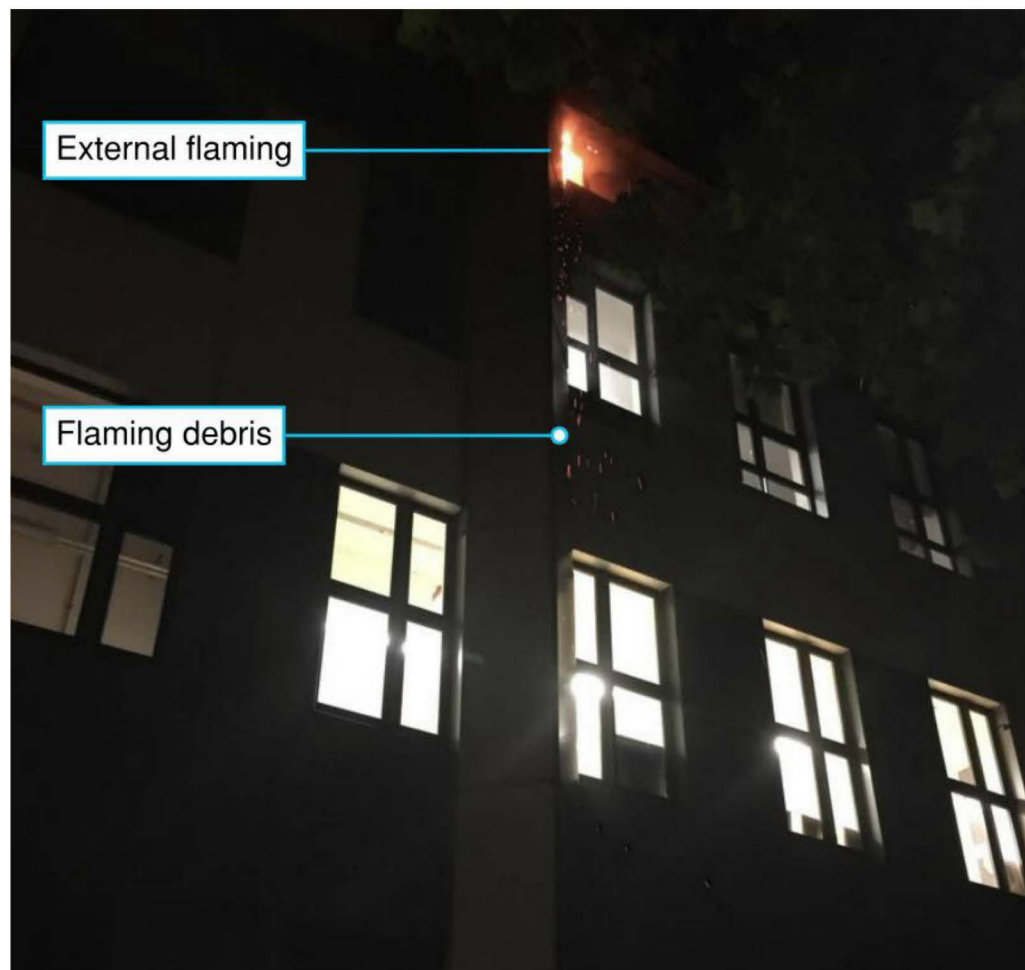
Figure 7.4: First external flaming observed at 01:08 (IWS00000051)
